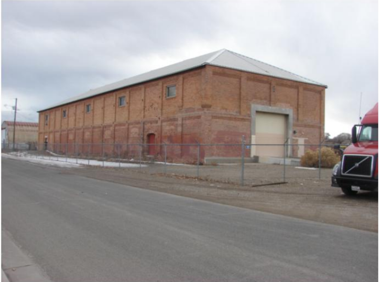
Photo 1 – Sugar Beet Factory building
