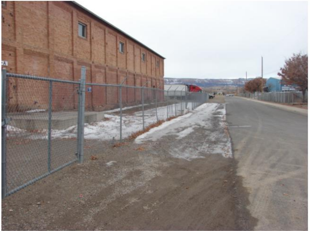
Photo 2 – Right-of-way next to Sugar Beet building
