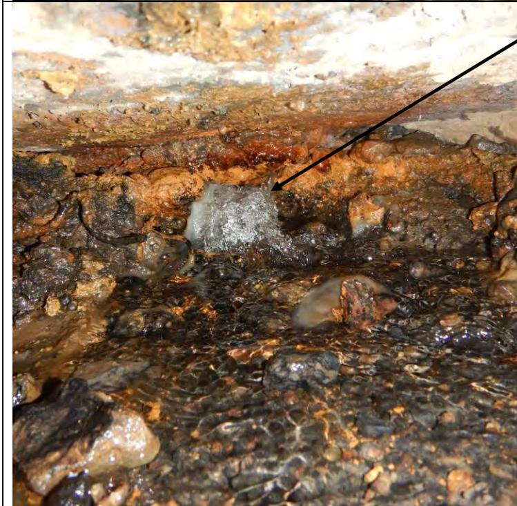
Water is bubbling from a broken pipe in the top of the outlet conduit encasement. The pipe is believed to extend to the upstream end of the conduit, passing along the conduit within the concrete encasement.
