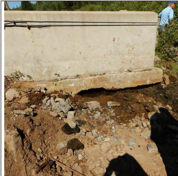
Water from the broken pipe emerges from under the slab and drains to the right side of the conduit, where it is collected in the excavation and routed around the right end of the headwall for measurement.
