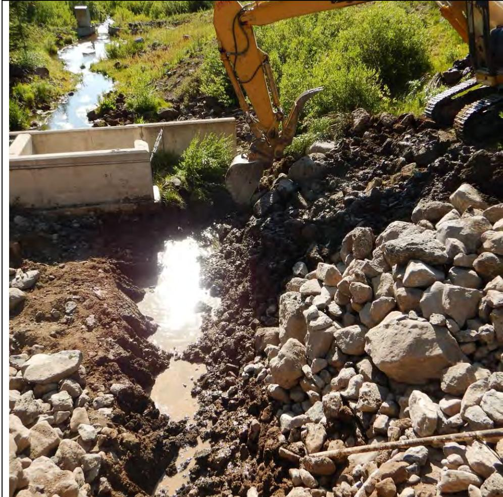
Backhoe cleaning channel for draining excavation along right side of conduit.
