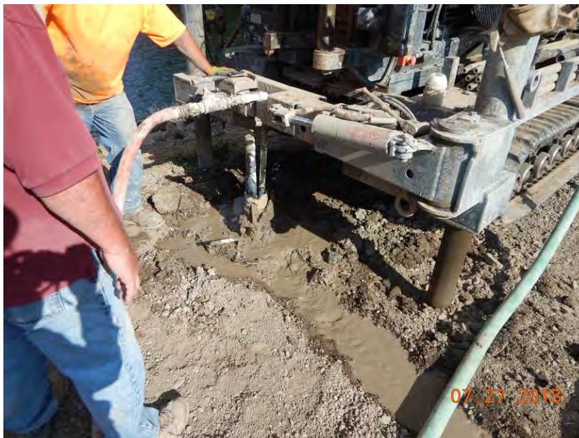
Figure 2. B-101 equipment set-up during grouting, looking southeast.
