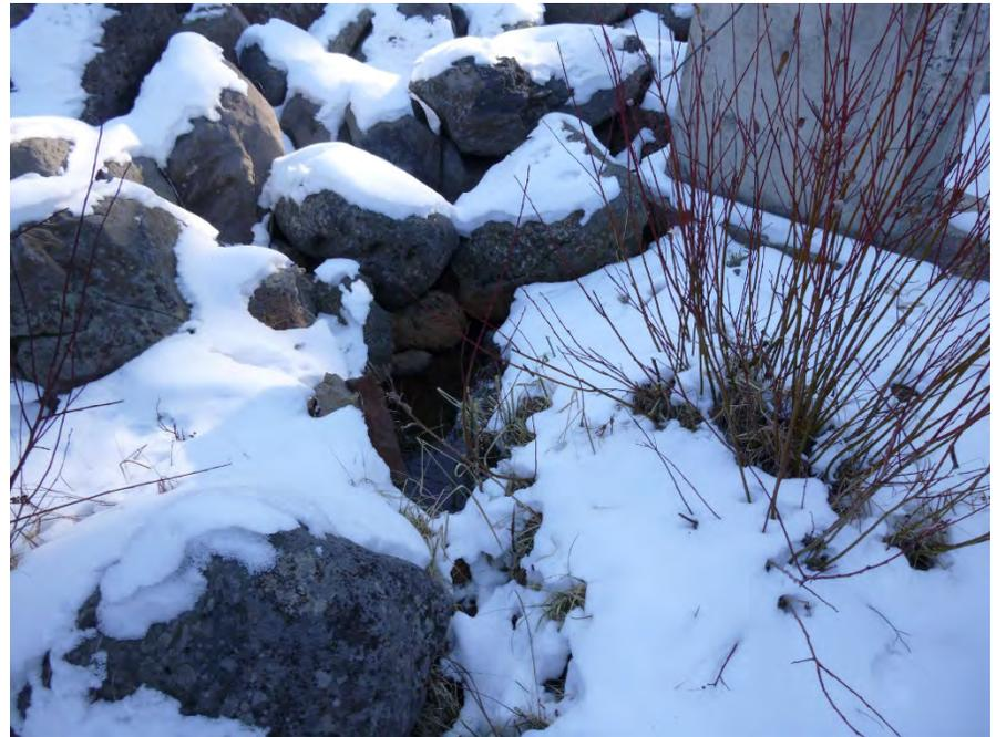
*Photo 11: Seepage behind right side of outlet headwall.*
