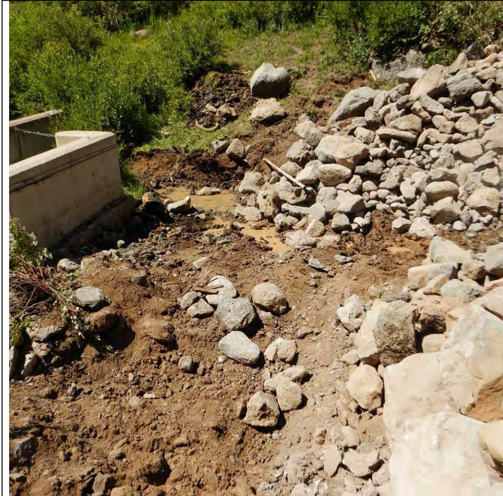
Pooled seepage water draining around right end of headwall.
