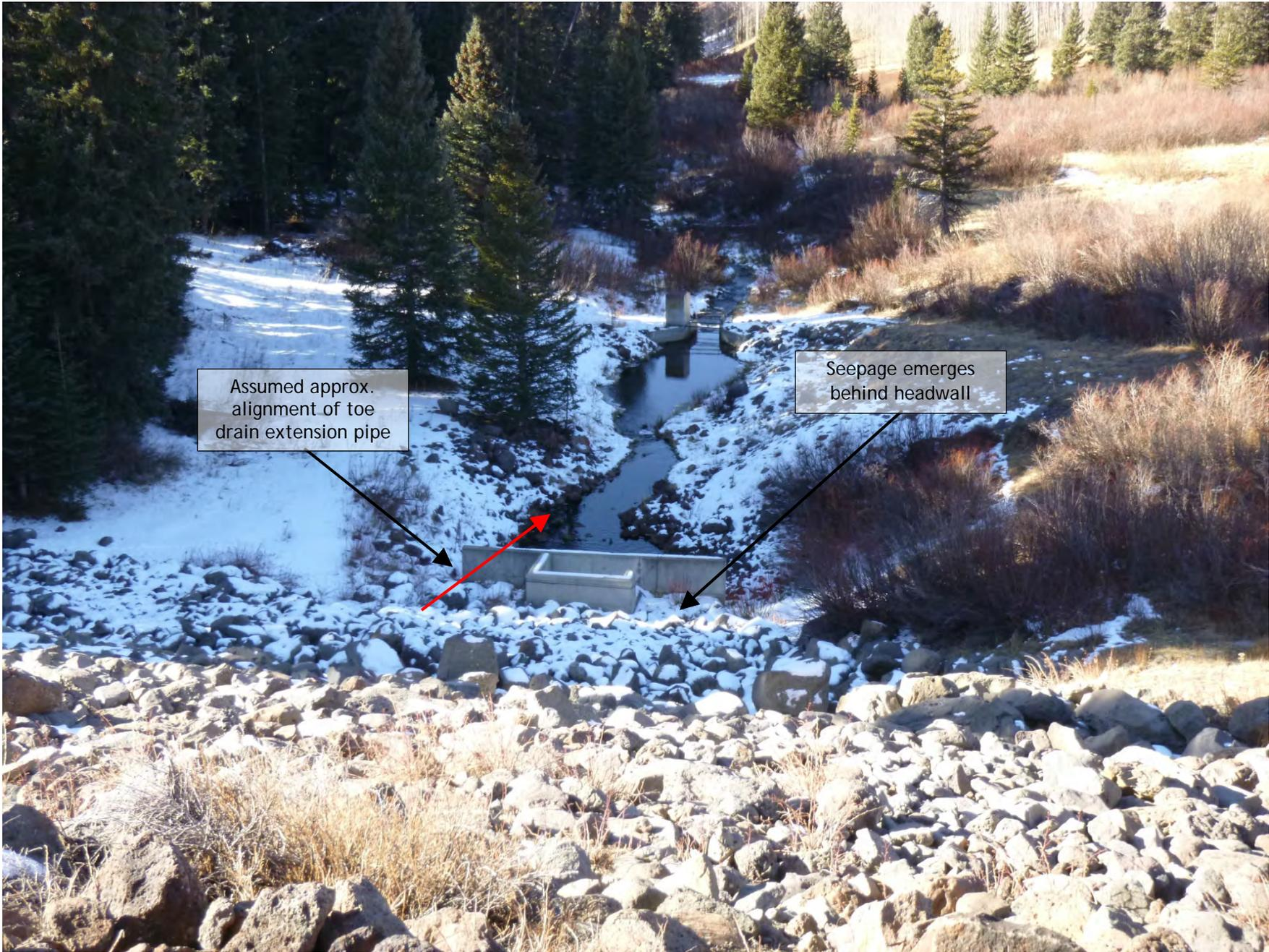
Photo 4: Downstream outlet headwall.
