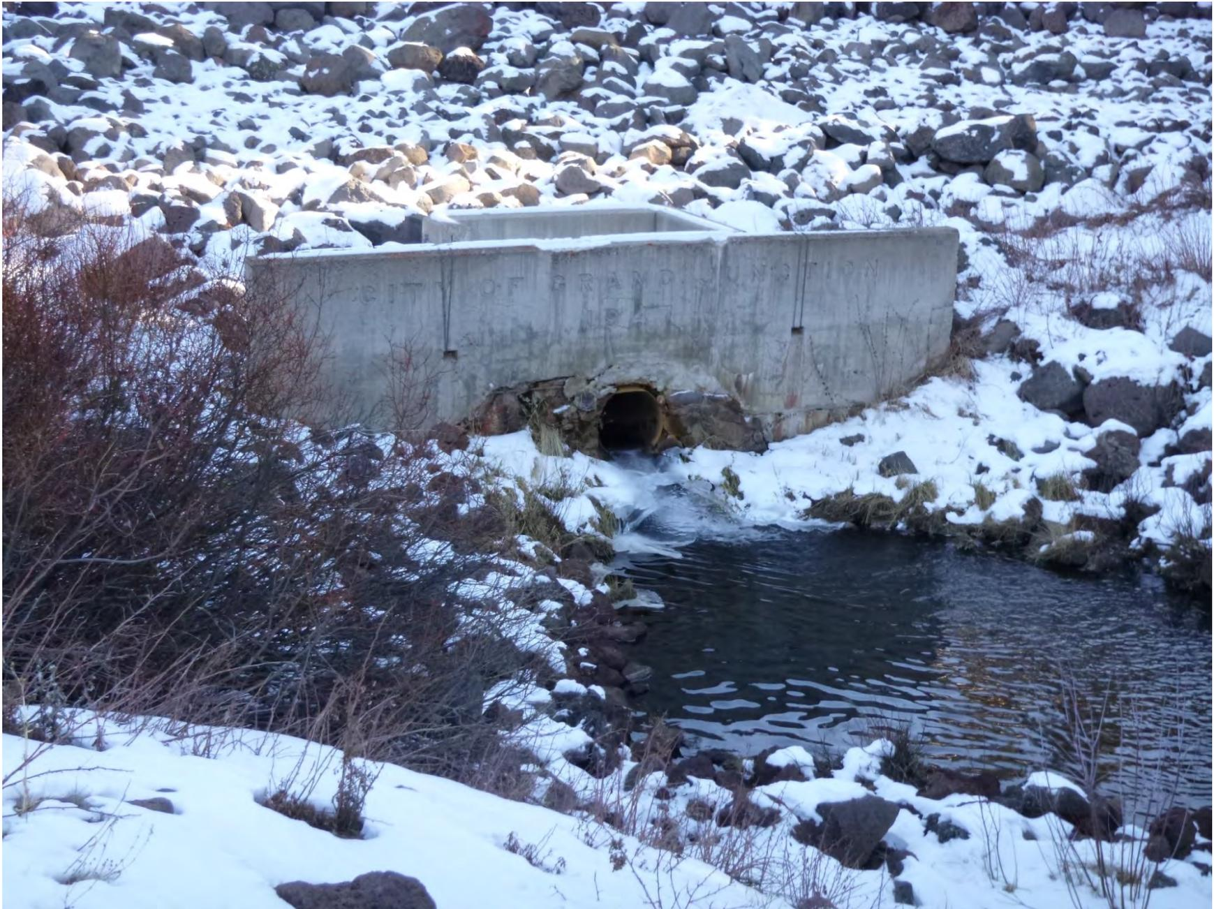
*Photo 5: Downstream outlet pipe headwall.*
