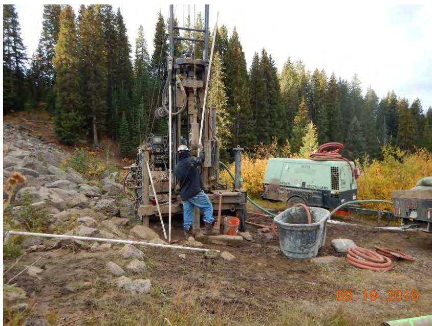
Figure 2. B-105A during monitoring well installation, looking south.
