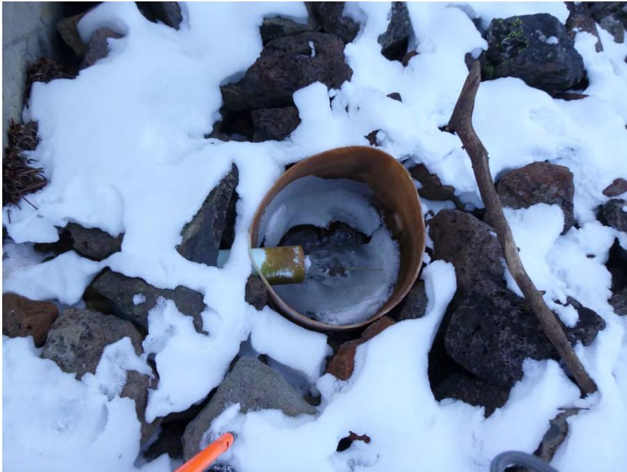
*Photo 7: Collection and monitoring pipe from right side of outlet headwall.*
