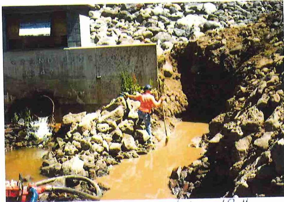
*Excavation of existing toe drain outfall*
