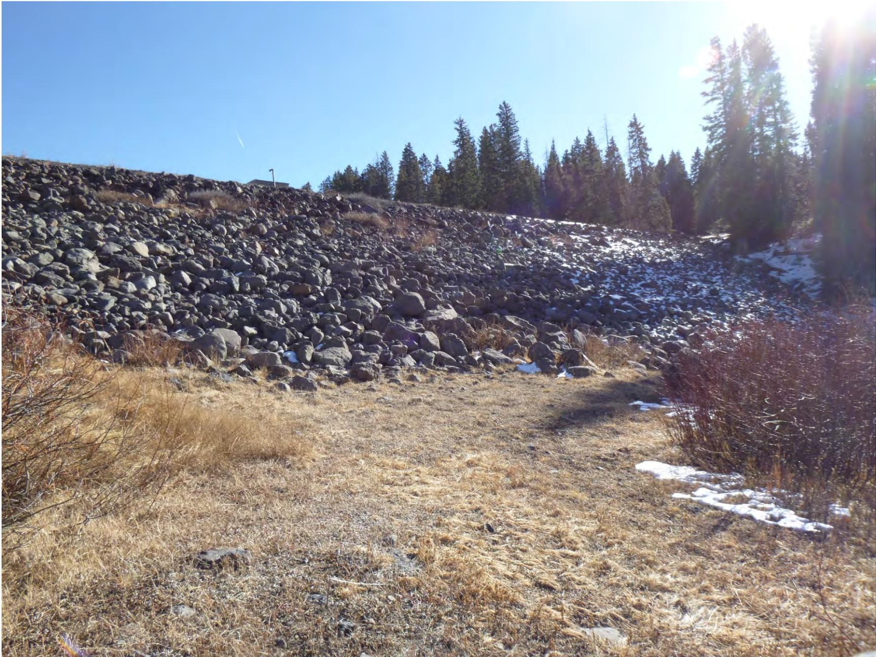
*Photo 3: Downstream slope; Zone 2 material per C-454*
