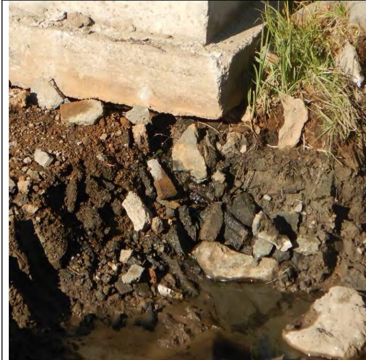
Seepage emerging from under the old control structure foundation slab is the only measurable water entering the excavation.
