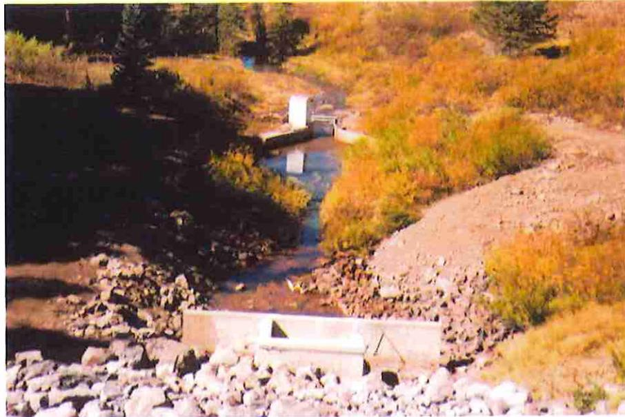
Old valve house removed & toe drain extension complete
