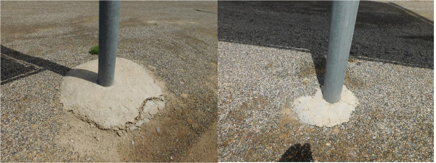
Footers for each pole need to be strengthened and repaired
