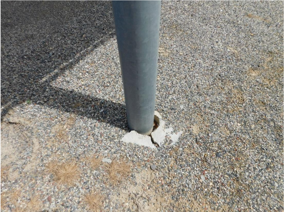
Footers for each pole need to be strengthened and repaired
