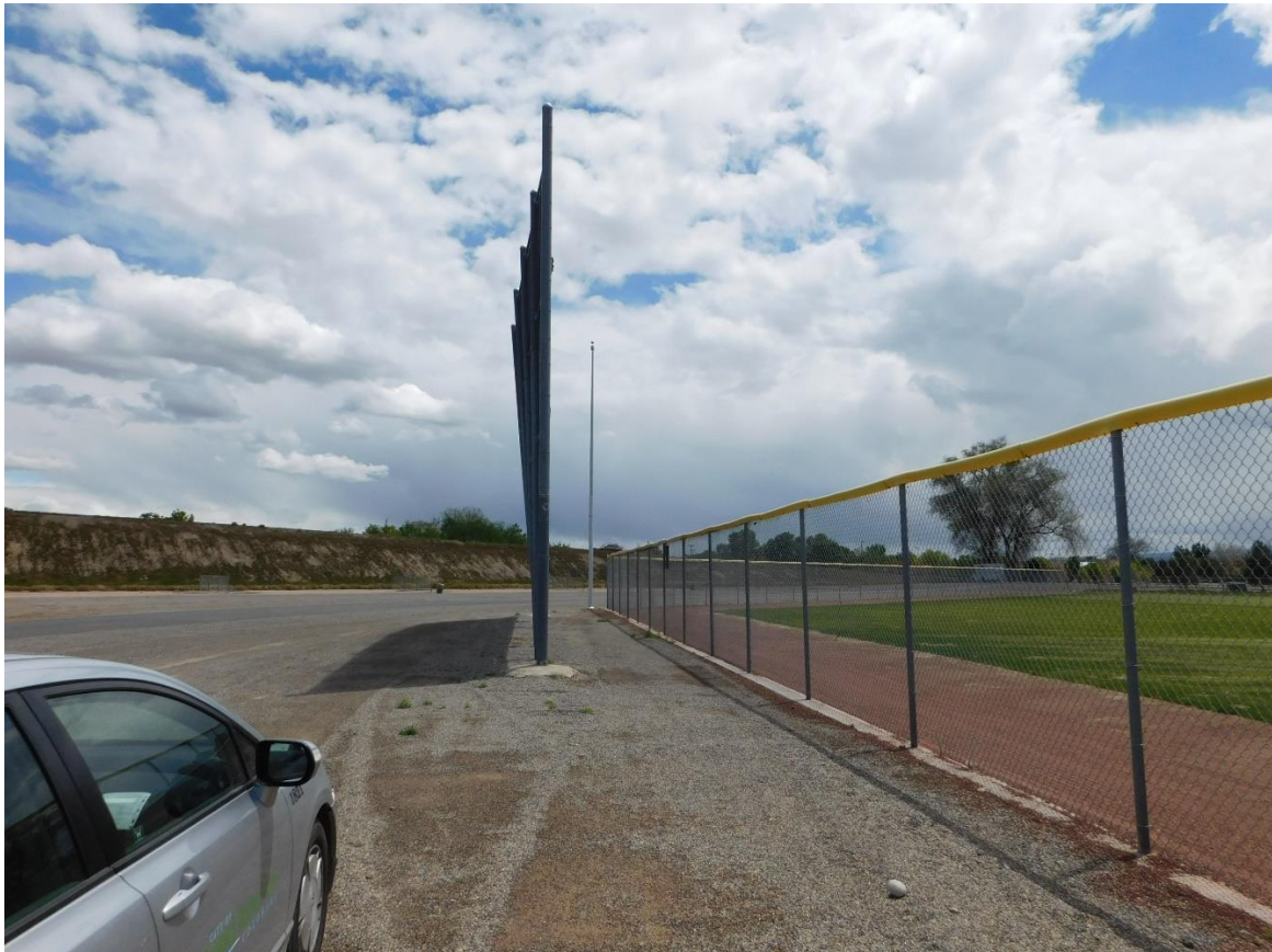
Looking from West to East, supports are bent and no longer plumb
