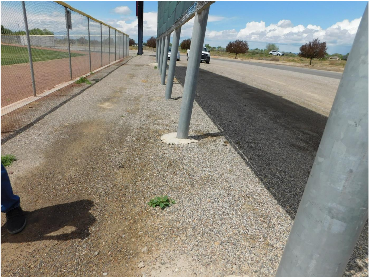
Approximately 10' between poles, and 6' from ground to bottom of screen
