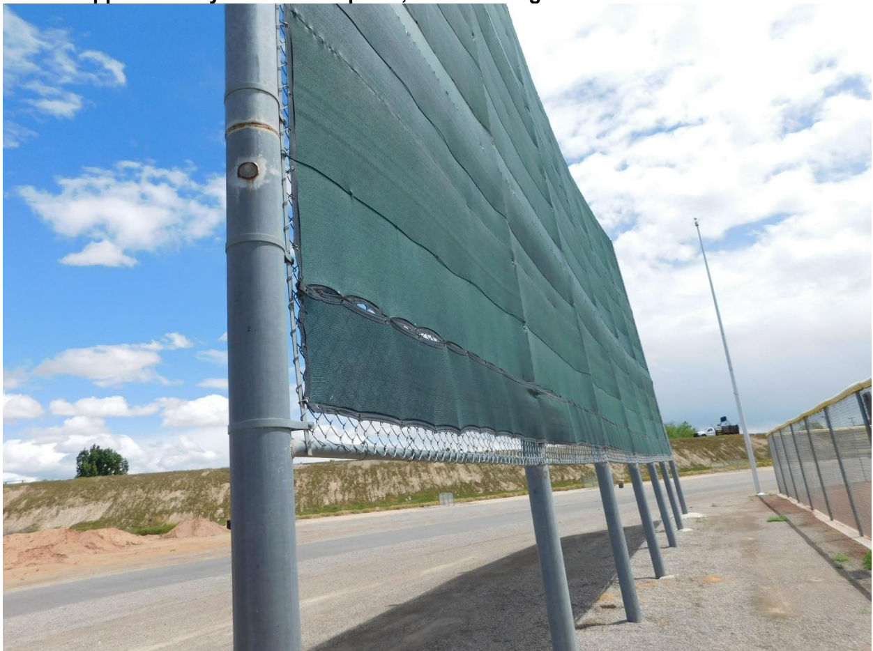
Approximately 10' between poles, and 6' from ground to bottom of screen
