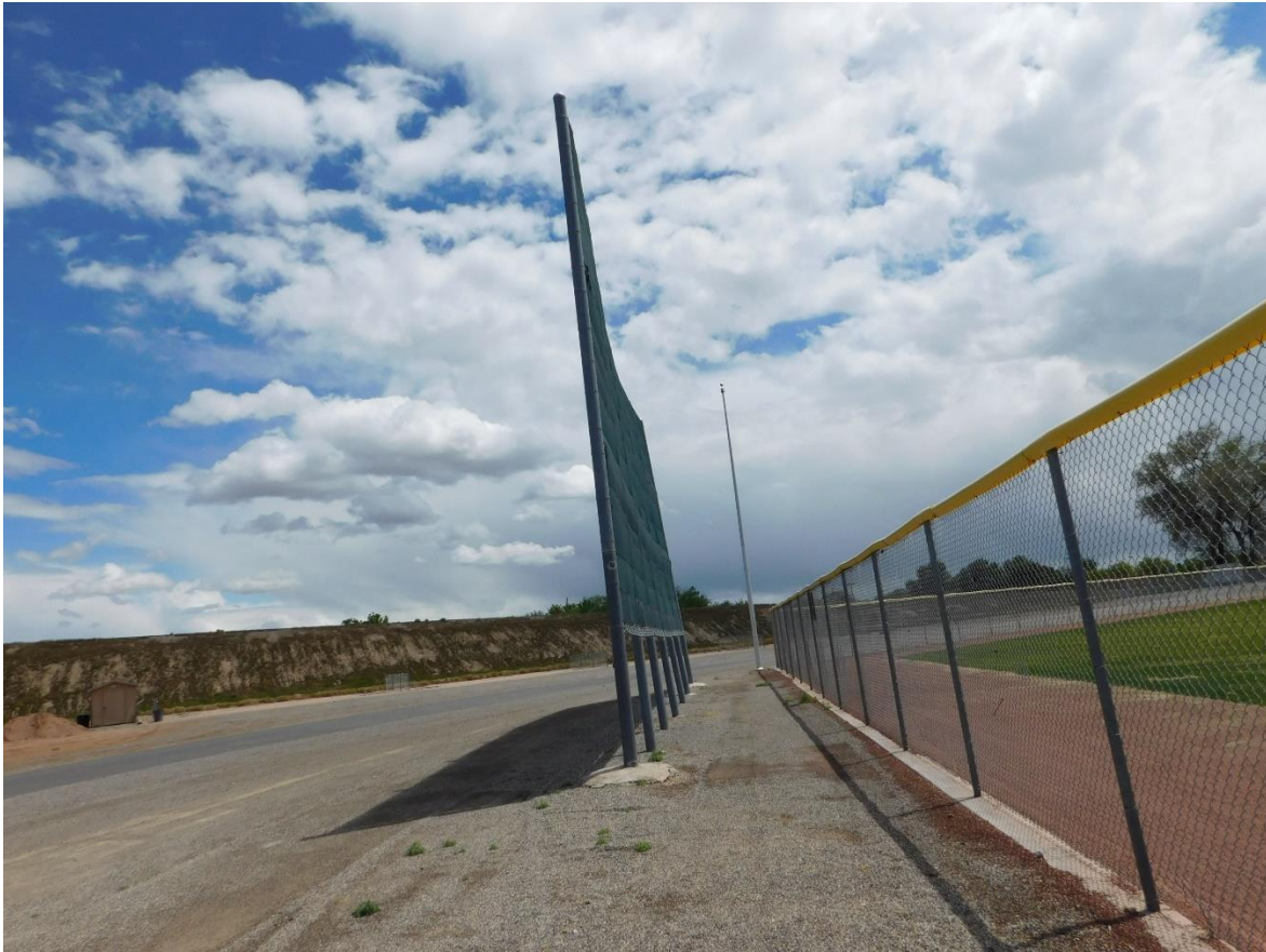
Looking from West to East, supports are bent and no longer plumb
