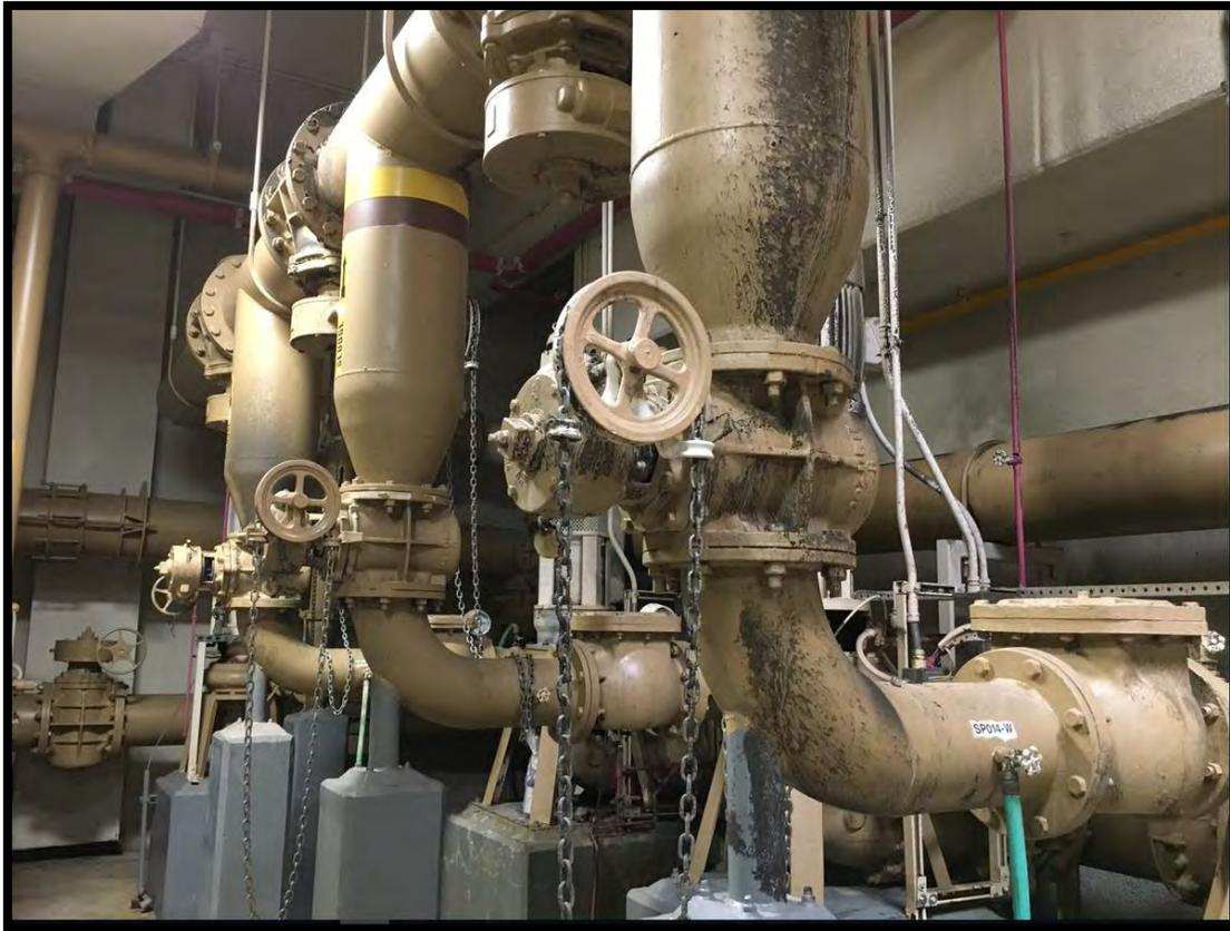
Picture 17, Aerobic Basin Basement Pump Pipe with spray from reducer leak
