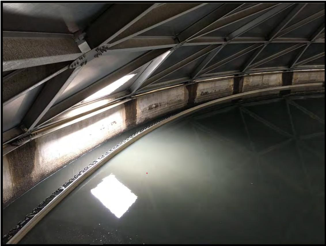
Picture 8, Primary Clarifier Wall and Roof
