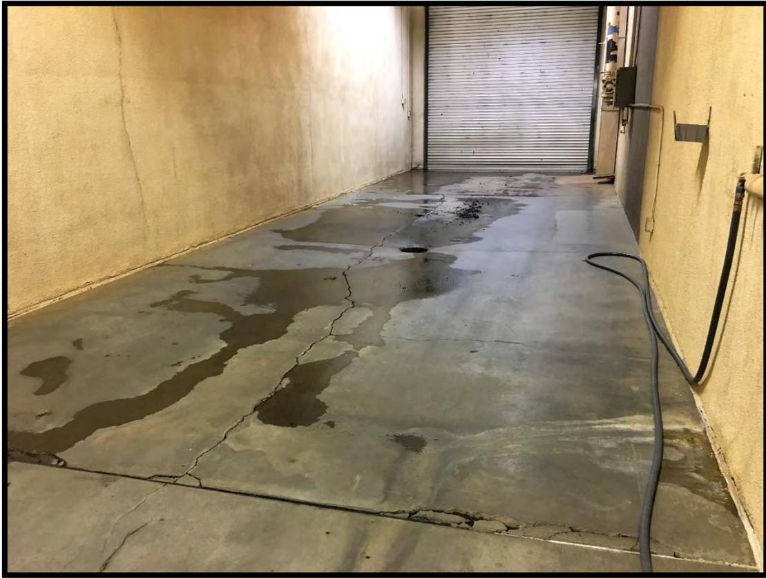
Picture 25, Aerobic Digester Concrete and Wall Cracks (Truck Sludge Loading)
