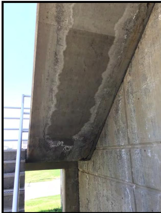
Picture 24, Aerobic Digester Stairway, Rebar erosion in concrete
