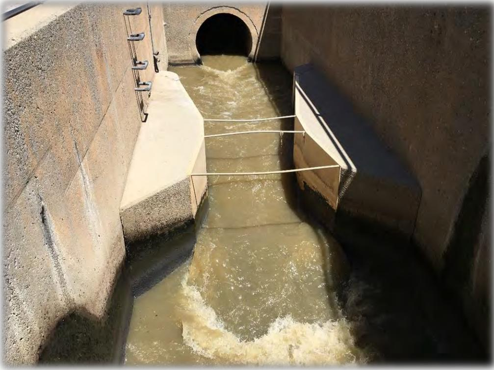
Wastewater enters the Persigo plant at the Headworks through a parshall flume which meters the volume of wastes to be treated.
