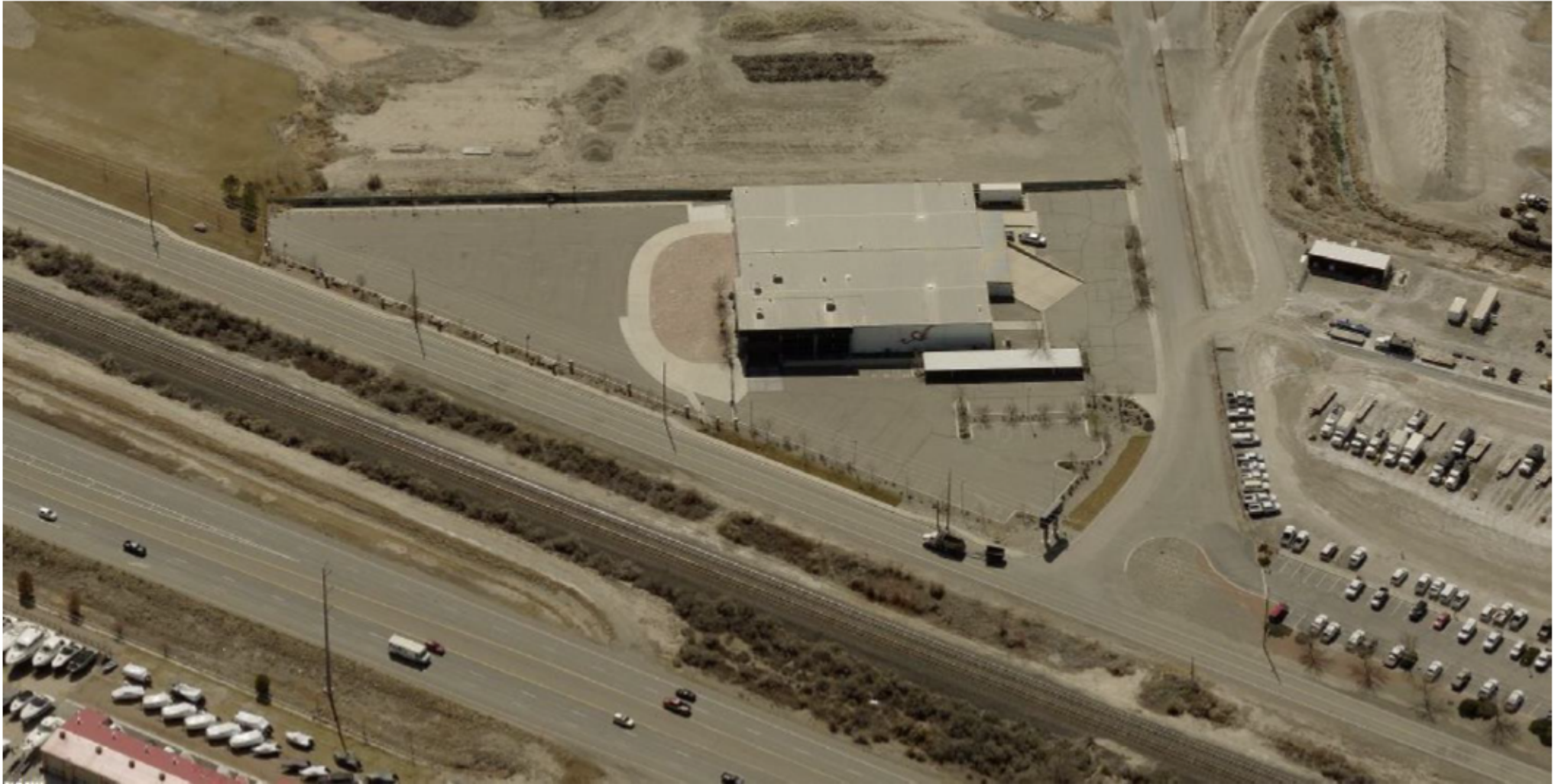
2285 River Road – View Across Site Looking South
