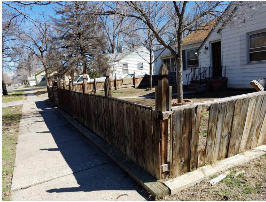
Encouraged Acceptable Fencing
