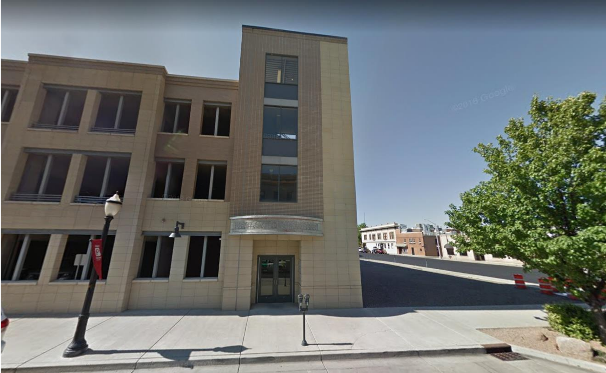
North-Facing Façade of Parking Garage – Showing Location of Elevator/Stairwell Subject Endcap Property on Right
