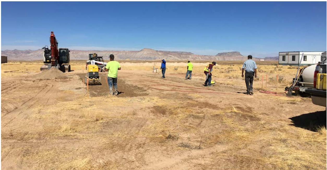
Burn Slab Project Site – Looking north (building foundation under construction)
