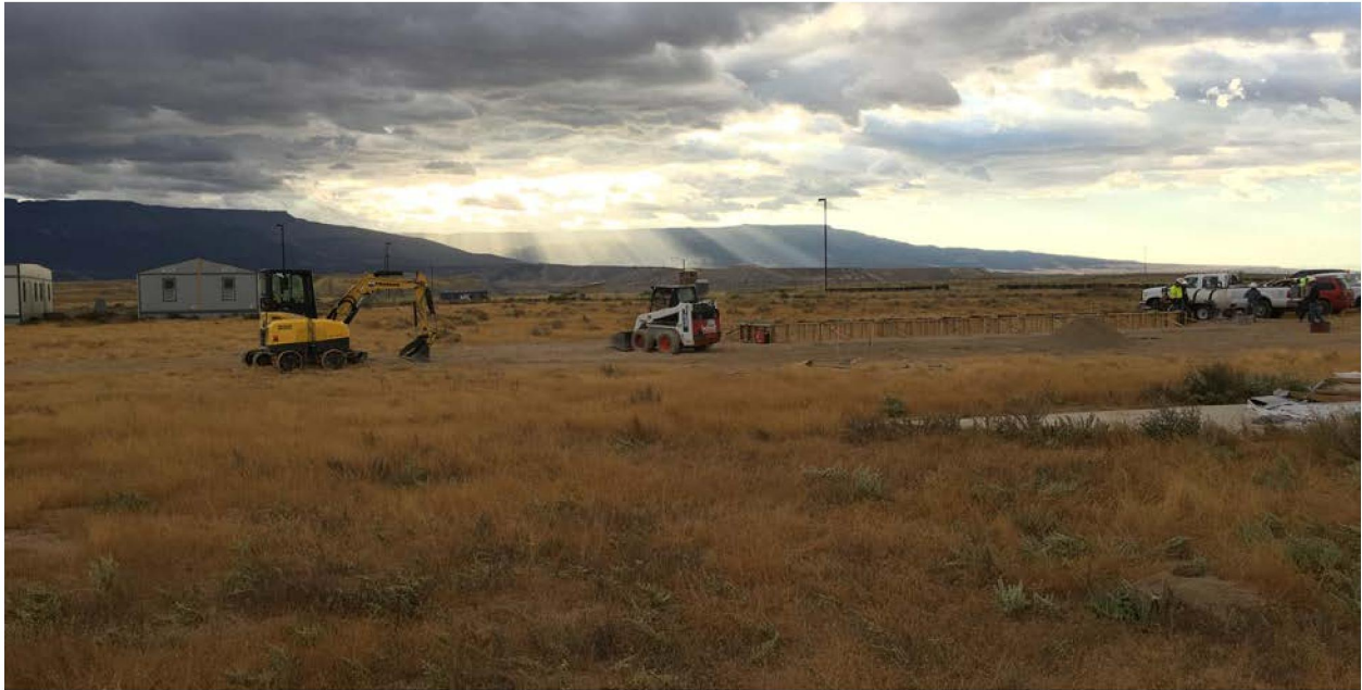
Burn Slab Project Site – Looking southeast
