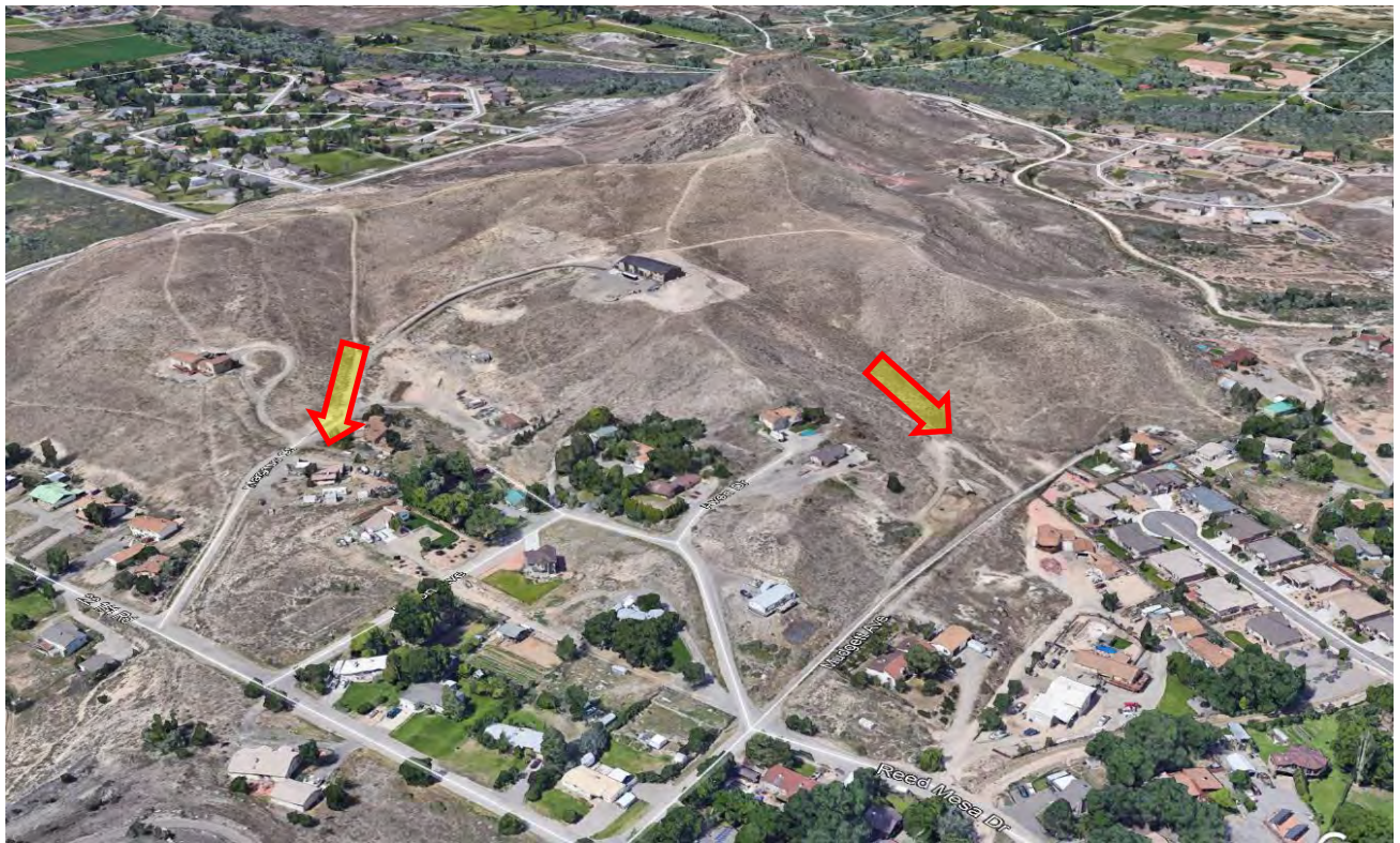
Existing Drainages Along North Edge of Project
