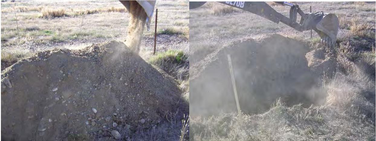
The top 1 foot was generally consistent with that of a sandy clay (CL) material. 1 - 4 feet the material was a pit run, cobble material (SM). 4 – 7 feet the material turned to a decomposed shale material.
