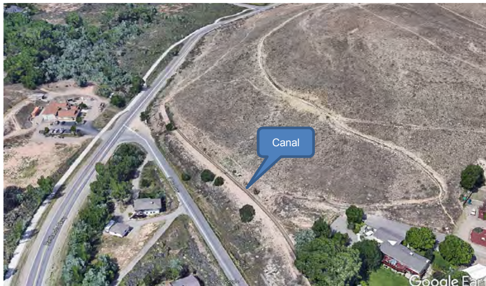
Redlands Second Lift Canal
