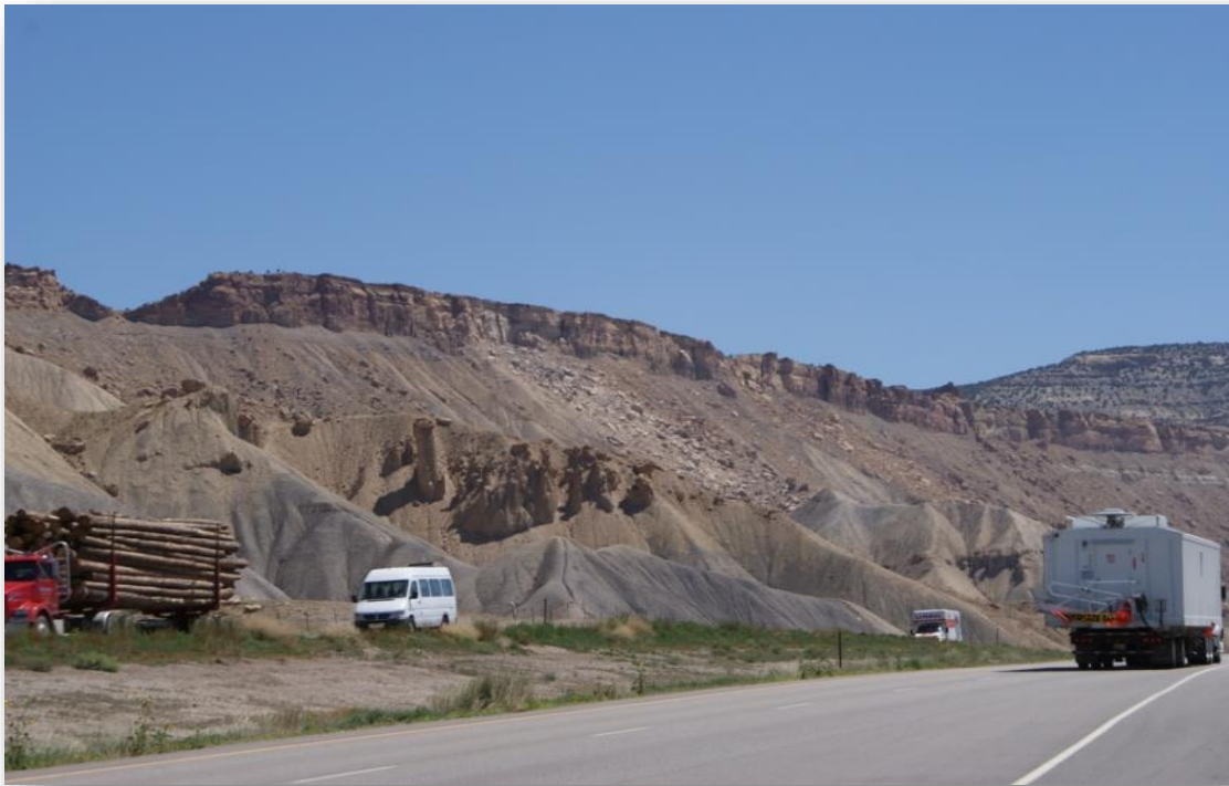
FIGURE 13 ROCKFALL WEST OF PALISADE ALONG INTERSTATE 70
