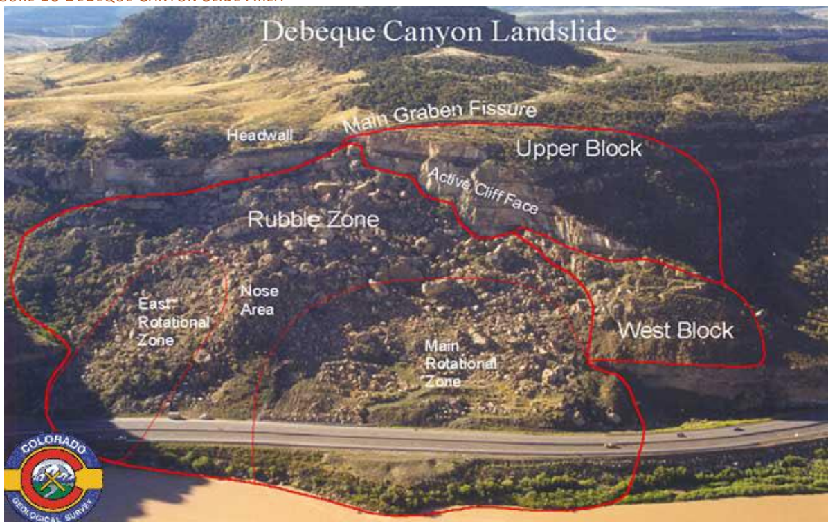
FIGURE 10 DEBEQUE CANYON SLIDE AREA
