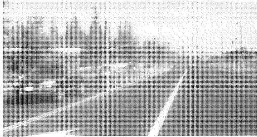
**EXHIBIT 14-14** Installation of flexible pylons to restrict movements on opposite sides of this roadway and permit right-in, right-out only.
