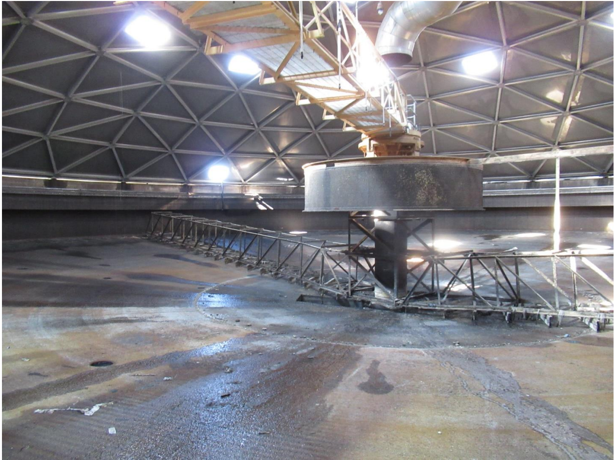
Figure 7. Overall view of clarifier interior.
