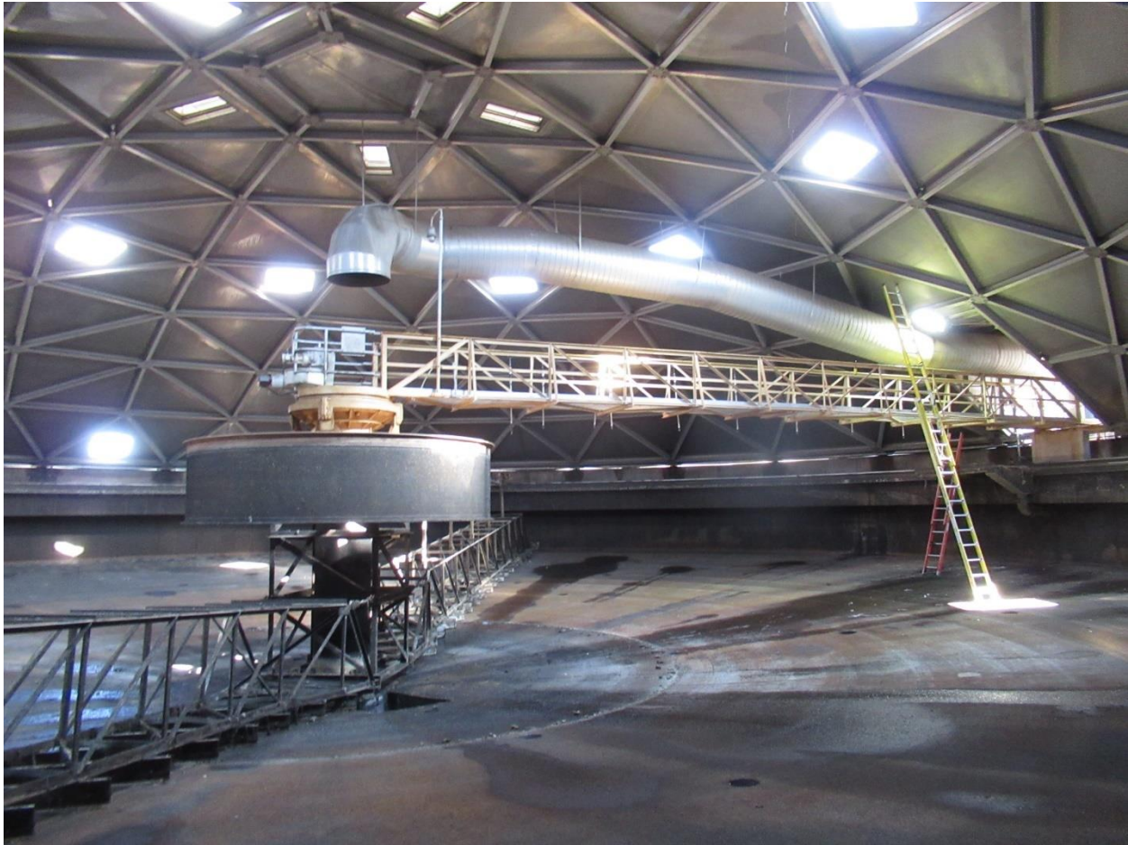
Figure 9. Overall view of clarifier interior.
