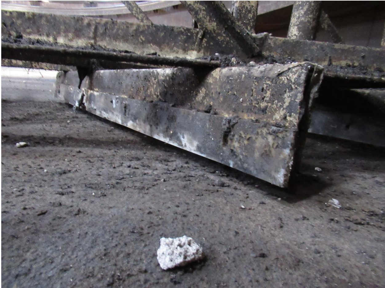
Figure 26. Close-up of bottom screed plate. Blade height will be adjusted by Owner.
