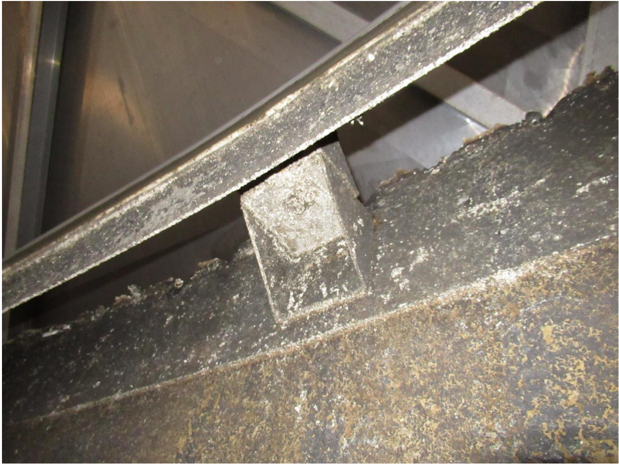
Figure 18. Close-up view of weir plate to scum baffle connection.
