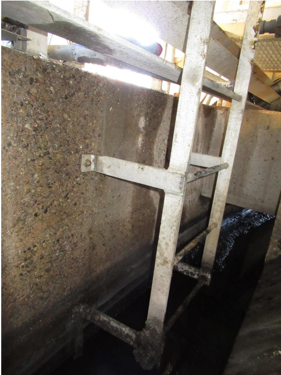
Figure 20. Ladder at entry viewed from trough.
