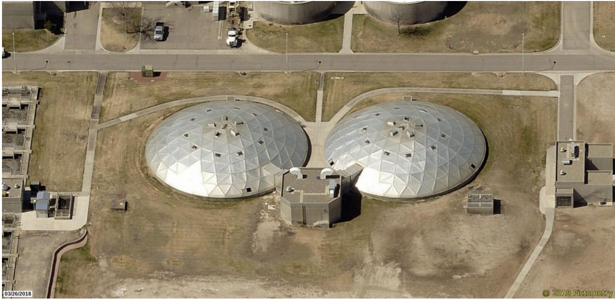
Figure 4. View of Primary Clarifiers looking west (photo from Pictometry, taken 3/26/2018).
