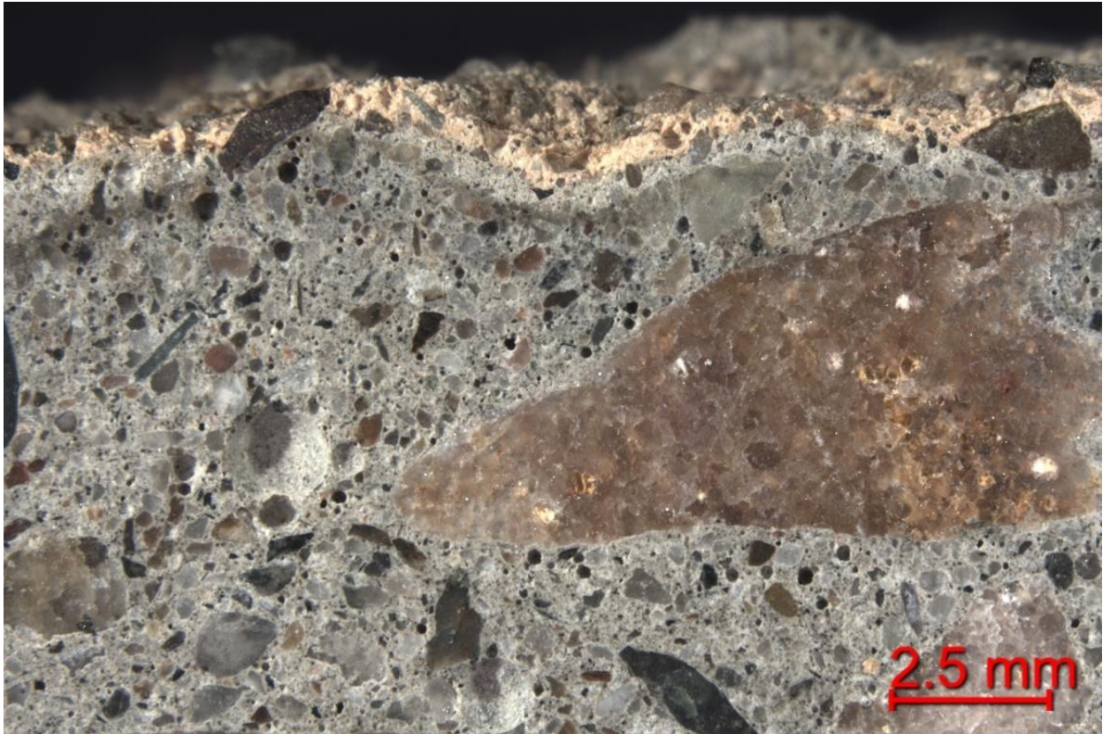
Figure 35. Near surface showing discoloration (Core 1) taken from within trough.
