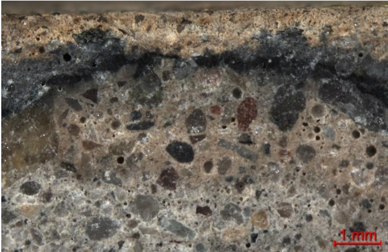
Figure 36. Near surface showing discoloration (Core 3) taken from within lower portion of basin.
