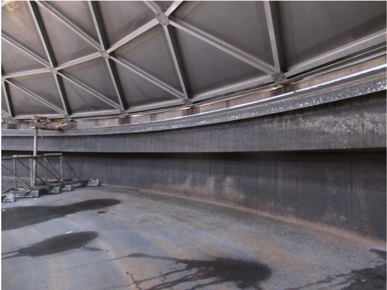
Figure 12. Interior view of exterior clarifier wall and trough.
