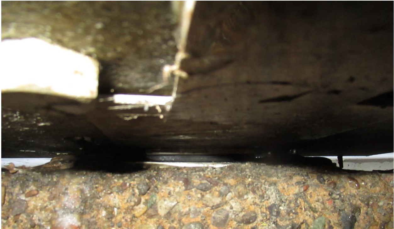
Figure 33. Close-up view of underside of dome node connection hardware.
