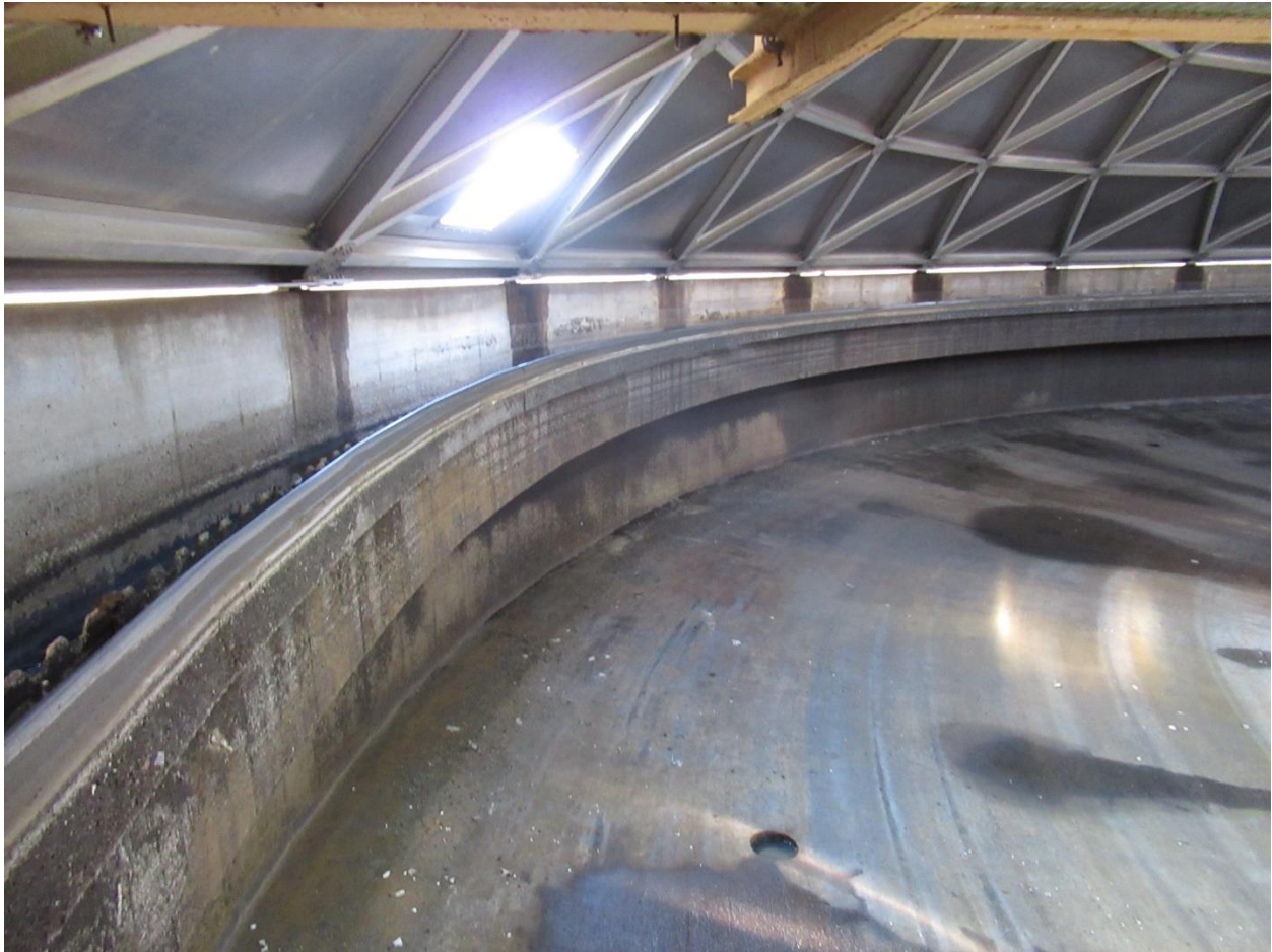
Figure 29. Overall view of trough.
