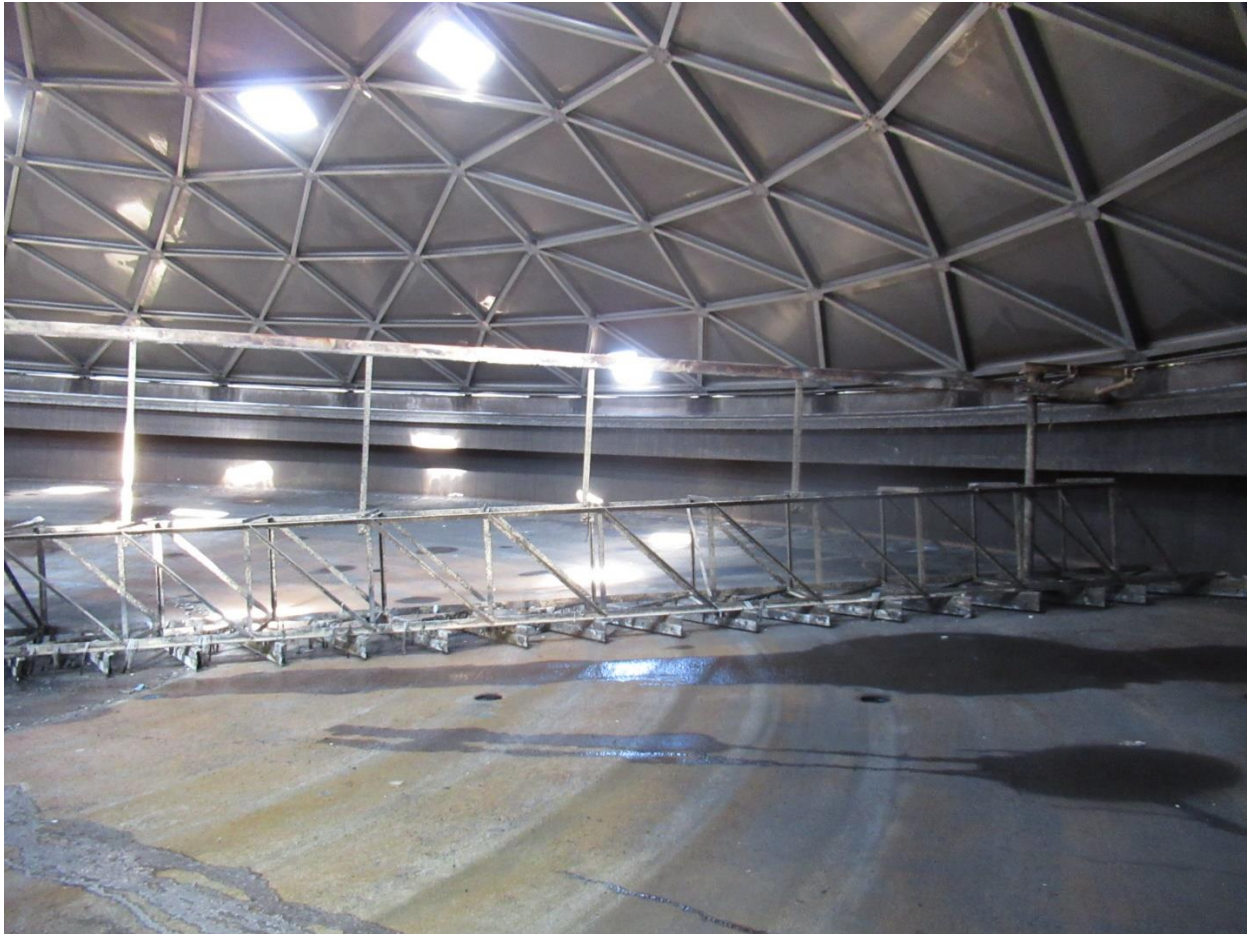
Figure 8. Overall view of clarifier interior.
