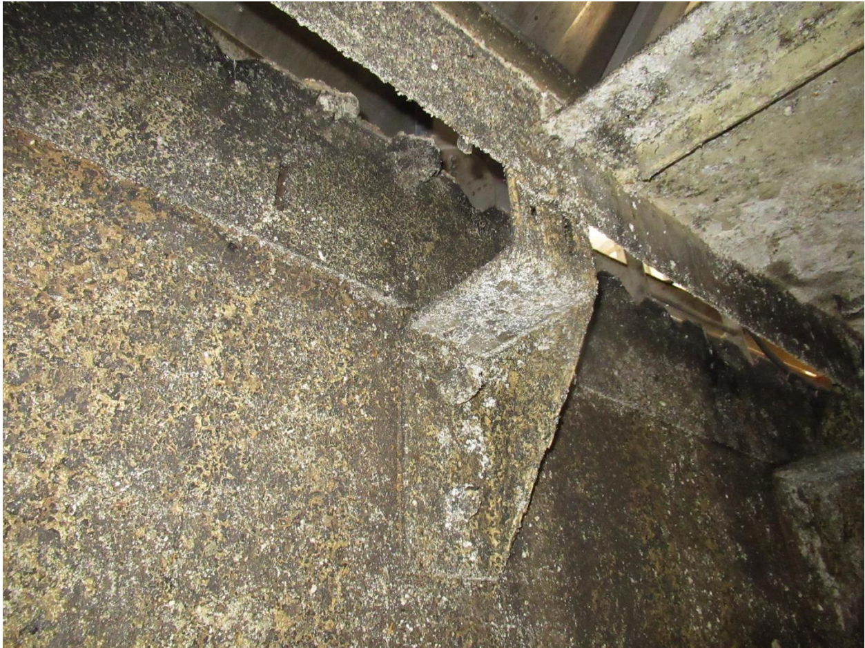
Figure 15. Scum box connection to exterior wall of trough.
