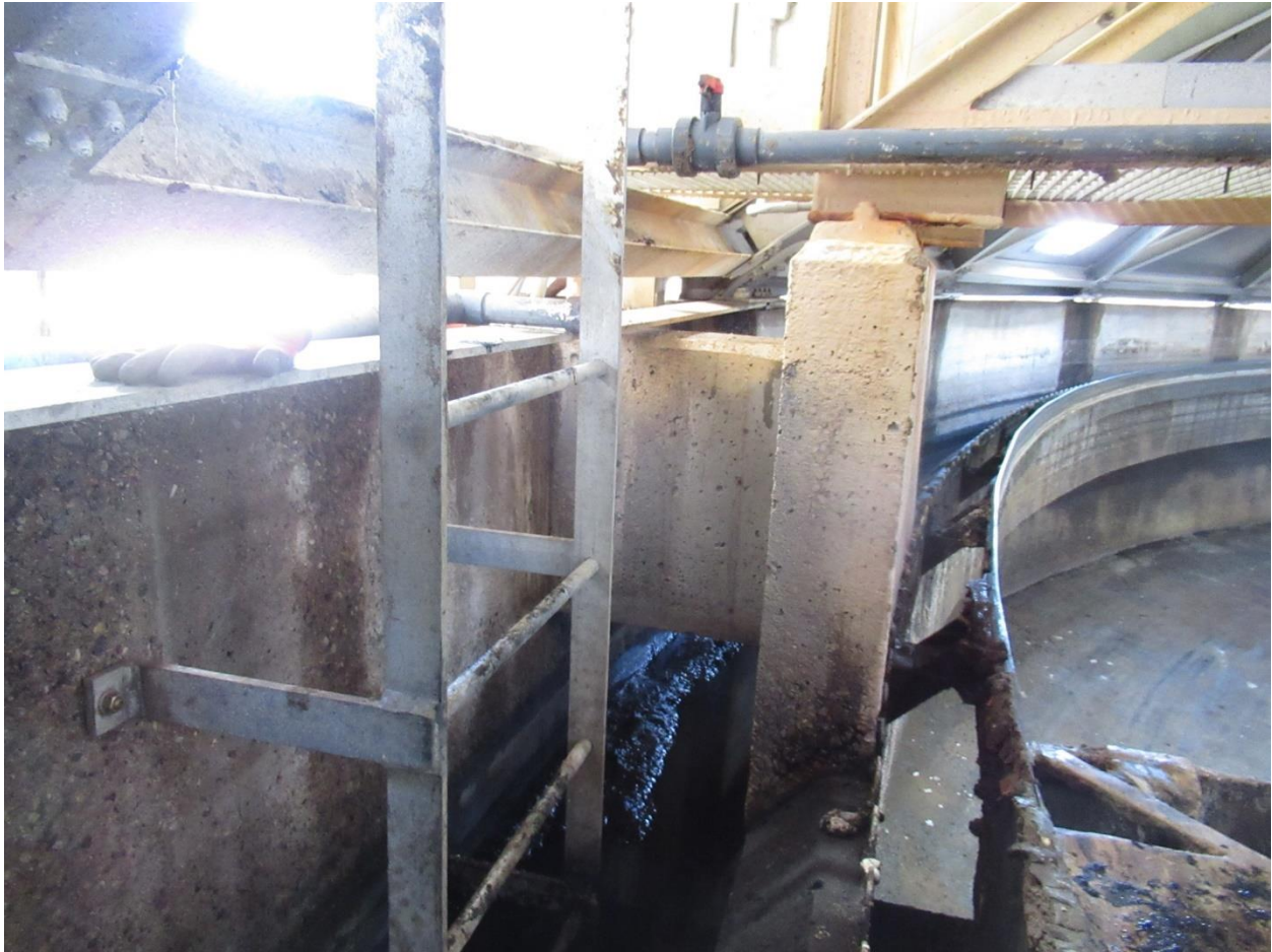
Figure 21. Catwalk bridge support pier.
