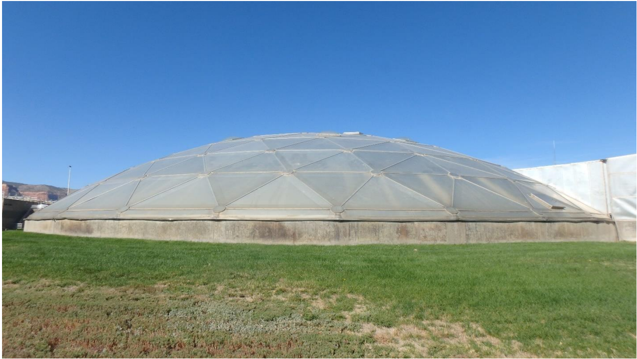
Figure 6. Clarifier No. 2 as viewed from the east side looking west.
