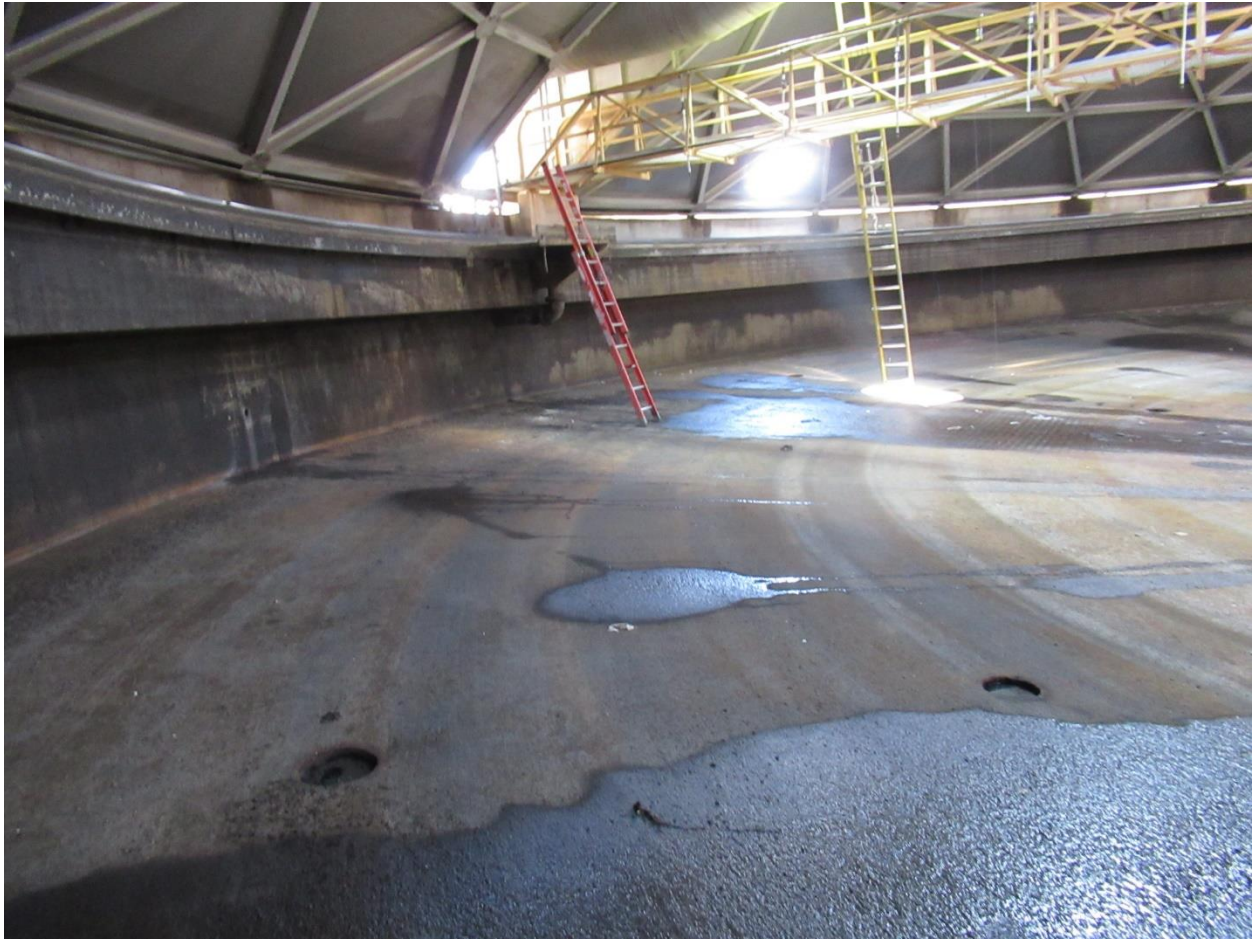
Figure 11. Overall view of clarifier interior.
