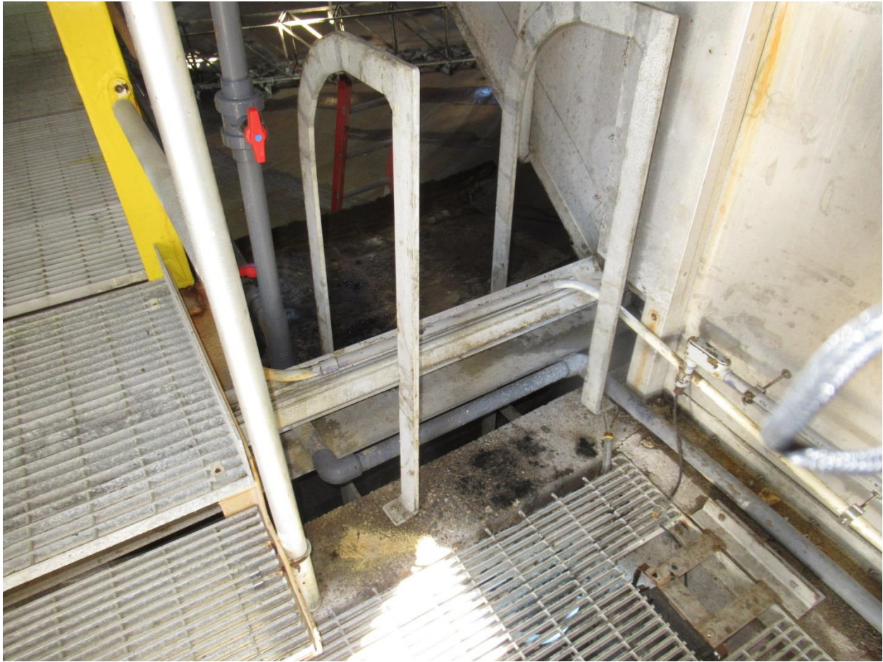
Figure 19. Trough access ladder as viewed from above, standing in entrance enclosure.
