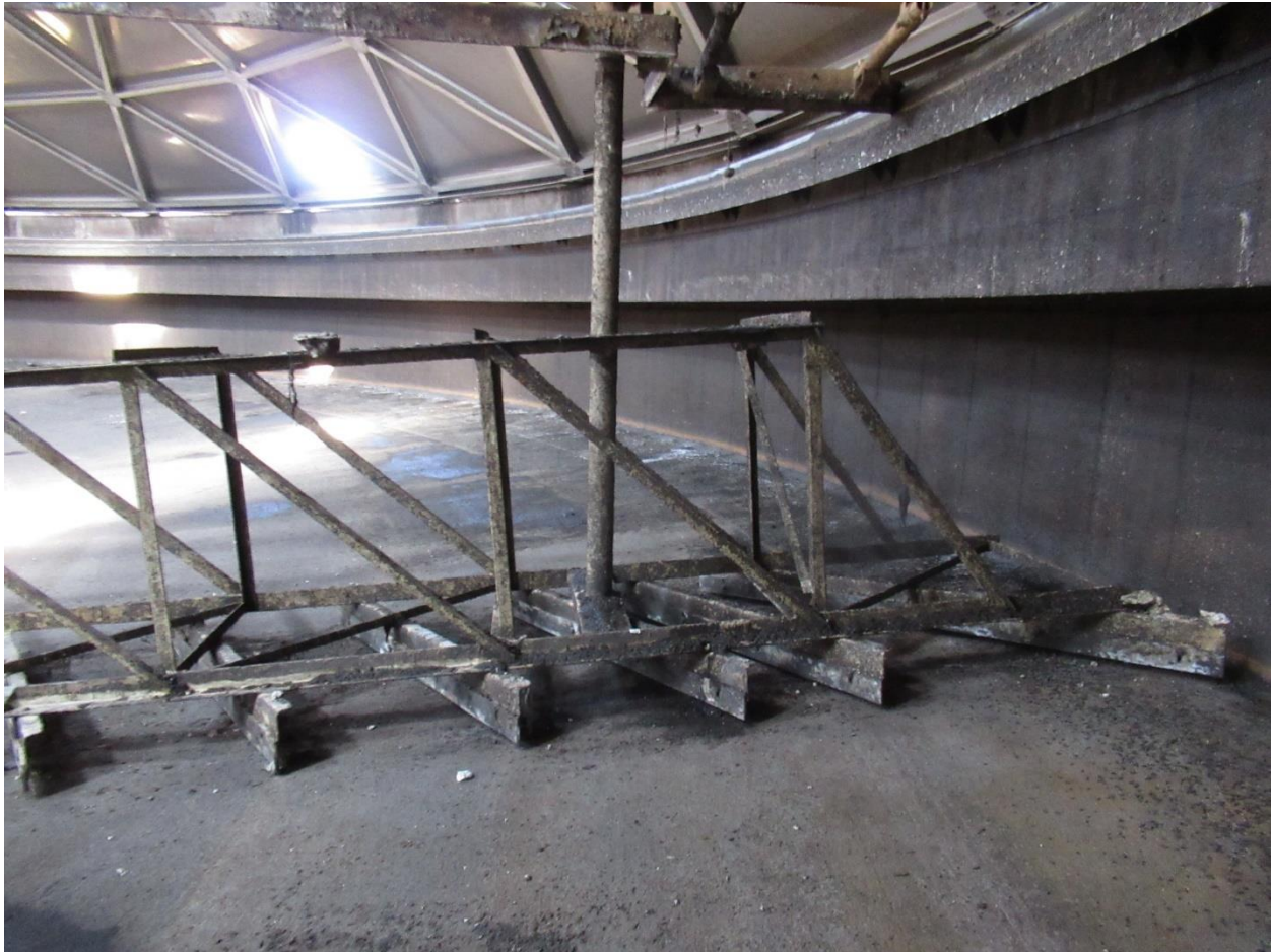
Figure 25. Bottom screed and blades at exterior wall.
