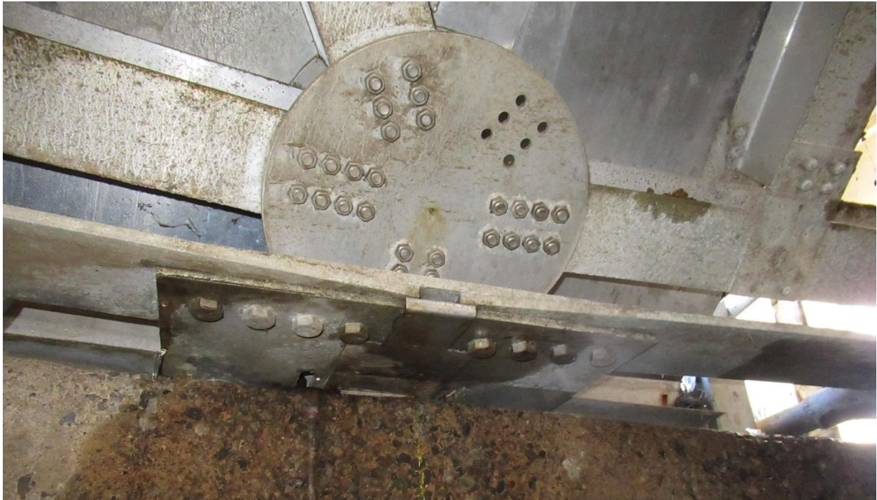
Figure 31. Typical dome-to-clarifier wall connection node.
