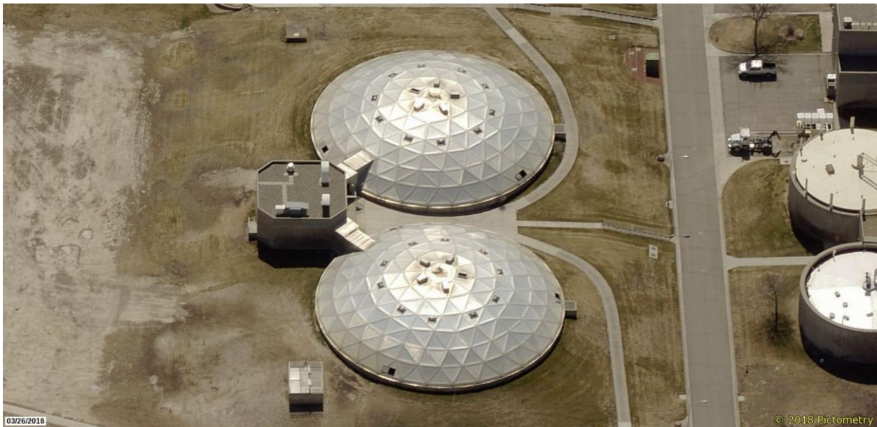
Figure 3. View of Primary Clarifiers looking south (photo from Pictometry, taken 3/26/2018).
