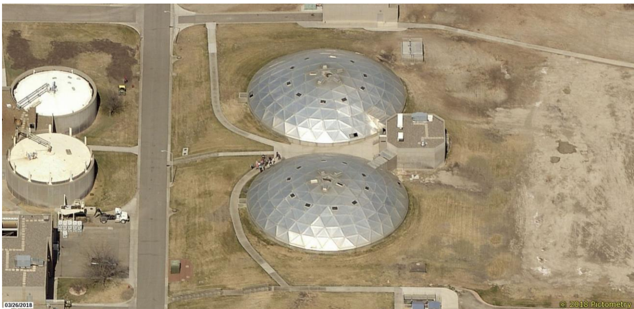
Figure 5. View of Primary Clarifiers looking north (photo from Pictometry, taken 3/26/2018).
