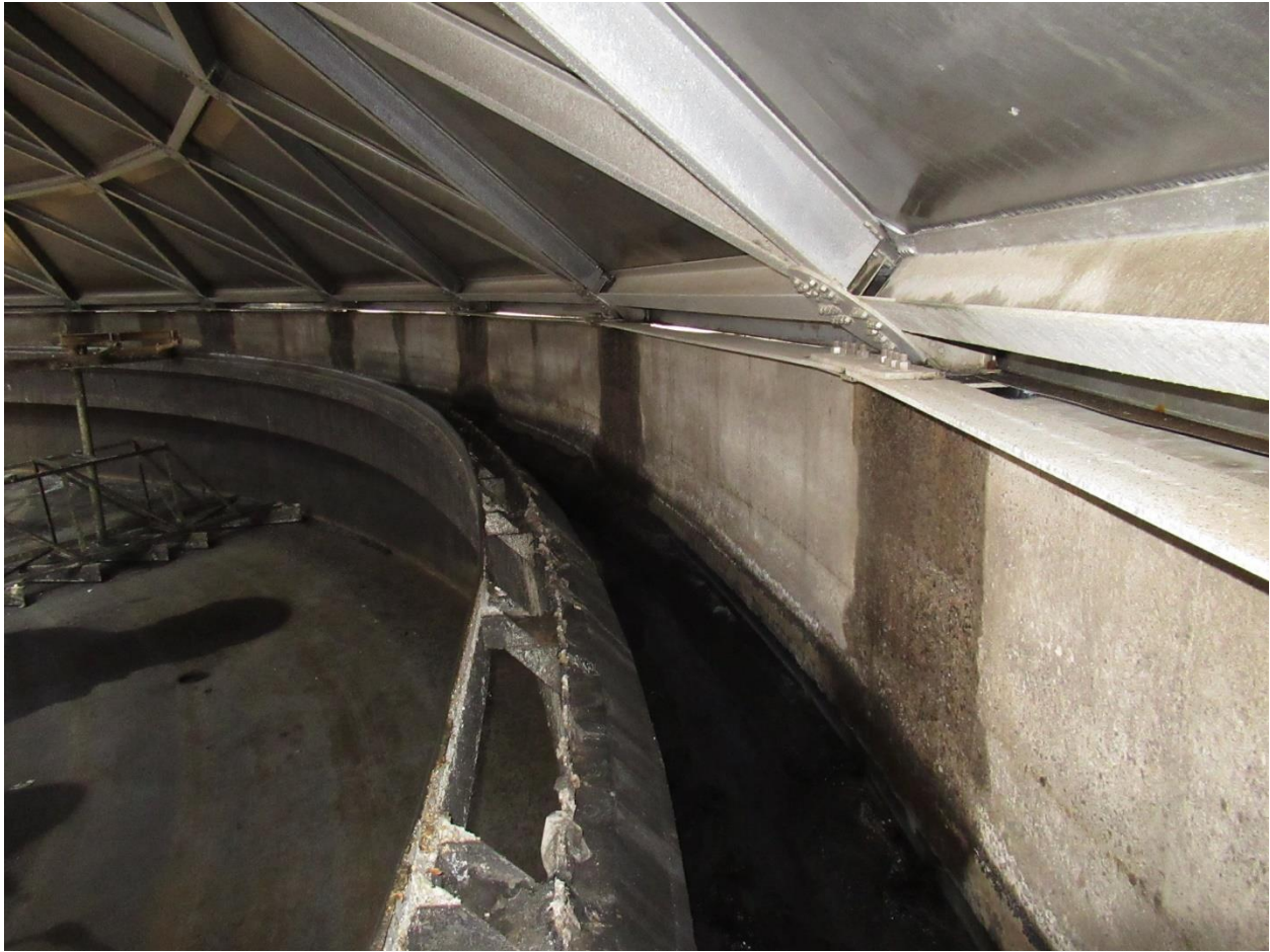
Figure 28. Overall view of trough and weir plate.
