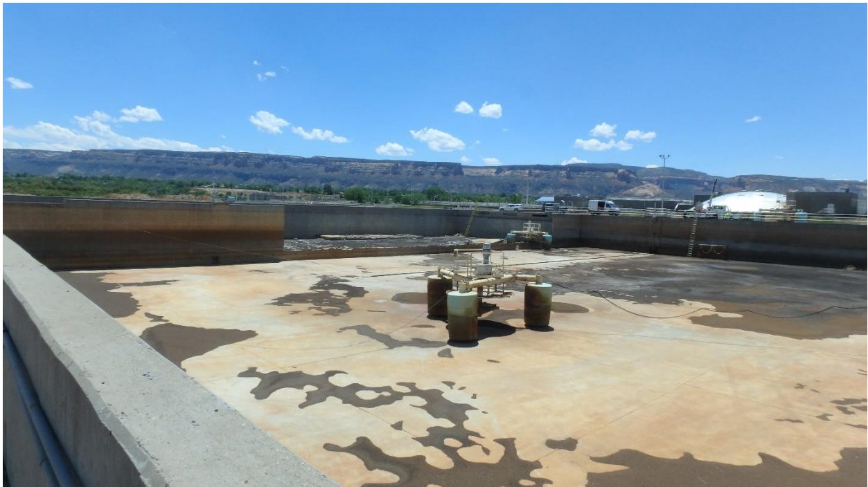
Figure 4. Overall view of the south dividing wall (June 2020)
