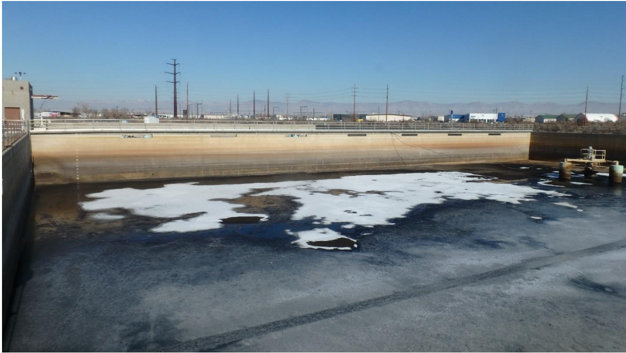
Figure 1. Overall view of north dividing wall (January 2020).
