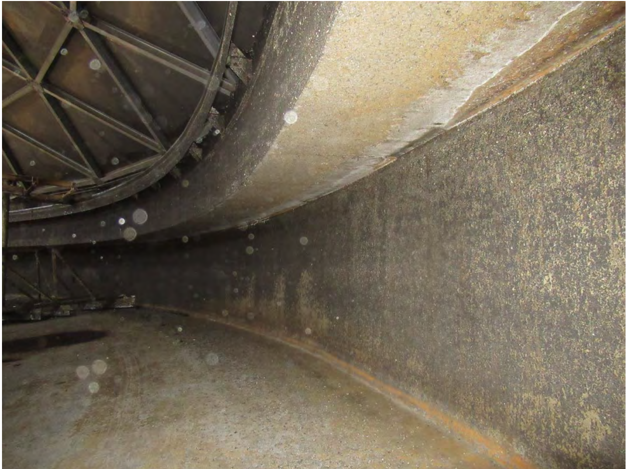
Figure 13. Interior view of exterior clarifier wall and trough.
