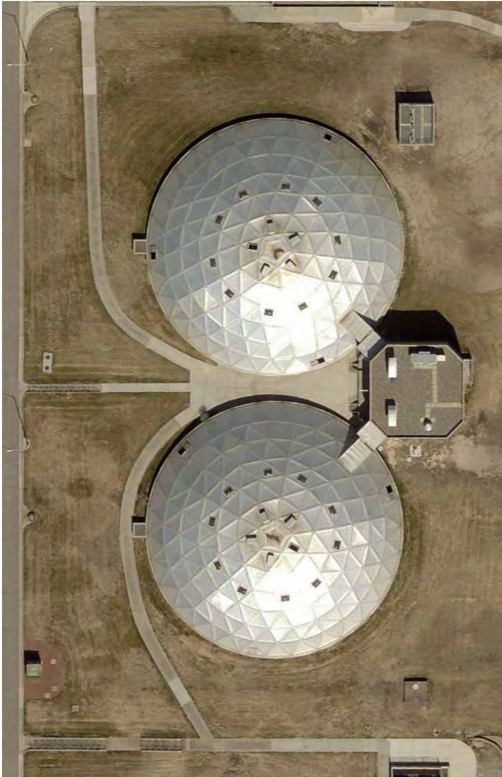
Figure 1. View of Primary Clarifiers from above, north is up (photo from Pictometry, taken 3/26/2018).
