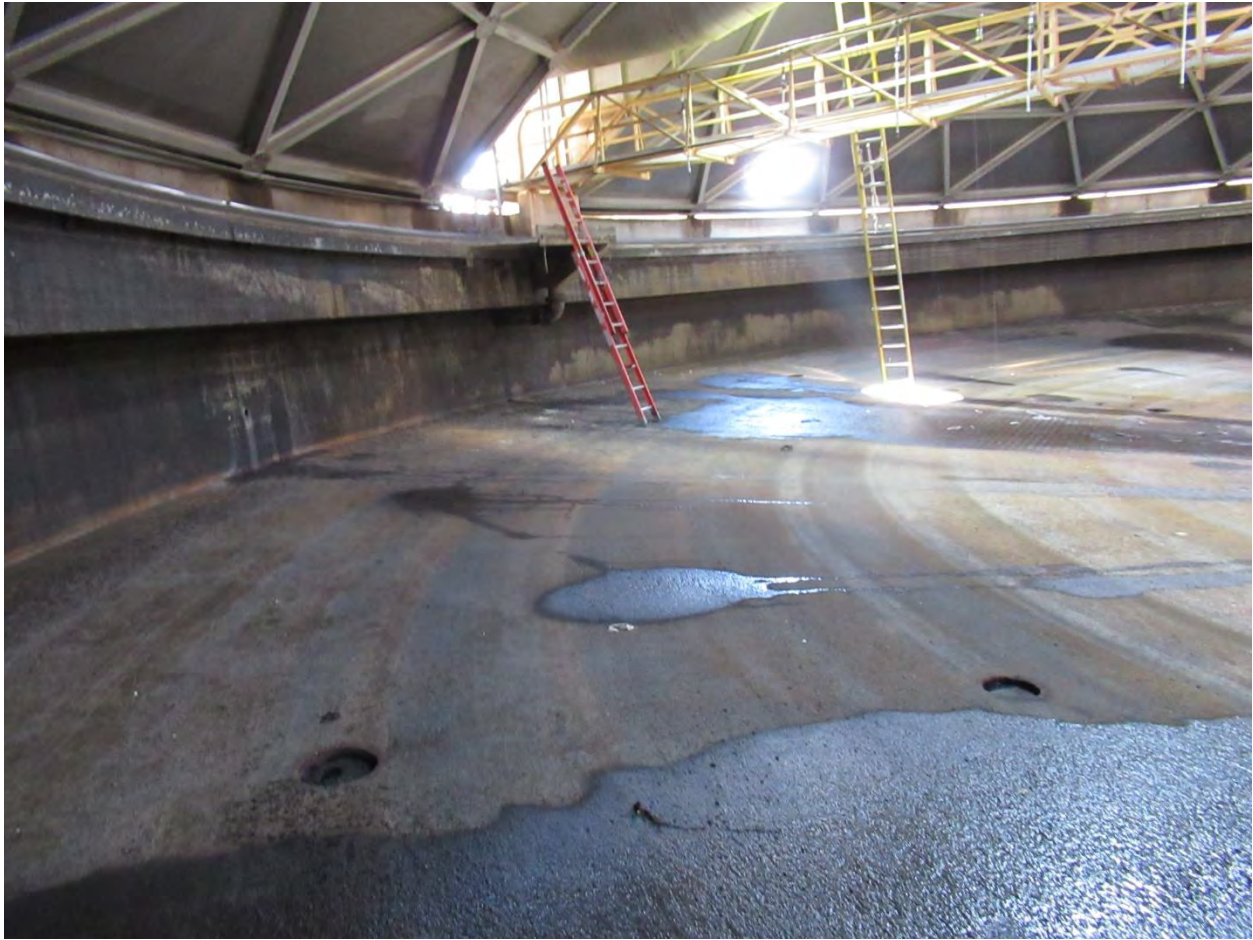
Figure 11. Overall view of clarifier interior.
