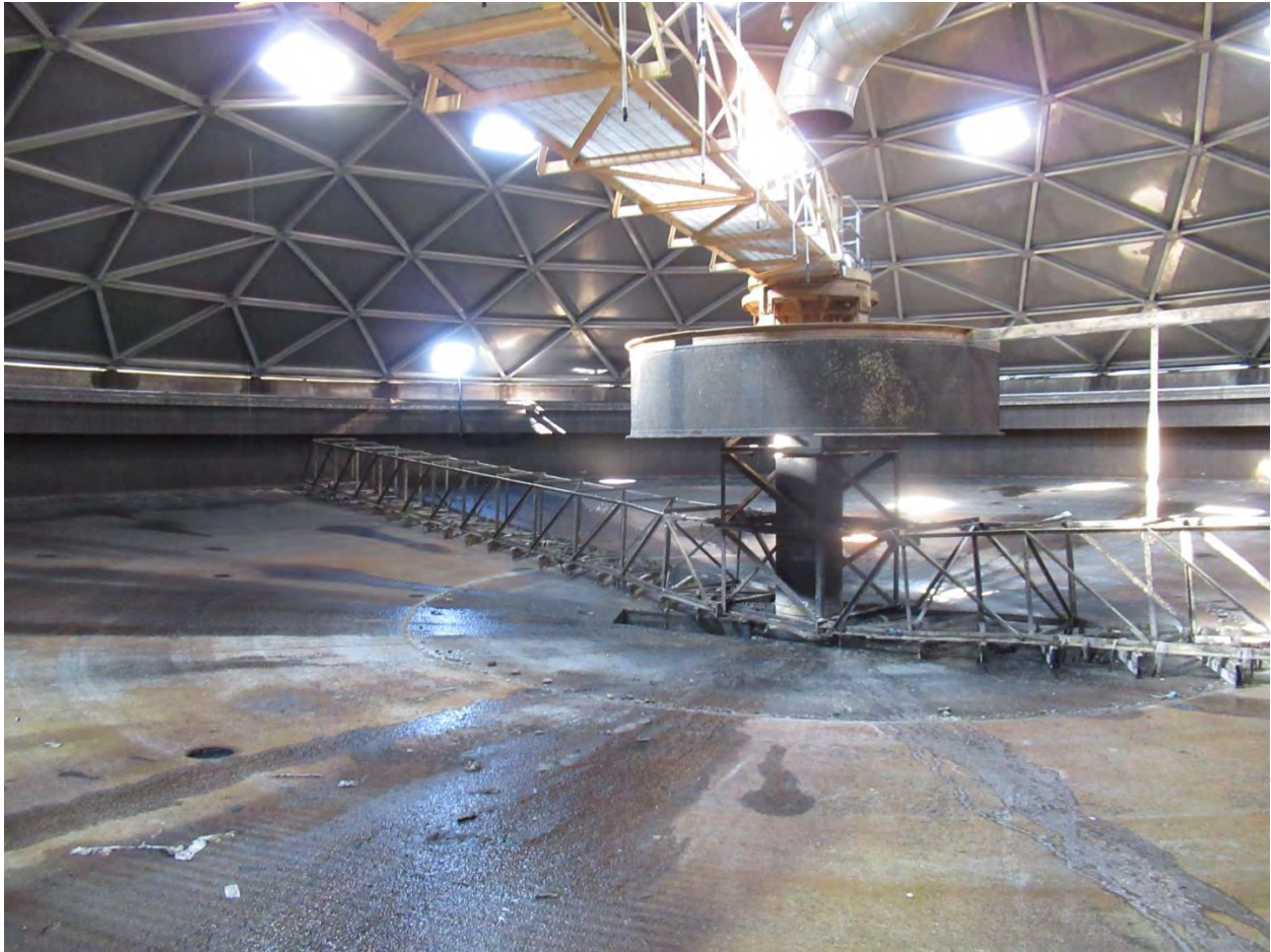
Figure 7. Overall view of clarifier interior.
