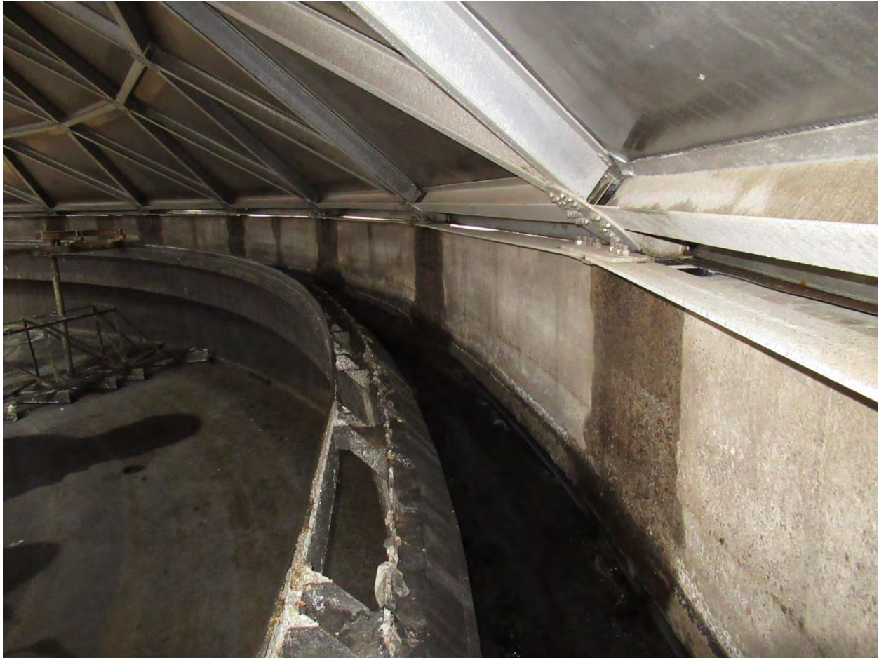
Figure 28. Overall view of trough and weir plate.
