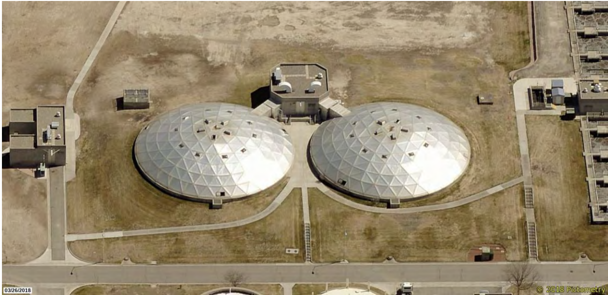
Figure 2. View of Primary Clarifiers looking east (photo from Pictometry, taken 3/26/2018).
