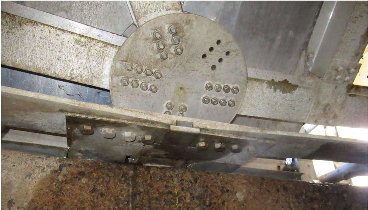
Figure 31. Typical dome-to-clarifier wall connection node.
