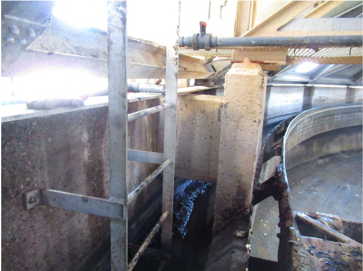
Figure 21. Catwalk bridge support pier.
