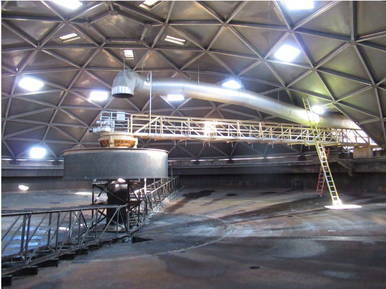
Figure 9. Overall view of clarifier interior.
