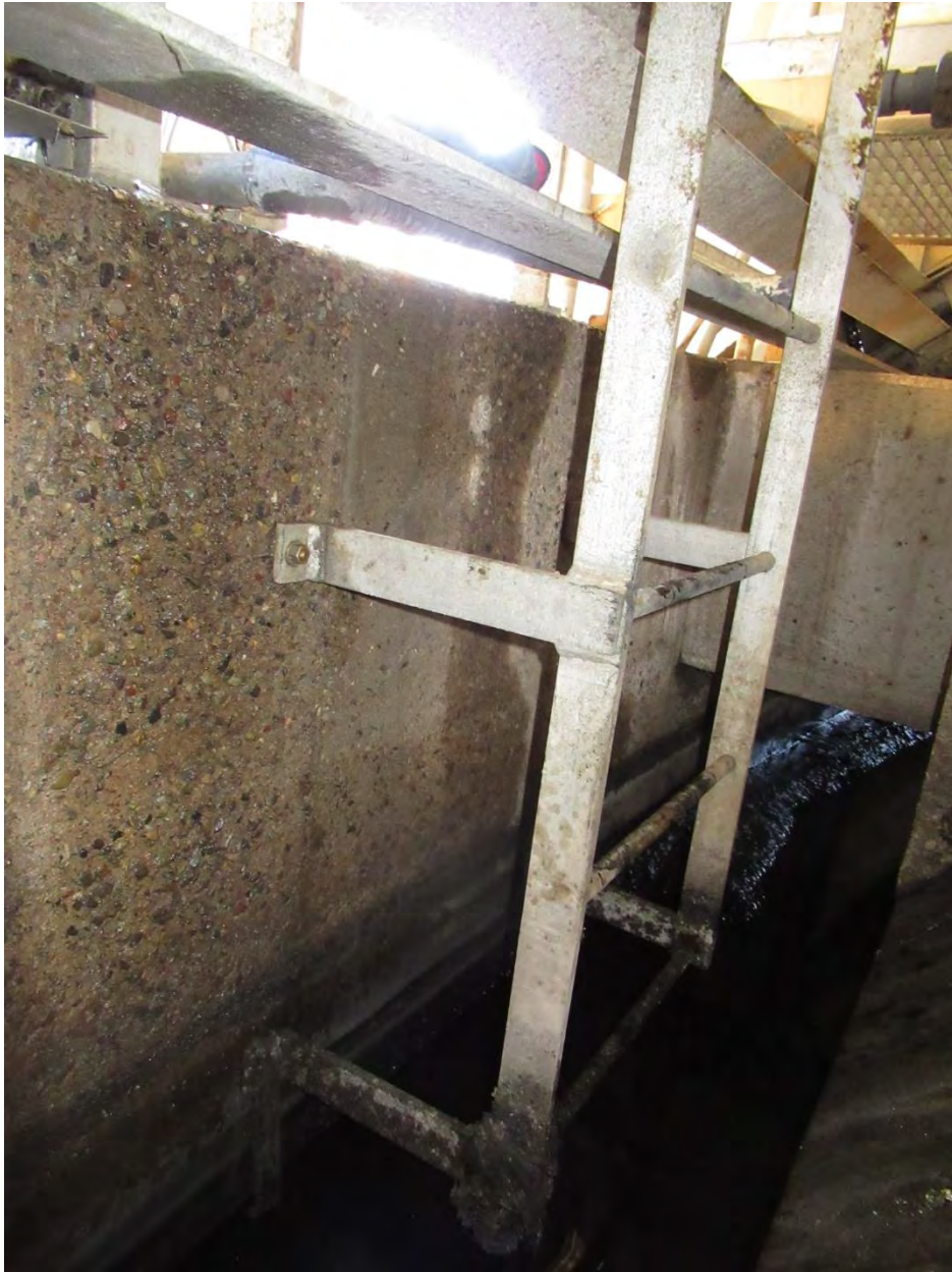
Figure 20. Ladder at entry viewed from trough.
