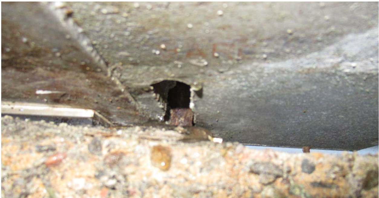
Figure 34. Close-up view of underside of dome node connection hardware.
