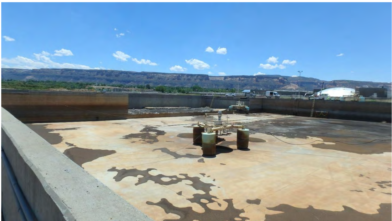
Figure 4. Overall view of the south dividing wall (June 2020)
