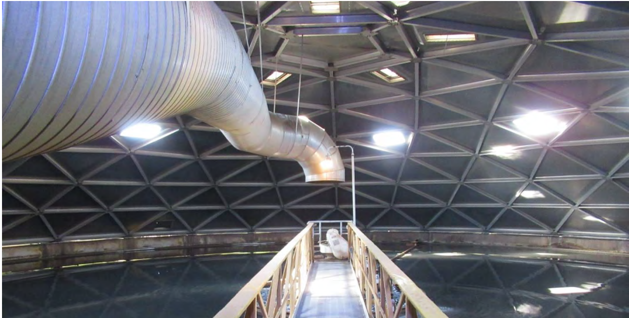
Figure 10. View from catwalk bridge, showing ventilation pipe and dome.
