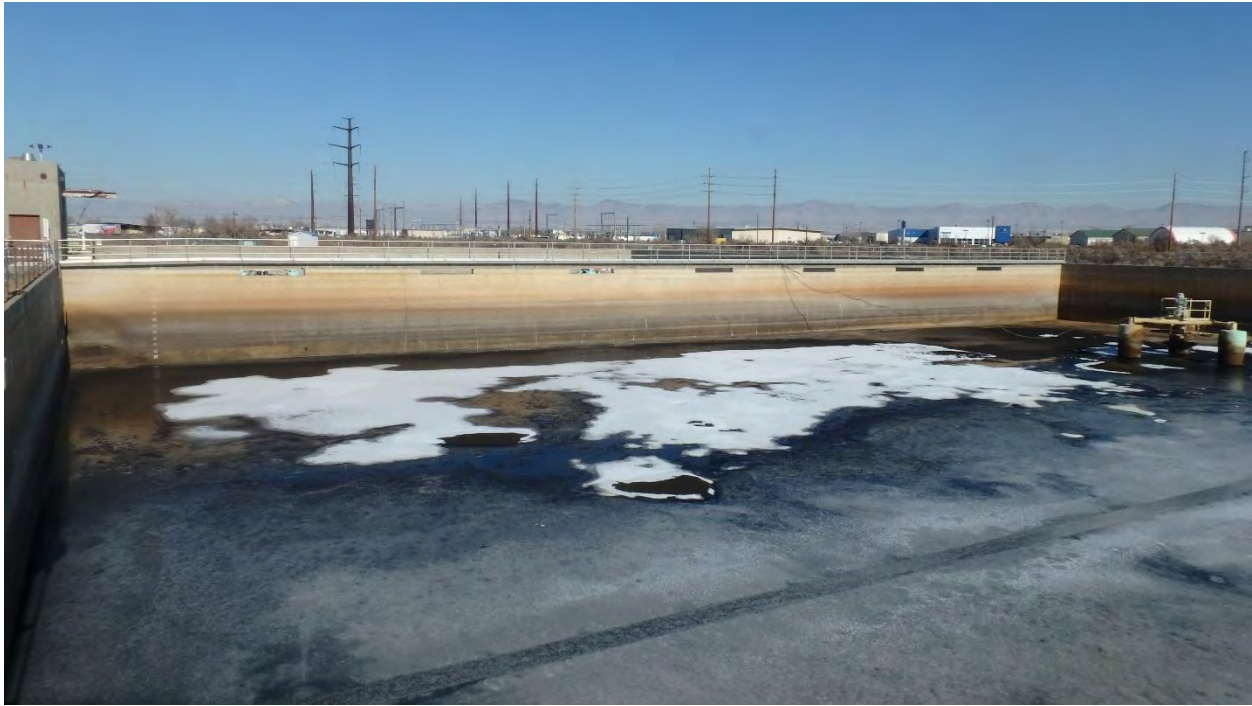
Figure 1. Overall view of north dividing wall (January 2020).
