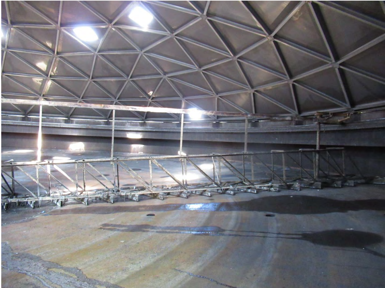
Figure 8. Overall view of clarifier interior.
