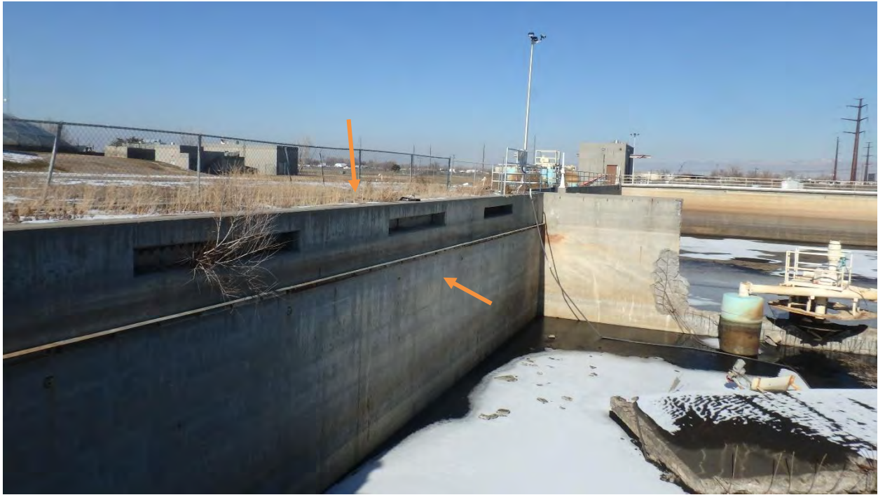
Figure 7. Chlorine contract area/chamber adjacent to south wall which has been filled with soil.
