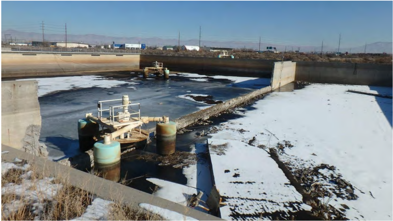
Figure 3. Overall view of the south dividing wall (January 2020).
