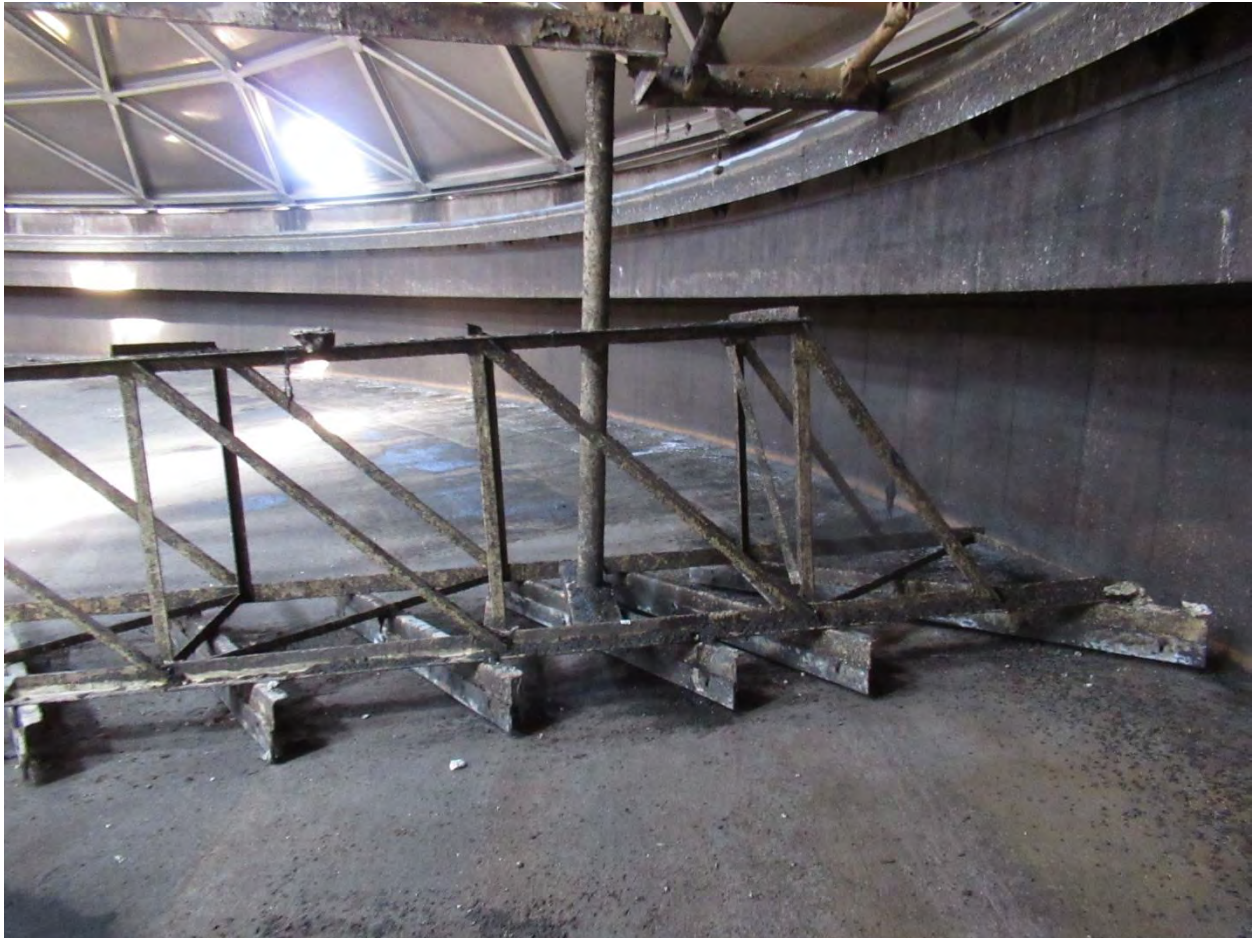
Figure 25. Bottom screed and blades at exterior wall.
