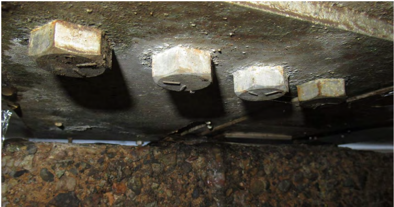
Figure 32. Close-up view of underside of dome node connection hardware.
