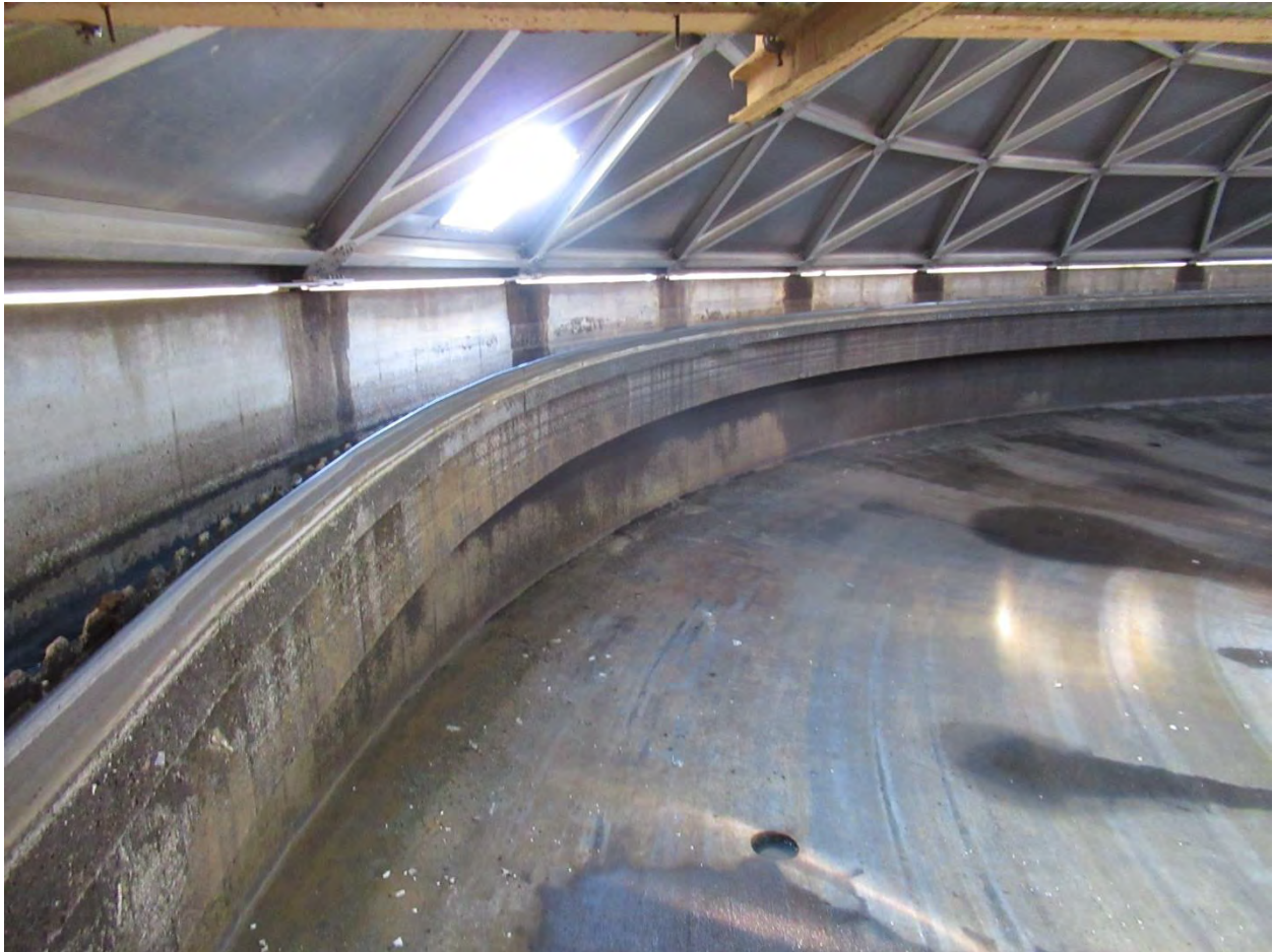
Figure 29. Overall view of trough.
