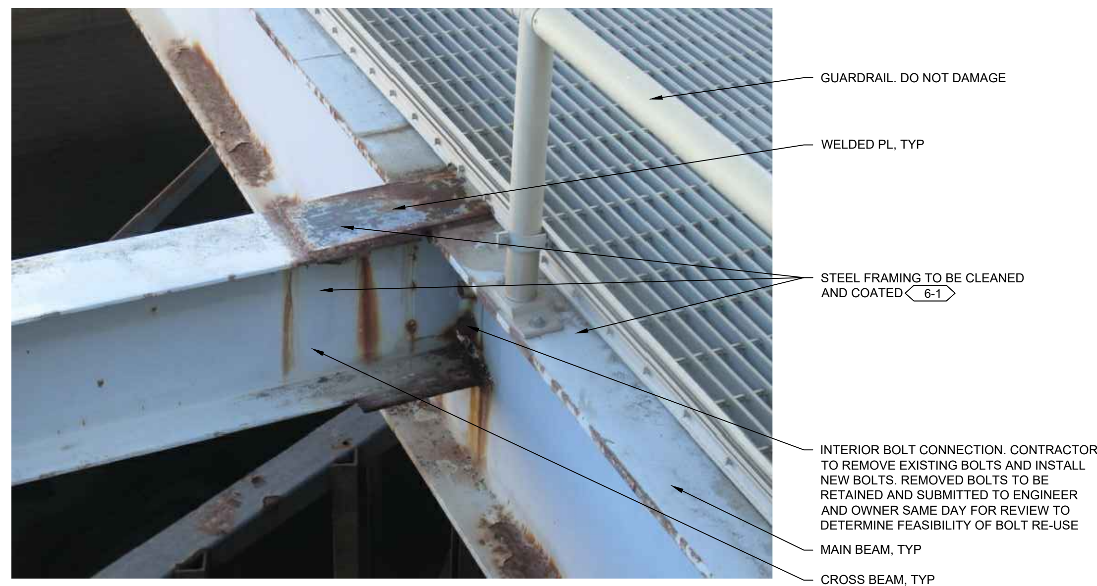
4 Typical Interior Connection Detail SCALE: NOT TO SCALE
