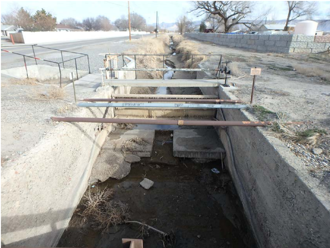
View Looking Upstream
