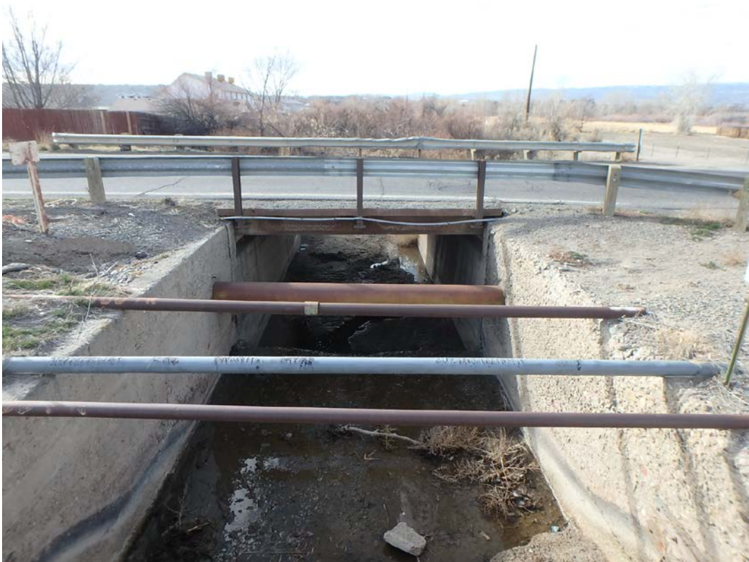
View of Bridge Side Elevation Looking Downstream
