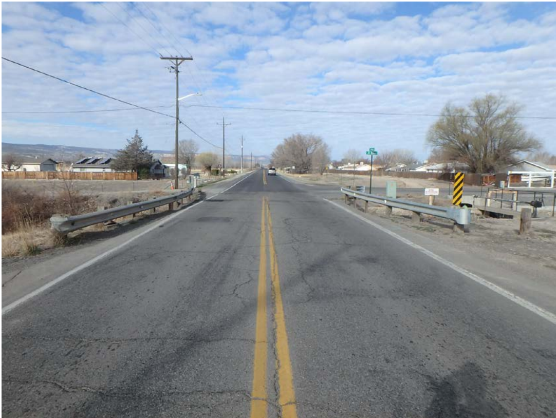
View Down Centerline of Roadway Looking West
