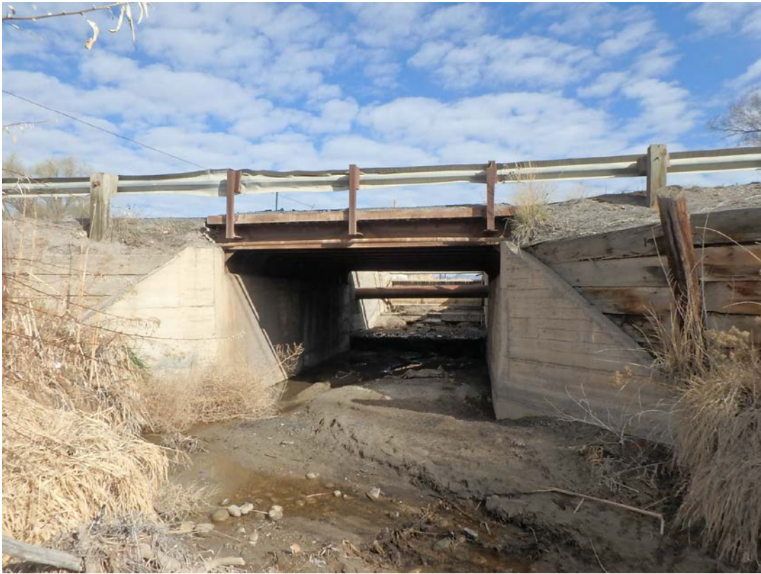
View of Bridge Side Elevation Looking Upstream
