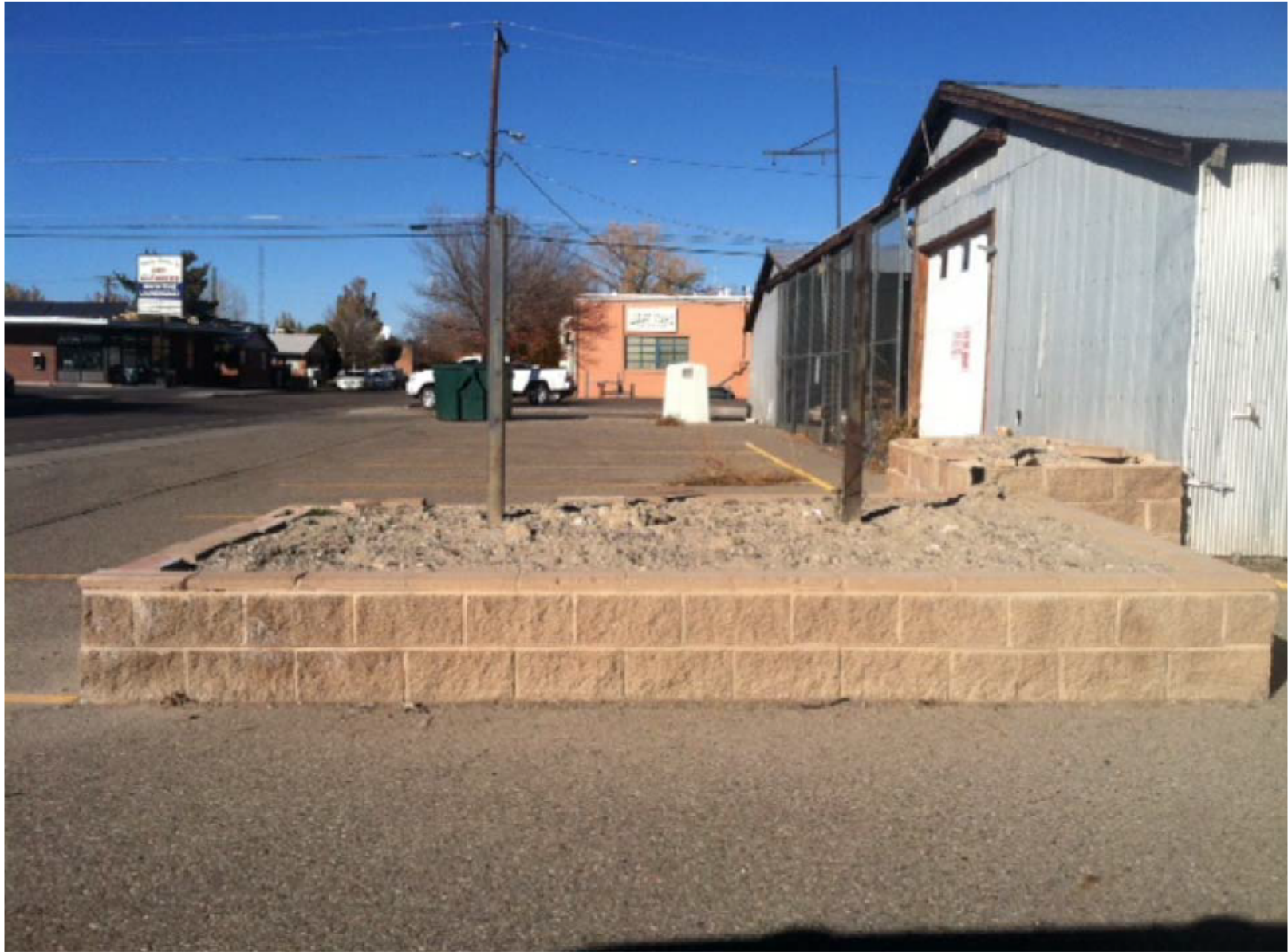
EXISTING SIGN POSTS
