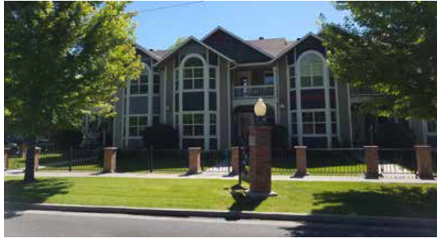
New building broken up into smaller segments; taller masses away from the street; design characteristics unique but relate to the neighborhood.
