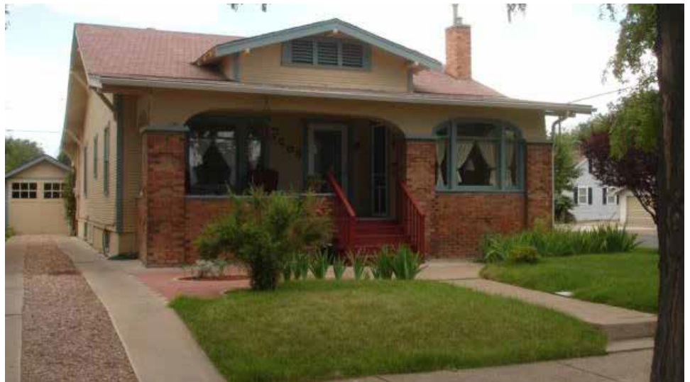
Primary entrance is elevated with stairs, and in this case – like many in the neighborhood - the home is adorned with an elevated front porch. This one is open, some are screened or fully enclosed.
