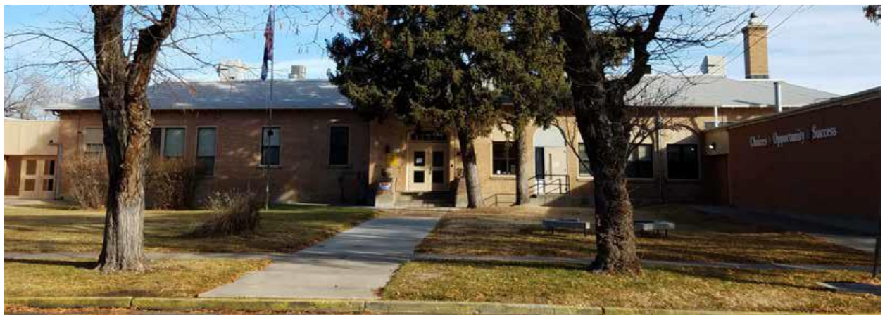
The historic Lincoln Park School was built in 1910 of brick construction with a gable or hip roof. Although there have been several additions to the school throughout the years, the core of the original building remains and shall be preserved and adaptive reuse encouraged.
