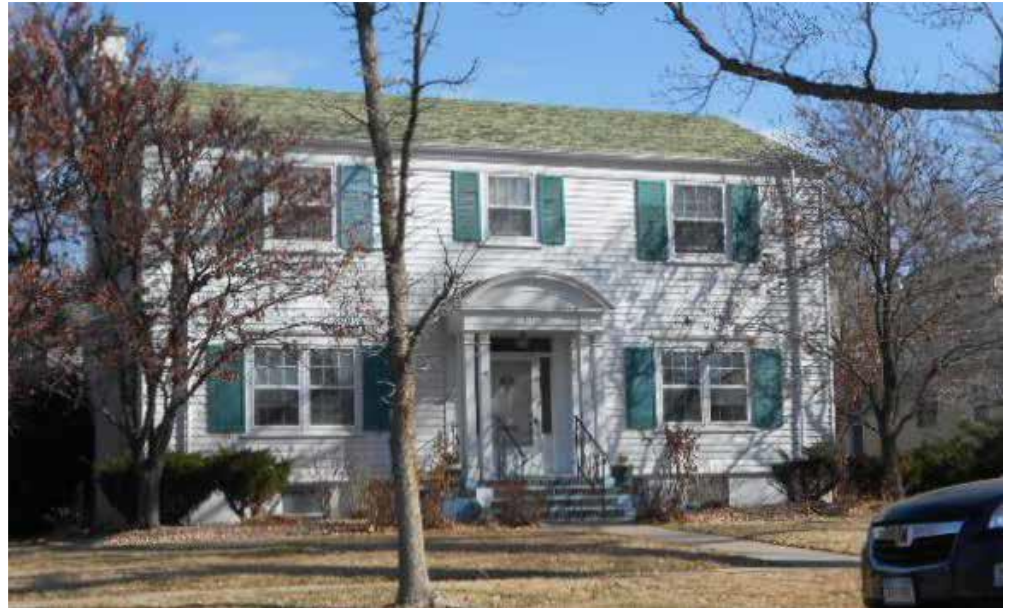
Not all houses within The District are single-story bungalows. This residence is a two-story Georgian Revival style constructed in 1935. The symmetrical arrangement of the windows, as well as the proportions of the windows, fits the Lincoln Park Historic District Standards & Guidelines.
