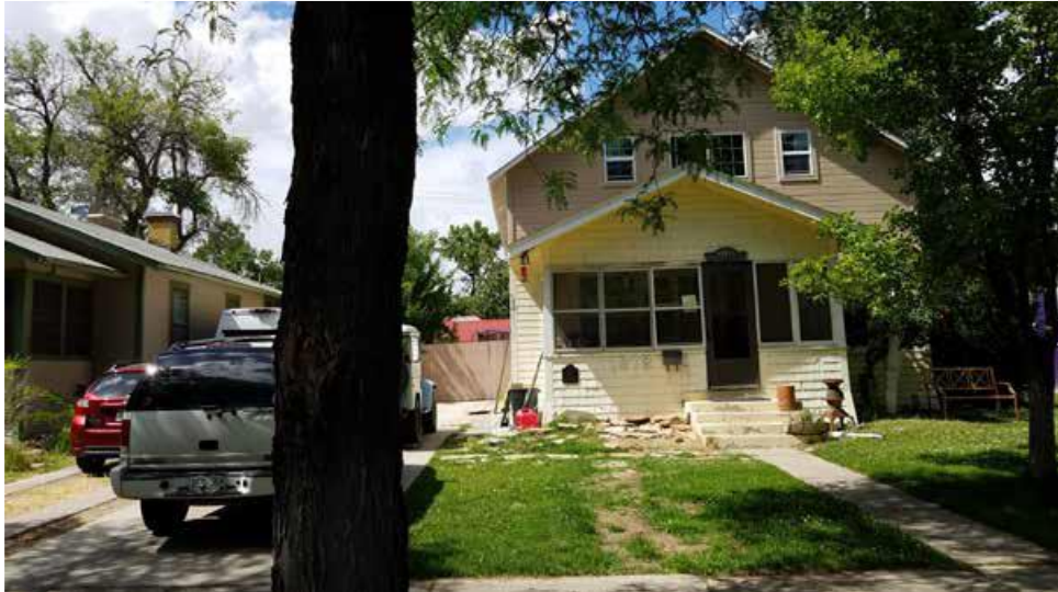
This recent second-story addition at a house on Ouray Avenue is in keeping with the tradition of the bungalow style. The short top-plate at the upper eaves minimized the overall height at the peak of the roof, reducing the appearance of height from the street. This configuration is referred to as 'story and a half.'
