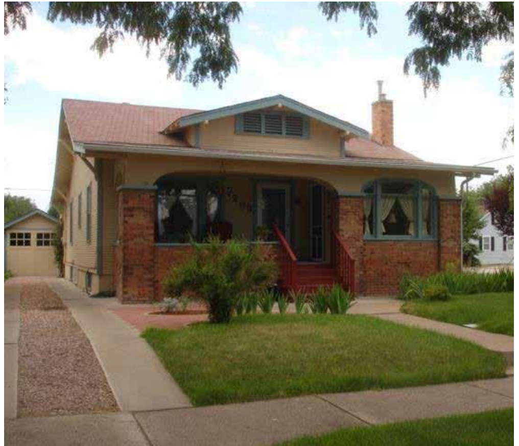
This bungalow on Ouray Avenue illustrates the typical property layout within the Lincoln Park Historic District - detached garage located behind the primary residence. The deep front porch connects the sidewalk to the front door of the house, while the large roof overhangs shade the windows from the summer sun.
