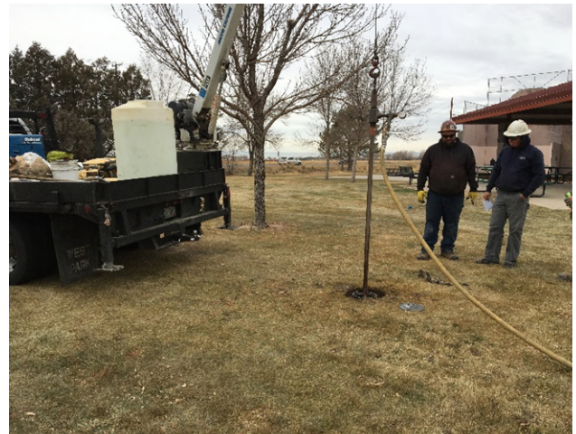
FIGURE: 4 – Developing well (MW-1).
