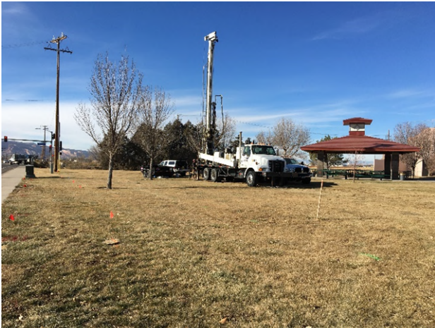
FIGURE: 1 – View west at drilling BH#2 (MW-1).
