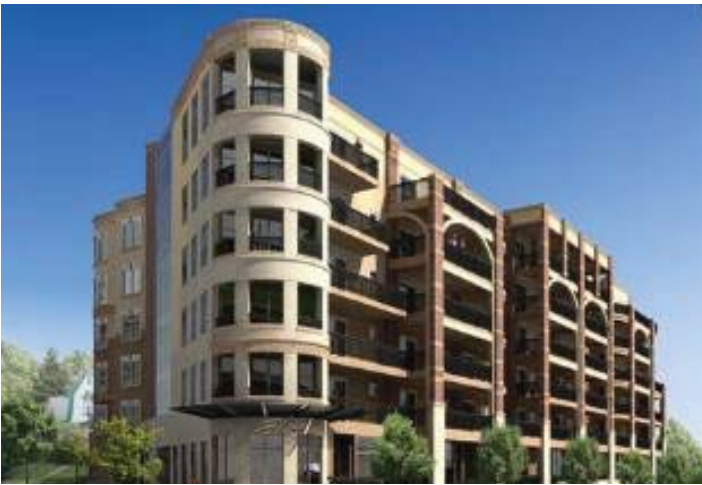
Image 23. RiverClay Condominiums represent the Rocky Mountain region's first LEED-certified multi-family project, located in Jefferson Park, Denver, Colorado. It includes 60 residential units with two commercial units in a six-story building totaling 138,000 square feet. Built by Zocalo Community Development.
