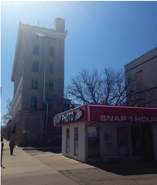
Image 14a. Existing building located in the east Rood Avenue endcap.
