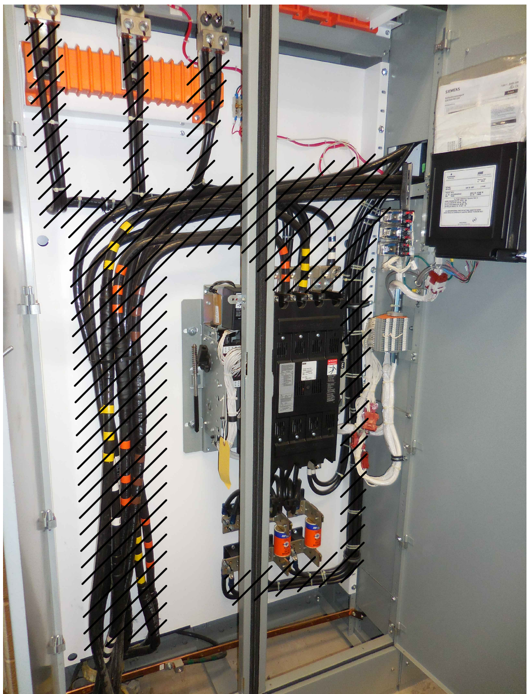
AUTOMATIC TRANSFER SWITCH CABLE DEMOLITION DETAIL
