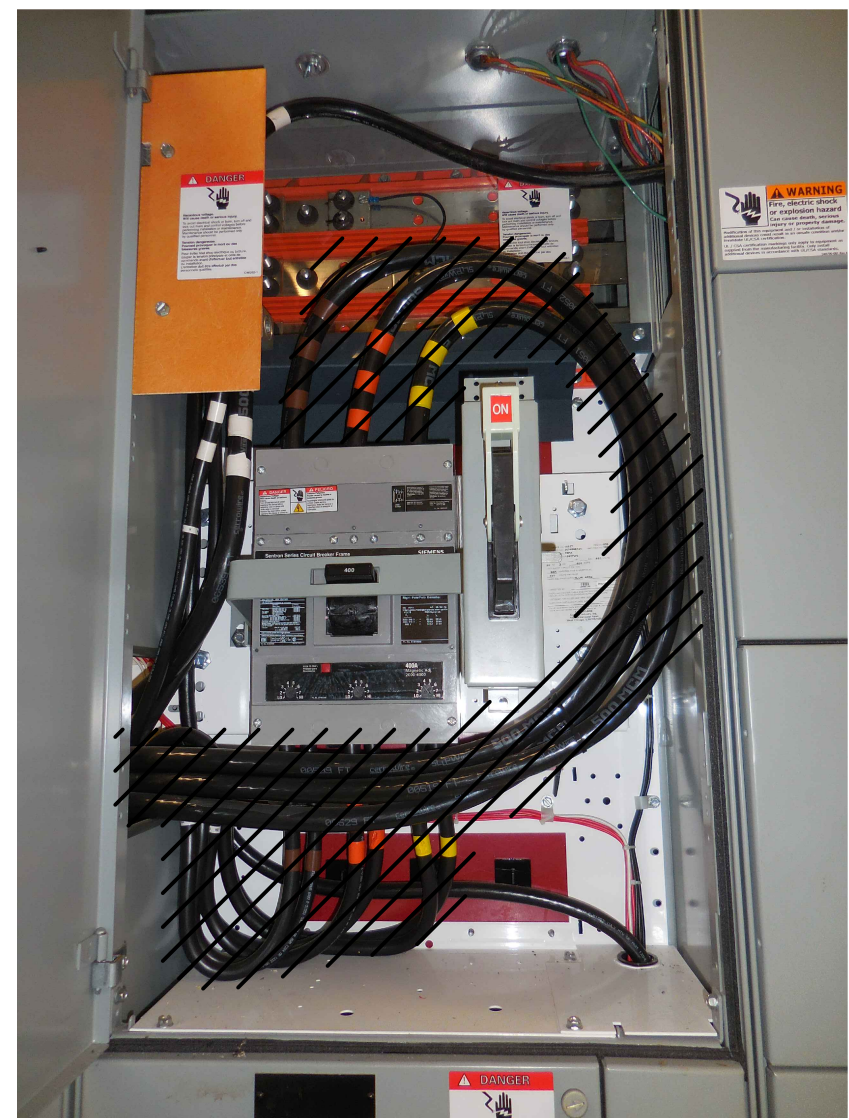
MAIN CB MCC-10 CABLE DEMOLITION DETAIL
