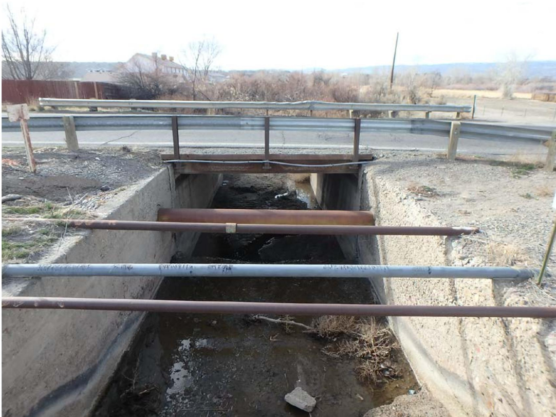
View of Bridge Side Elevation Looking Downstream
