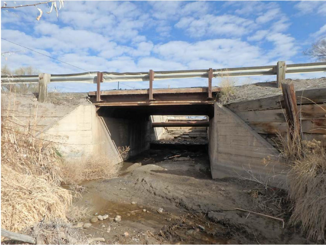
View of Bridge Side Elevation Looking Upstream
