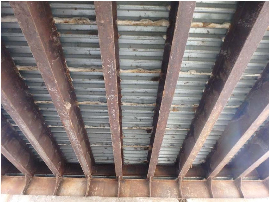
General View of Underside of Bridge Looking East
