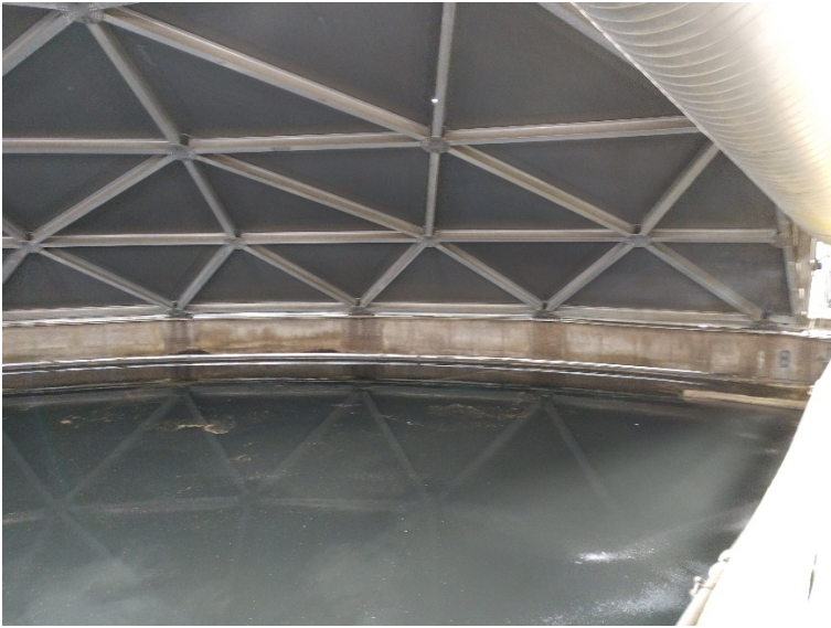
Figure 1 - Interior View of Primary Clarifier
