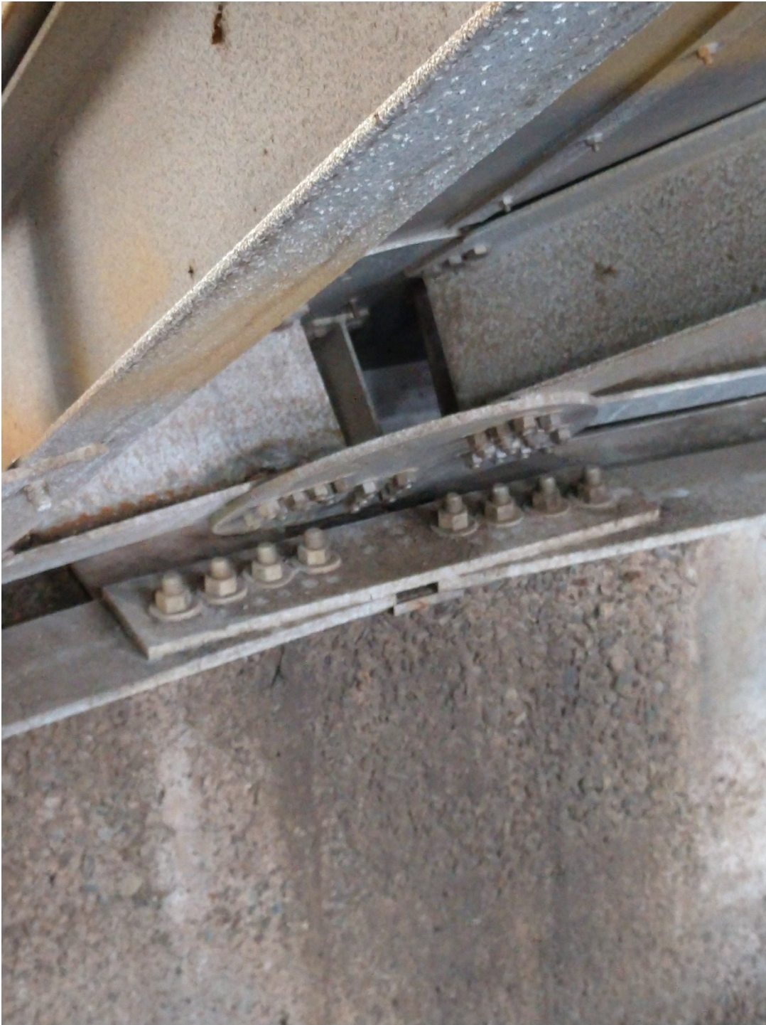
Figure 2 - Primary Clarifier Dome Anchors
