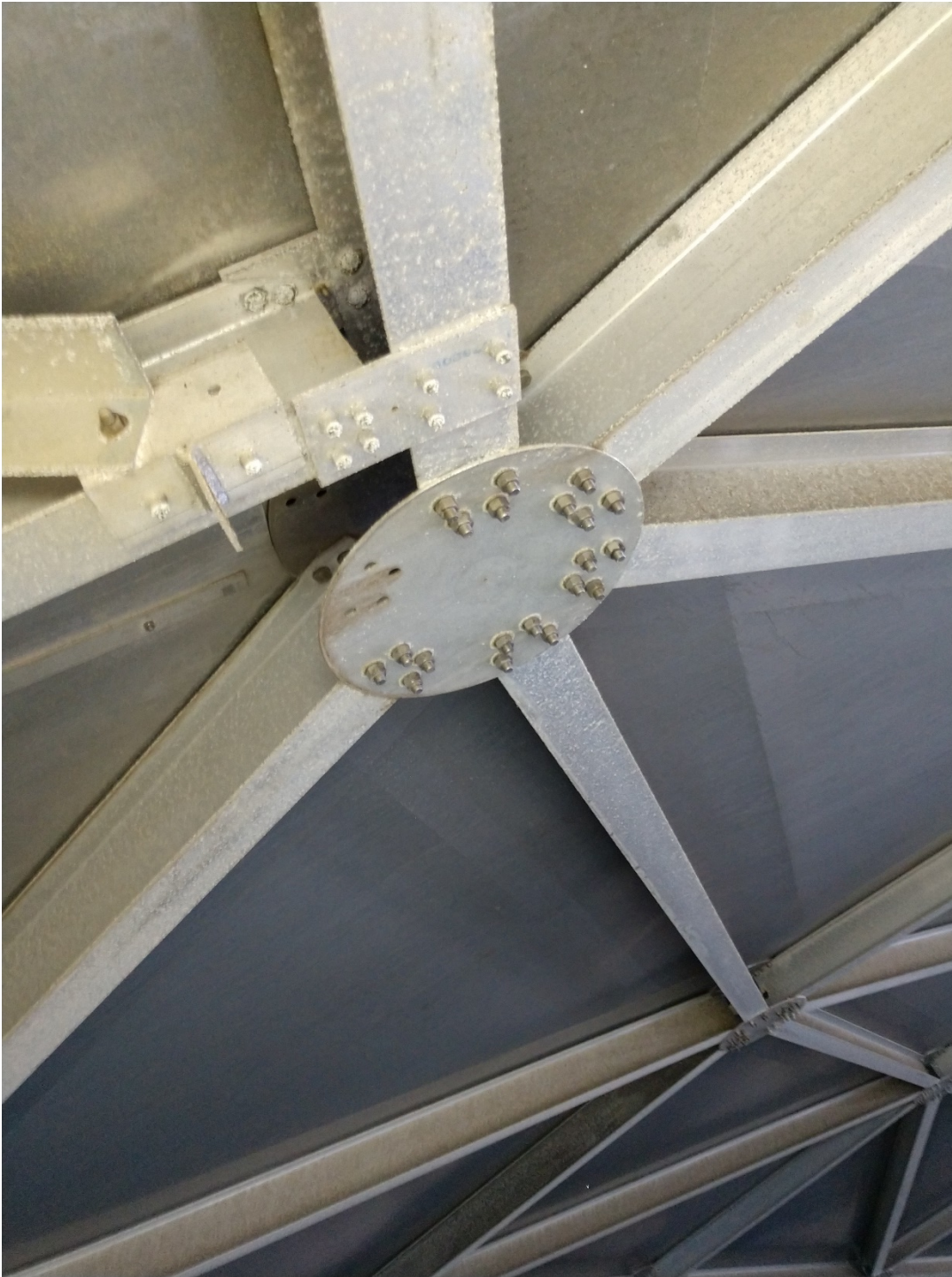
Figure 3 - Framing Connections
