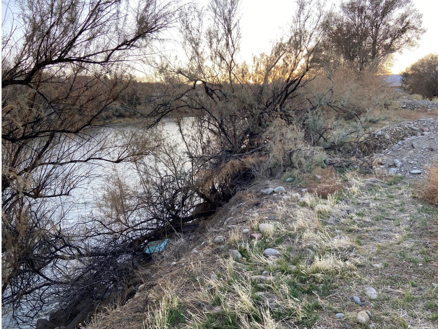
Existing Bank Conditions – November 2020
