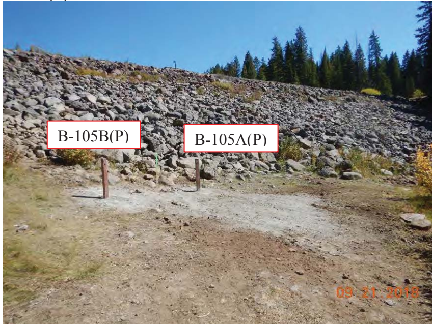
Figure 3. Riser casings to B-105A(P) on right and B-105B(P) on left in photo at the end of day, looking southeast.
