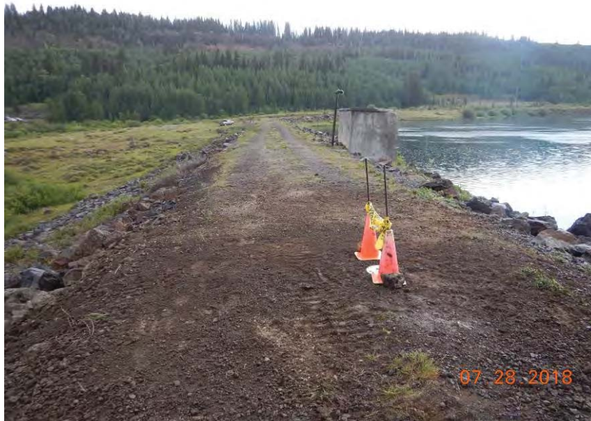
Figure 3. B-101 at end of day, looking north. Cones and caution tape placed either side of monitoring well surface mount casing.
