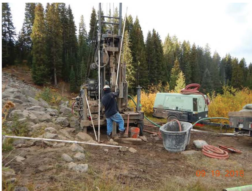
Figure 2. B-105A during monitoring well installation, looking south.
