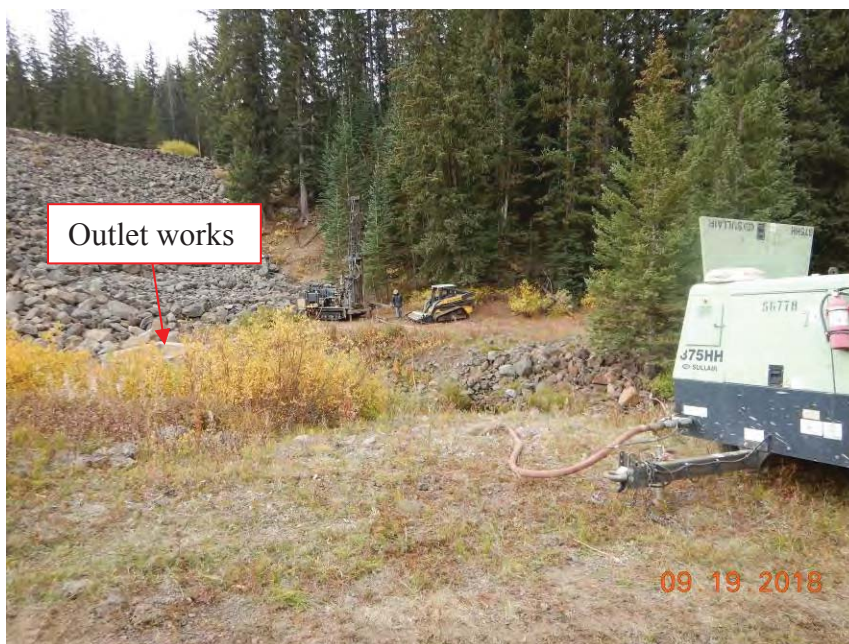
Figure 8. B-104 equipment set-up prior to drilling, looking southeast. Air compressor is right of outlet works and drill rig and skid steer are left of outlet works.
