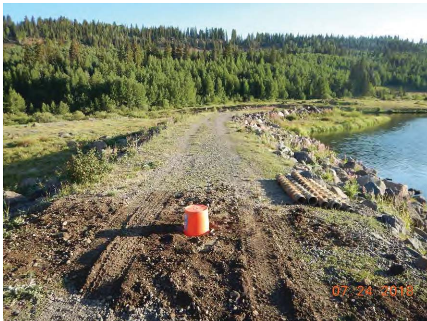
Figure 1. Monitoring well at B-103 covered with bucket while awaiting concrete backfill and well completion. Looking north.
