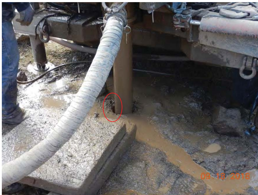
Figure 6. Area where water release was occurring at the surface, circled in red. Drilling stopped.
