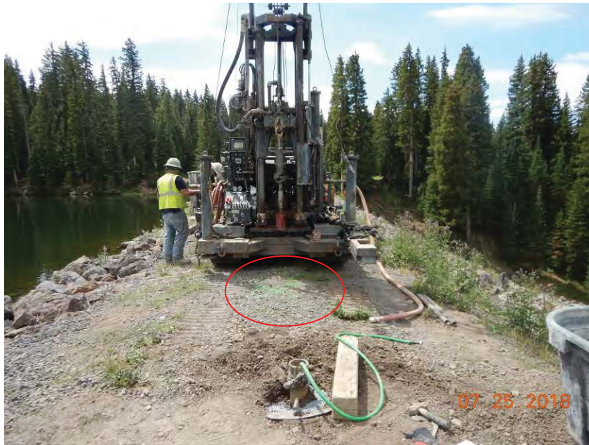
Figure 3. B-102B prior to drilling activity, boring area circled in red and indicated with green "X." Augers in foreground are in B-102A during coated pellet curing time. Looking south.
