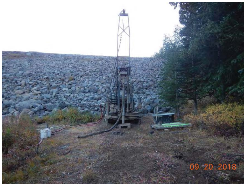
Figure 2. B-104 equipment set-up prior to drilling, looking east.
