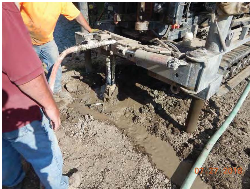
Figure 2. B-101 equipment set-up during grouting, looking southeast.
