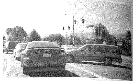
EXHIBIT 14-16 Problem resulting from an access connection located within the left-turn queue length.
