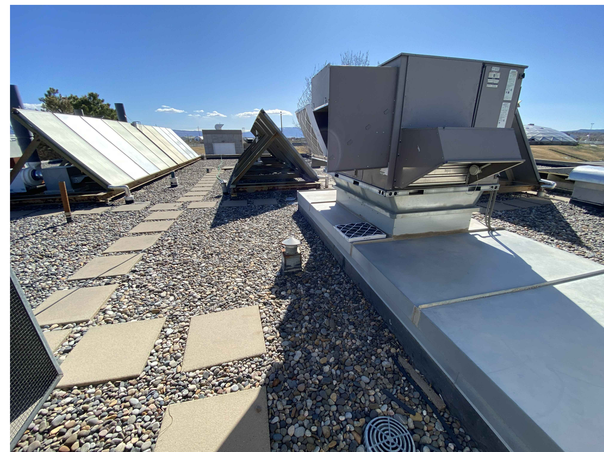
EXISTING OPERATIONS BUILDING JOHNSON CONTROLS SERIES 10
