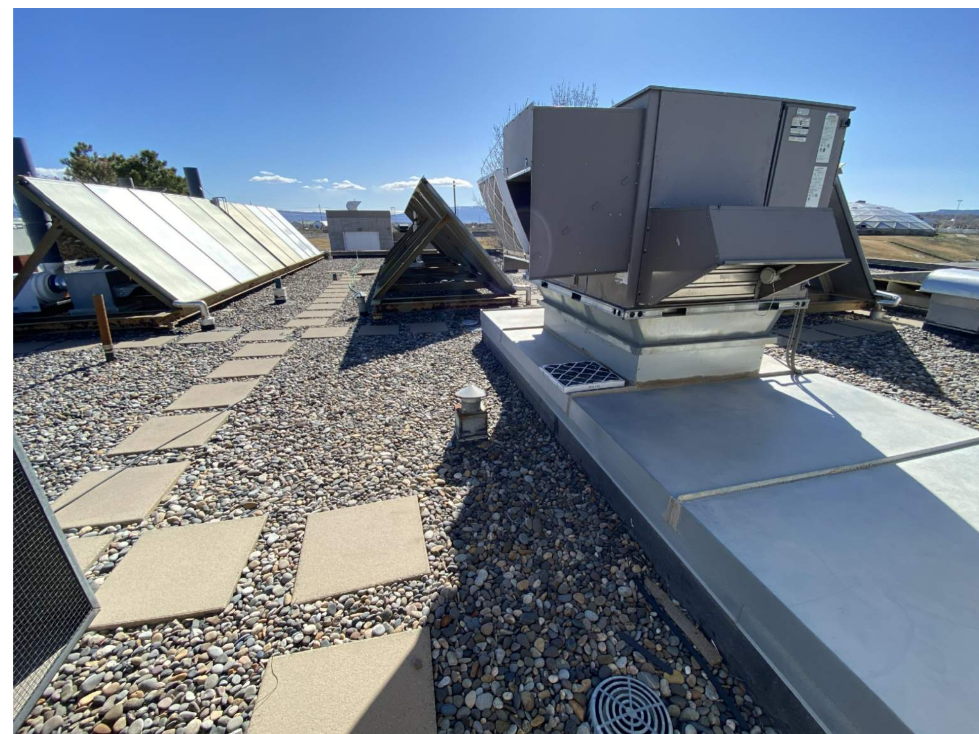
EXISTING OPERATIONS BUILDING JOHNSON CONTROLS SERIES 10
