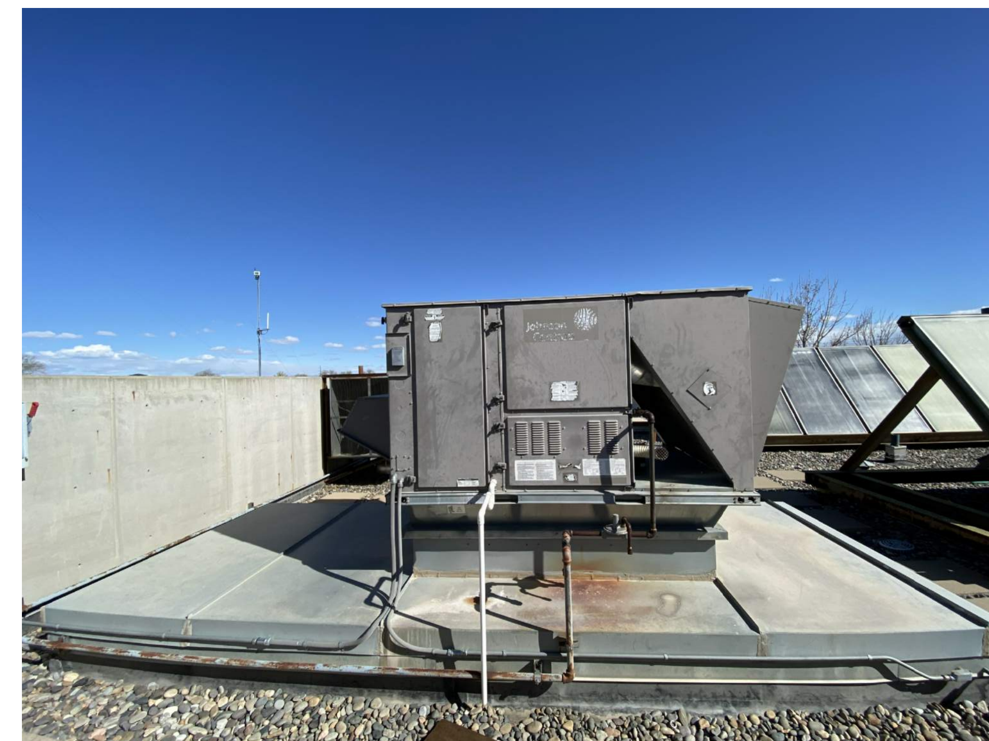
EXISTING OPERATIONS BUILDING JOHNSON CONTROLS SERIES 10
