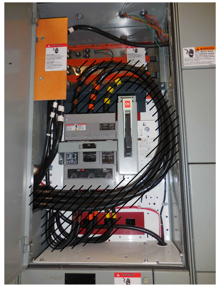
MAIN CB MCC-10 CABLE DEMOLITION DETAIL
