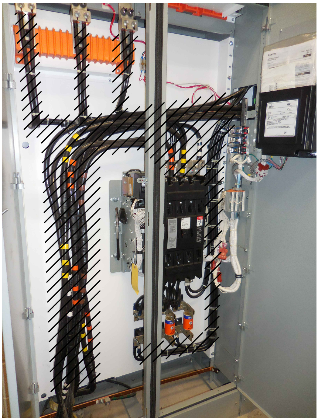
AUTOMATIC TRANSFER SWITCH CABLE DEMOLITION DETAIL
