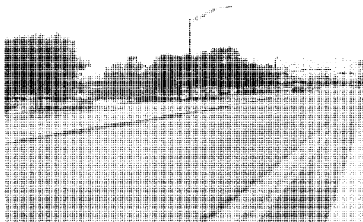
EXHIBIT 14-15 Nontraversable median installed circa 2009 on Southwest Parkway at Texas Avenue, College Station, Texas, as a retrofit action to restrict left turns at a driveway serving a strip commercial center.
