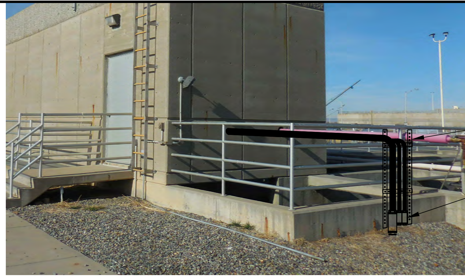
GENERATOR CONDUIT ROUTING DETAIL
