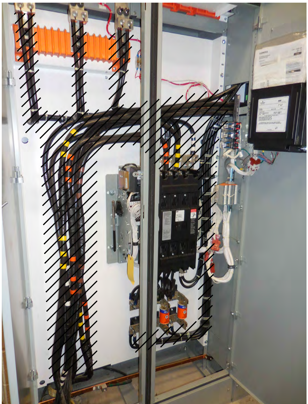
AUTOMATIC TRANSFER SWITCH CABLE DEMOLITION DETAIL
