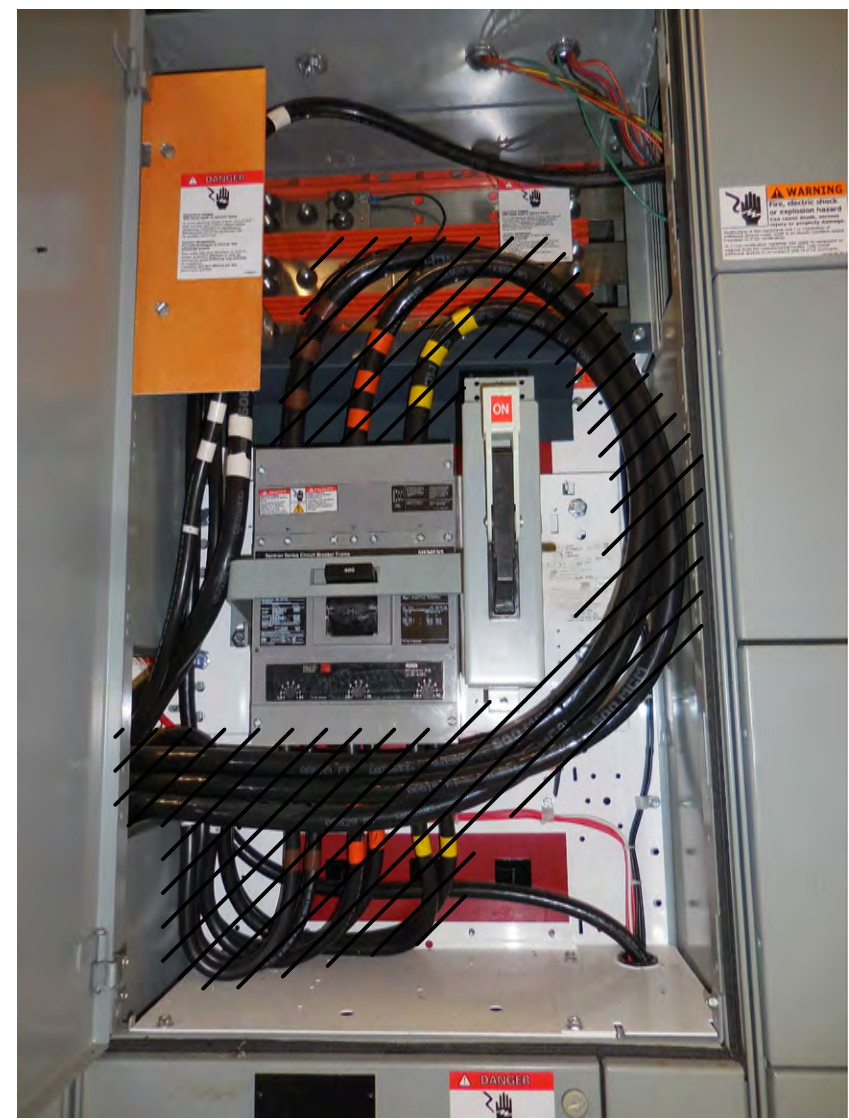
MAIN CB MCC-10 CABLE DEMOLITION DETAIL
