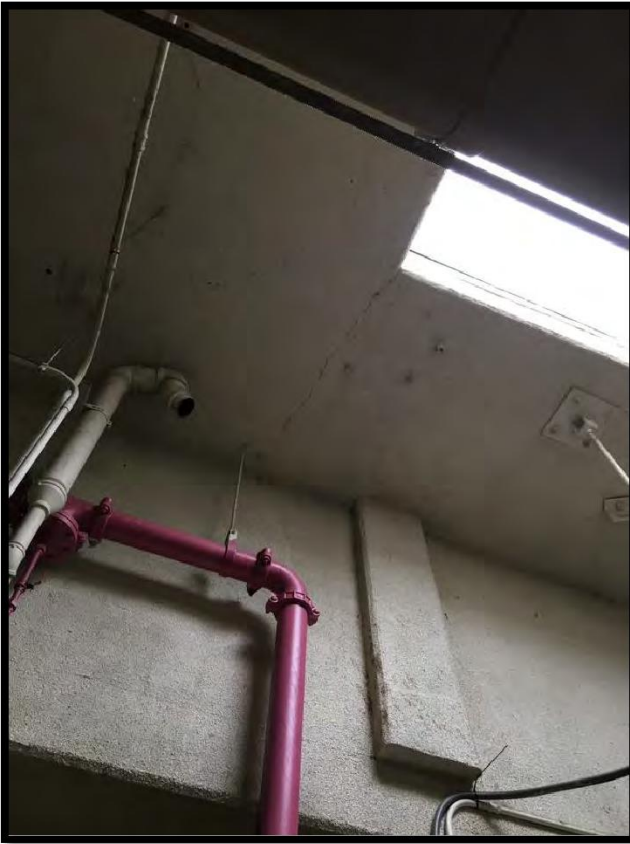
Picture 19 A&B, Aerobic Basement Ceiling Crack
