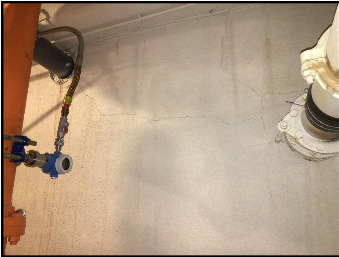
Picture 30, Anaerobic Digester Tank Wall
