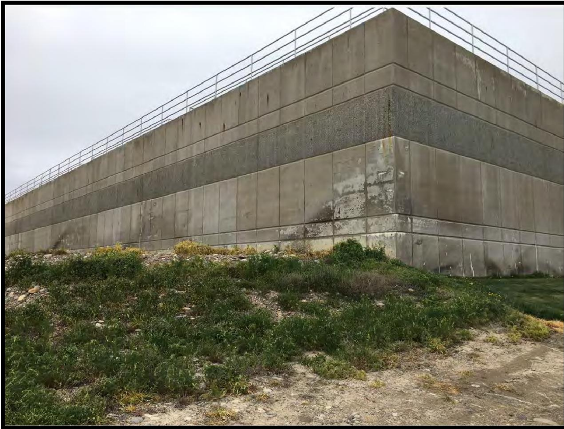
Picture 23, Aerobic Digester
