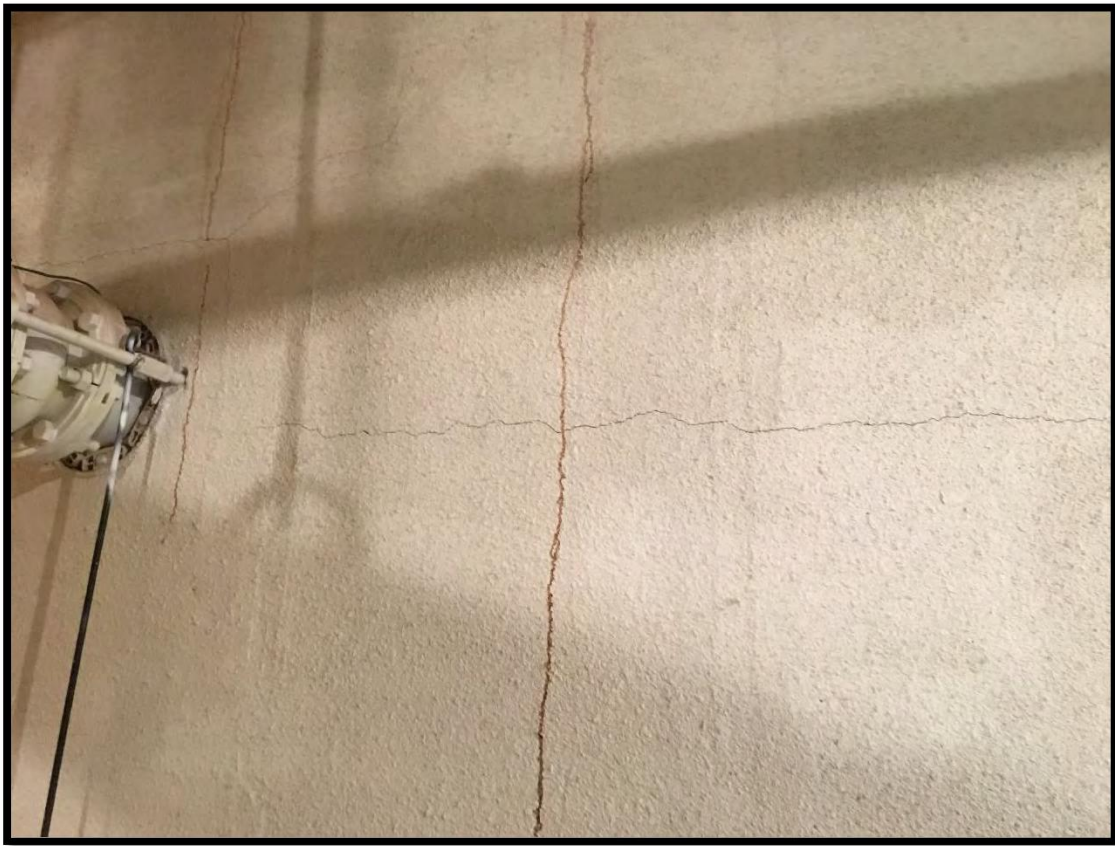
Picture 31, Anaerobic Digester Tank Wall
