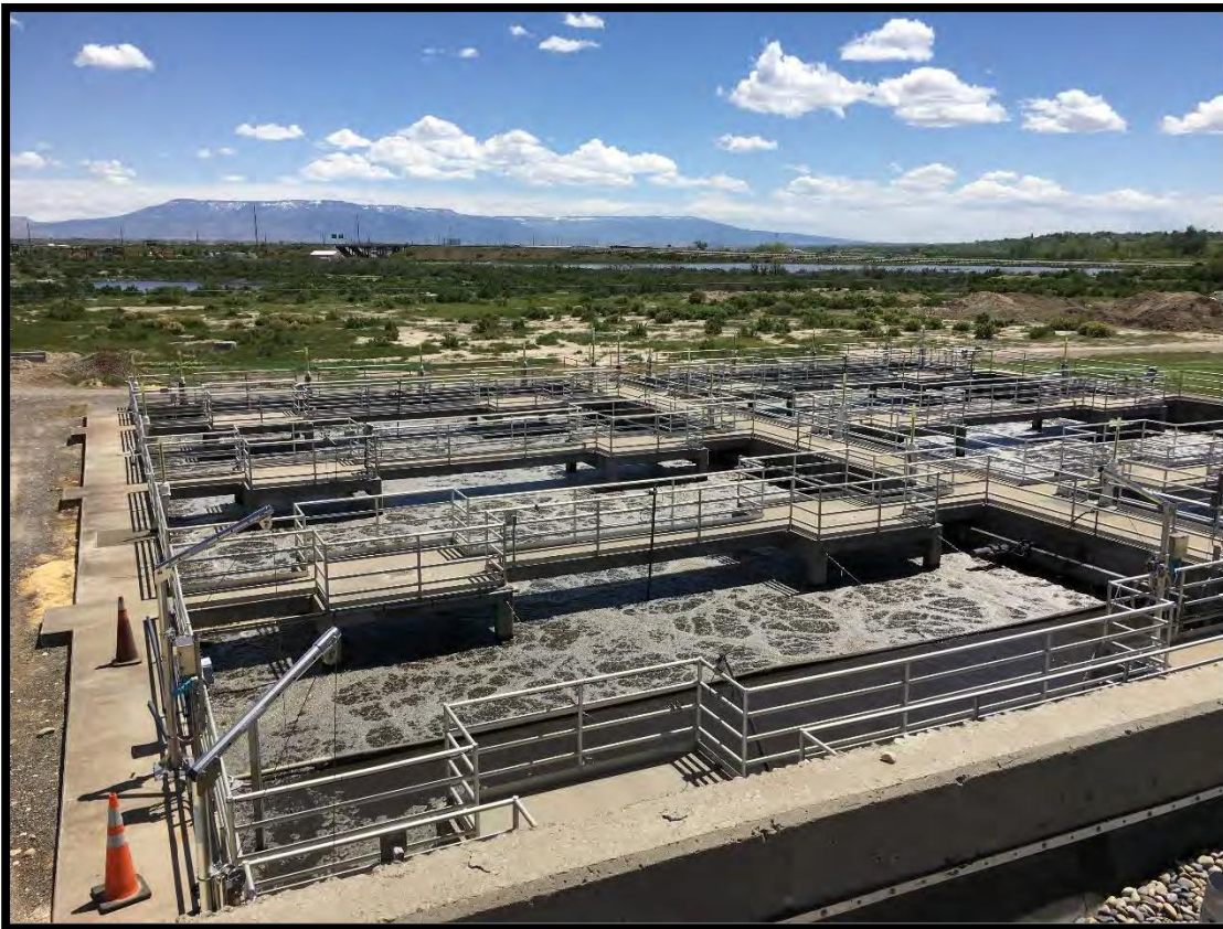
Picture 20, Aeration Basin
