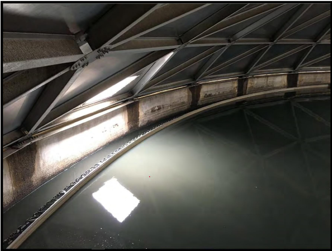
Picture 8, Primary Clarifier Wall and Roof
