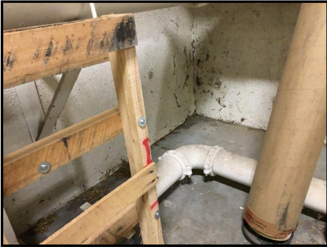
Picture 27, Aerobic Digester Basement Floor & Wall
