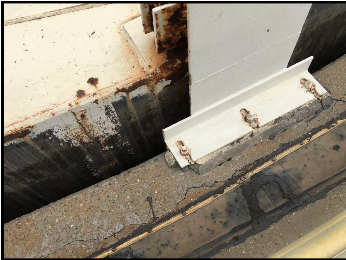
Picture 34, Top of Anaerobic Digester Digester Tank Wall
