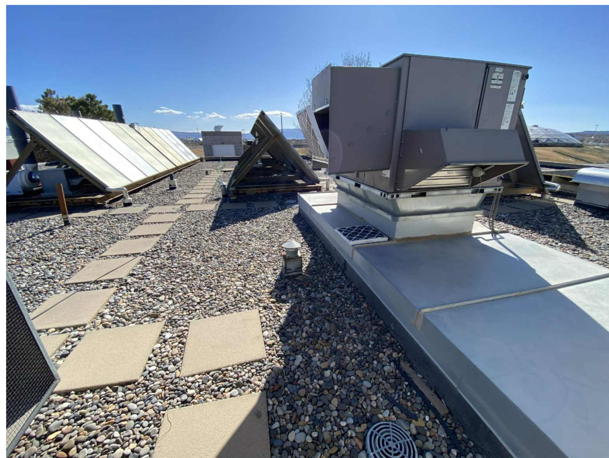
EXISTING OPERATIONS BUILDING JOHNSON CONTROLS SERIES 10
