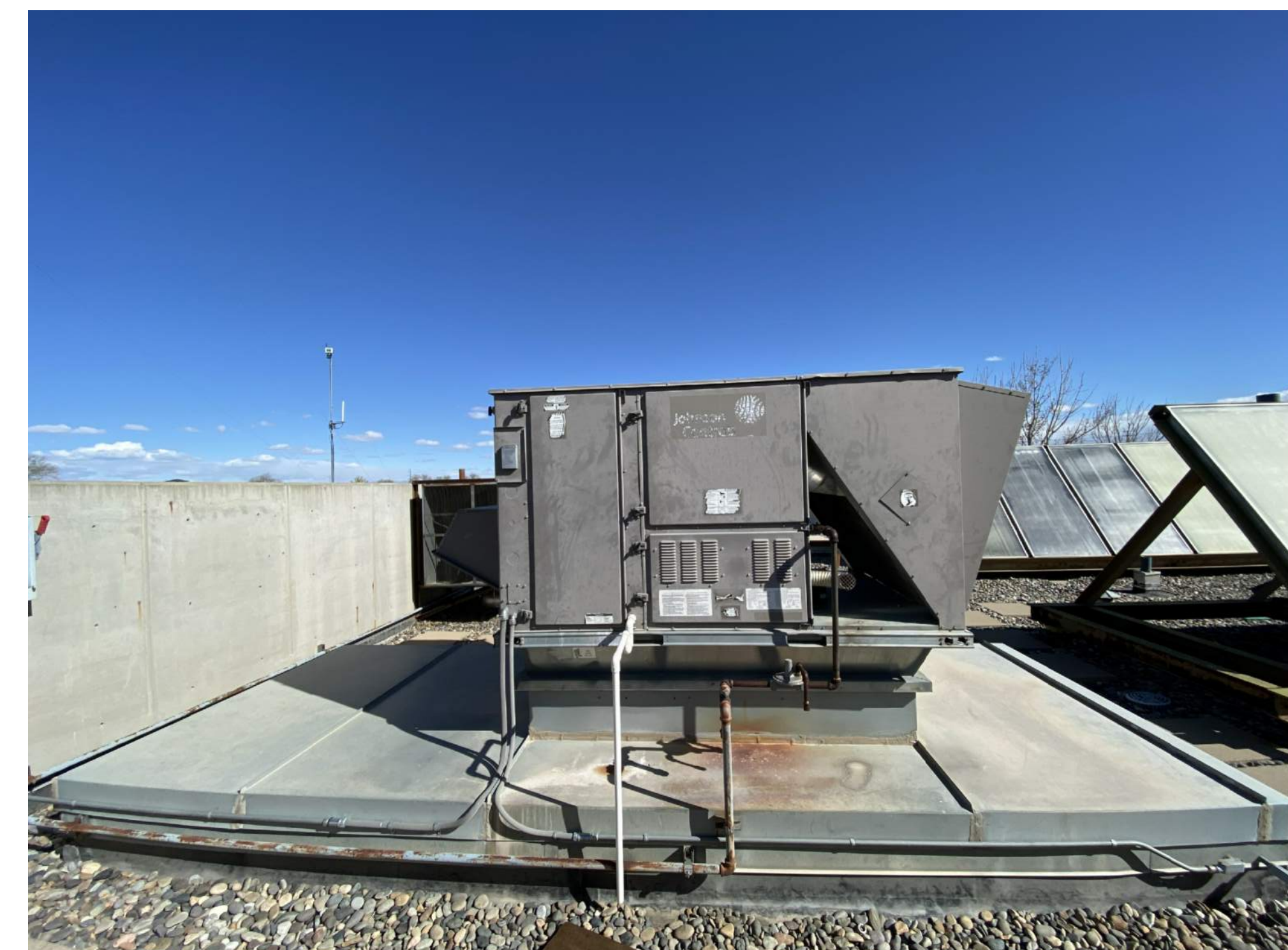
EXISTING OPERATIONS BUILDING JOHNSON CONTROLS SERIES 10
