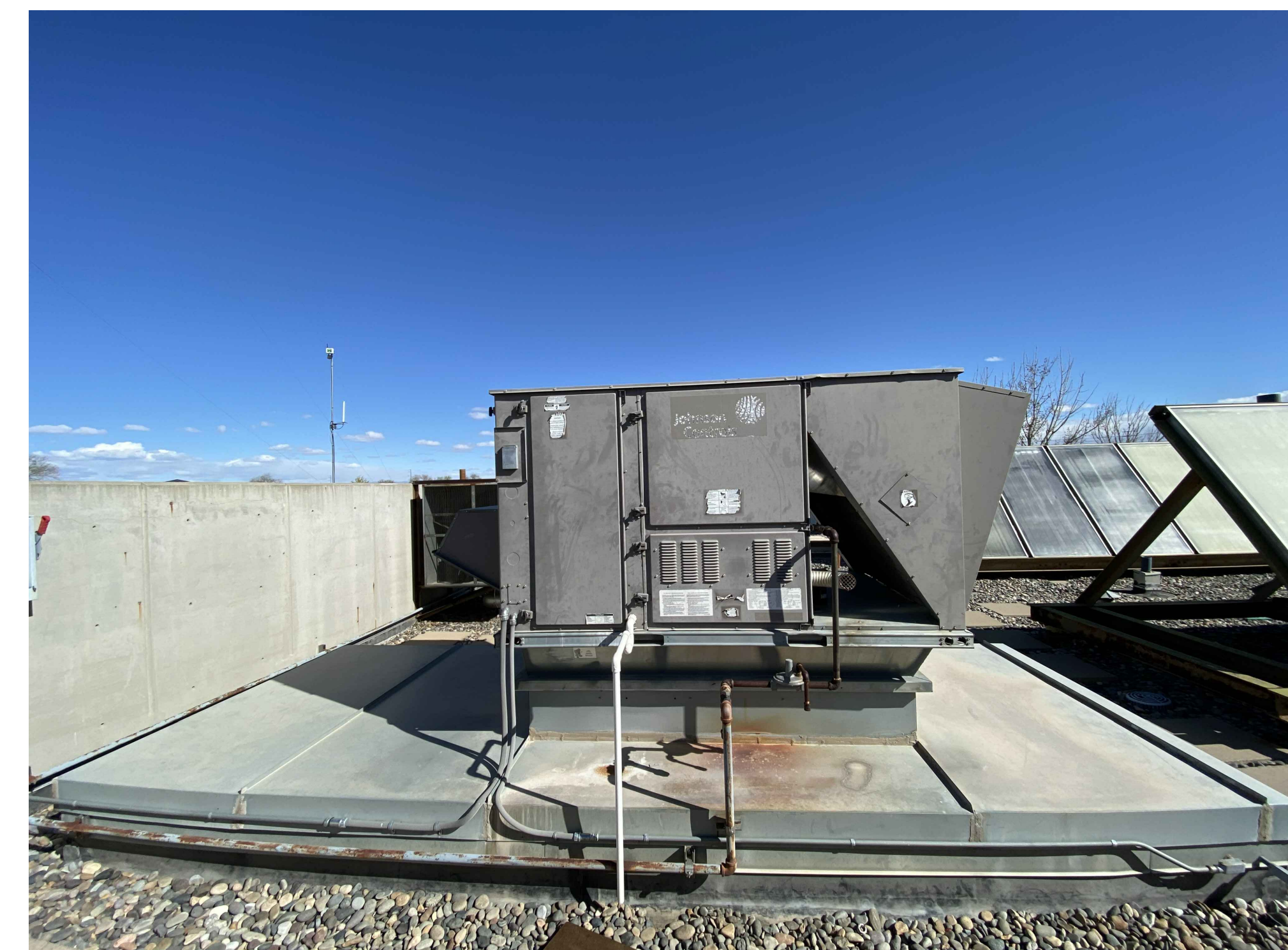
EXISTING OPERATIONS BUILDING JOHNSON CONTROLS SERIES 10
