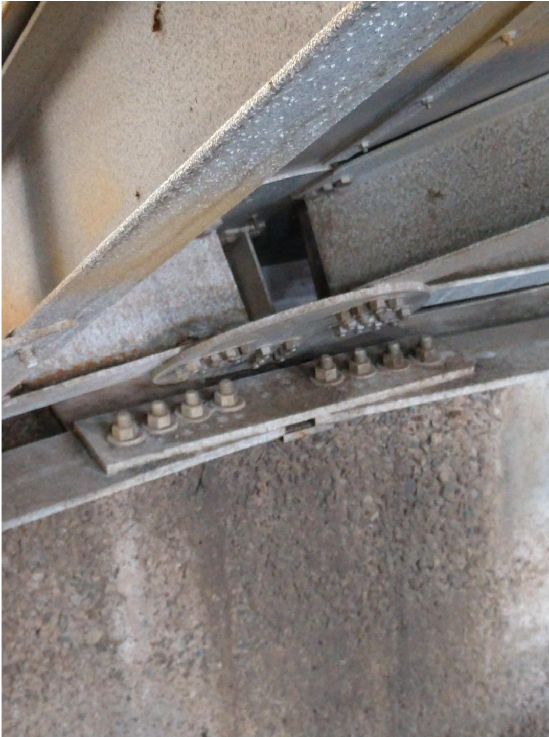
Figure 2 - Primary Clarifier Dome Anchors
