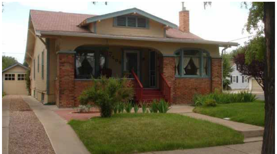
Primary entrance is elevated with stairs, and in this case – like many in the neighborhood - the home is adorned with an elevated front porch. This one is open, some are screened or fully enclosed.
