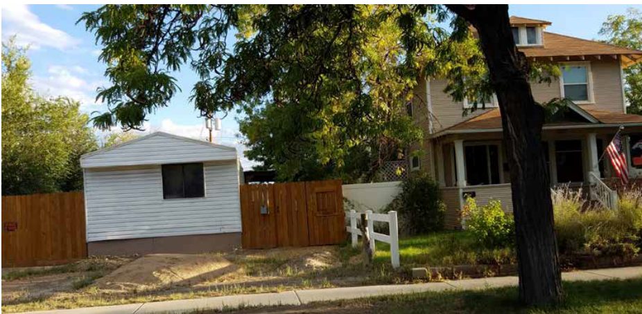
This is an example of a non-compatible manufactured home - Single-wide; it has no front entrance; and is incompatible with adjacent historic home to the right.
