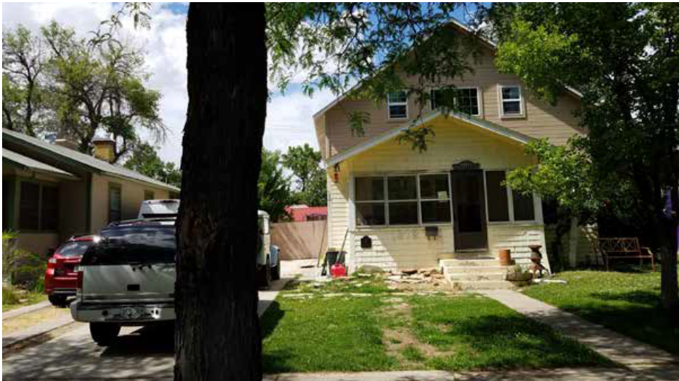
This recent second-story addition at a house on Ouray Avenue is in keeping with the tradition of the bungalow style. The short top-plate at the upper eaves minimized the overall height at the peak of the roof, reducing the appearance of height from the street. This configuration is referred to as 'story and a half.'
