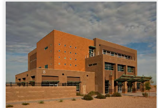
City of Phoenix Fire Dispatch Center
