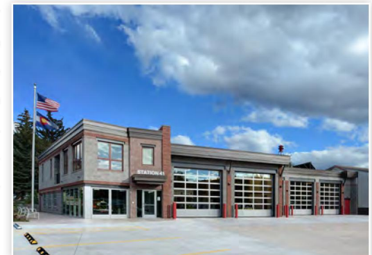
Basalt Fire Station No. 41
