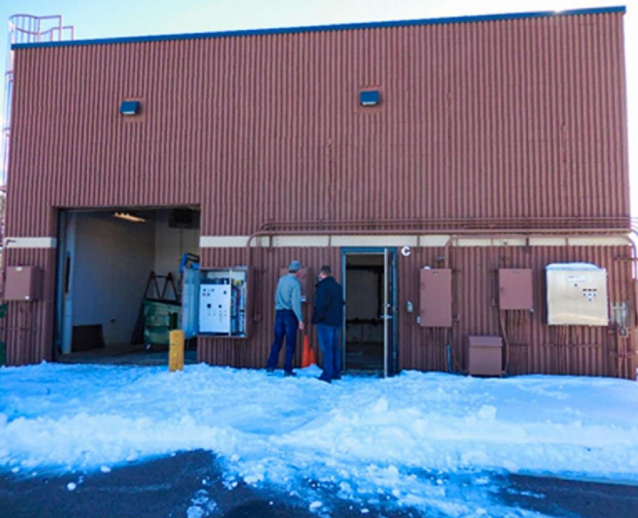
Stonegate Headworks WWTP
