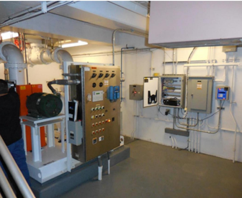
Interior of Lift Station #3
