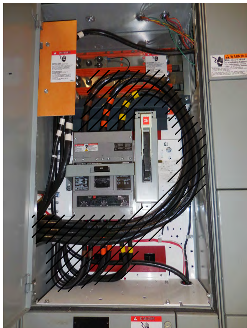
MAIN CB MCC-10 CABLE DEMOLITION DETAIL
