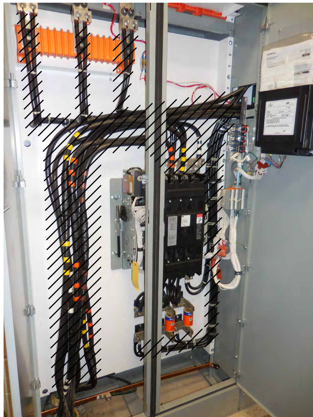
AUTOMATIC TRANSFER SWITCH CABLE DEMOLITION DETAIL
