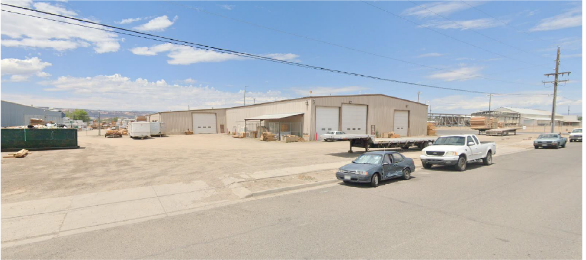
1101 Winters Avenue – Site Viewed from Southeast Corner of Property
