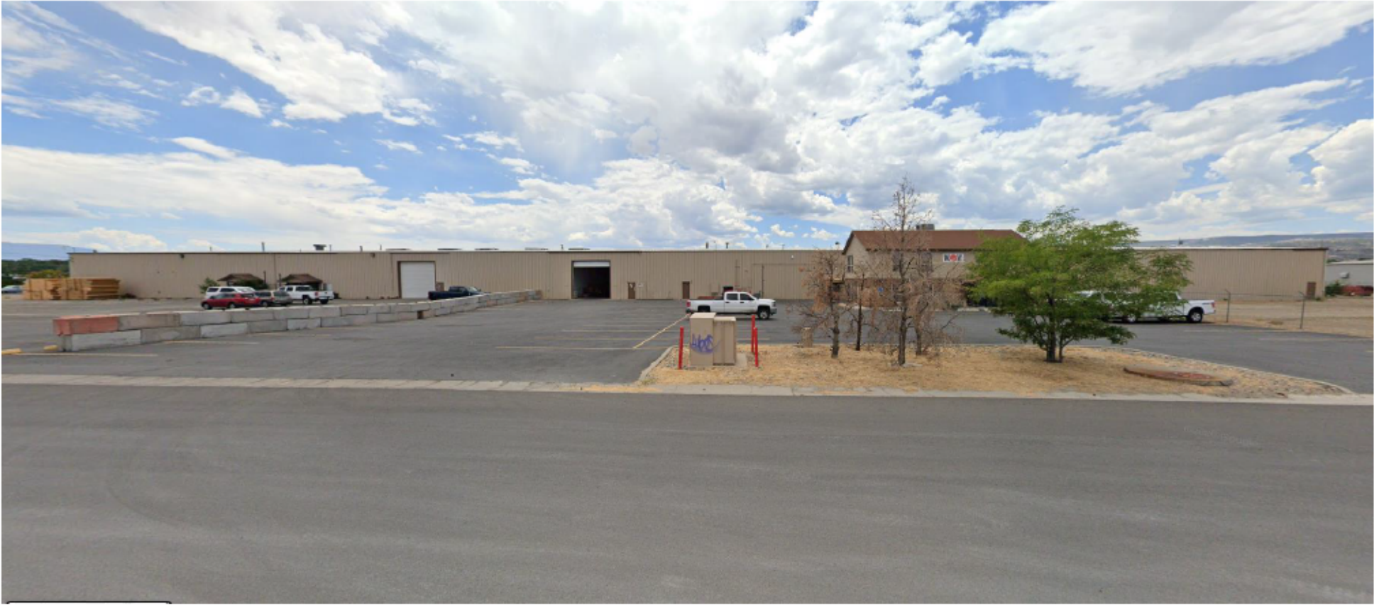
1101 Winters Avenue – North-Facing Façade Existing Building
