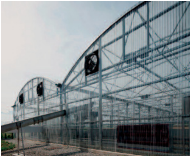
Figure 5.37 Sludge Conveyance to Solar Drying Facility
