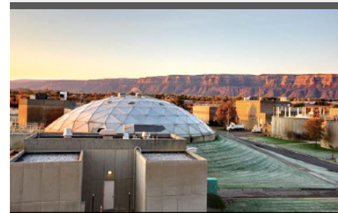
Persigo Wastewater Treatment Facility
