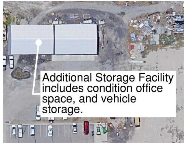
Figure 7.8 Additional Storage Facility
