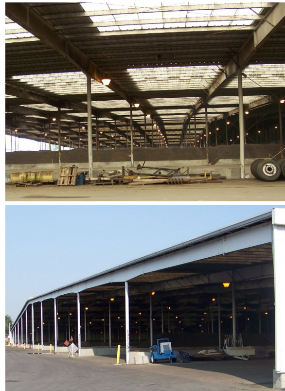
Figure 5.41 Examples of Metal Building Cake Storage Facility
