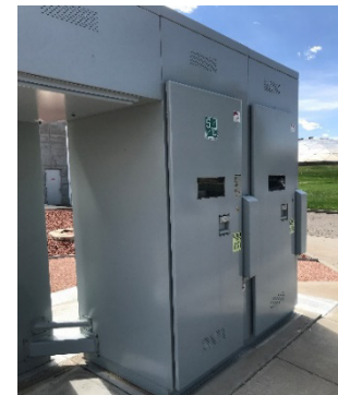
Primary switchgear.
