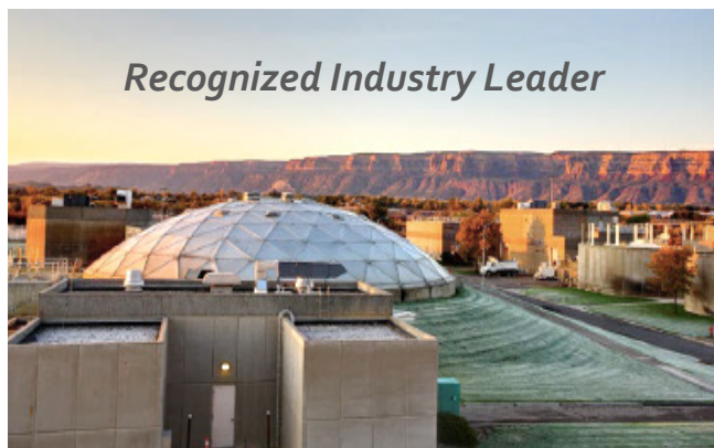
Persigo Wastewater Treatment Facility
