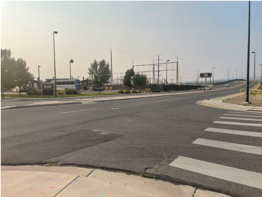
Figure 5. Sidewalk curb cuts and crosswalk west of 5th Street do not align with the pedestrian refuge island at the 5th Street Intersection.
