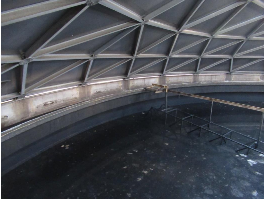
Figure 25. Overall view of the interior of the primary clarifier
