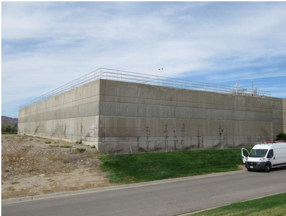
Figure 42. Overall view of the east elevation of the Aerobic Digester
