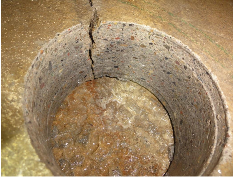
Figure 23. Topside of structural slab present after removal of topping slab. Note that the topping slab crack does not continue into the structural slab below.
