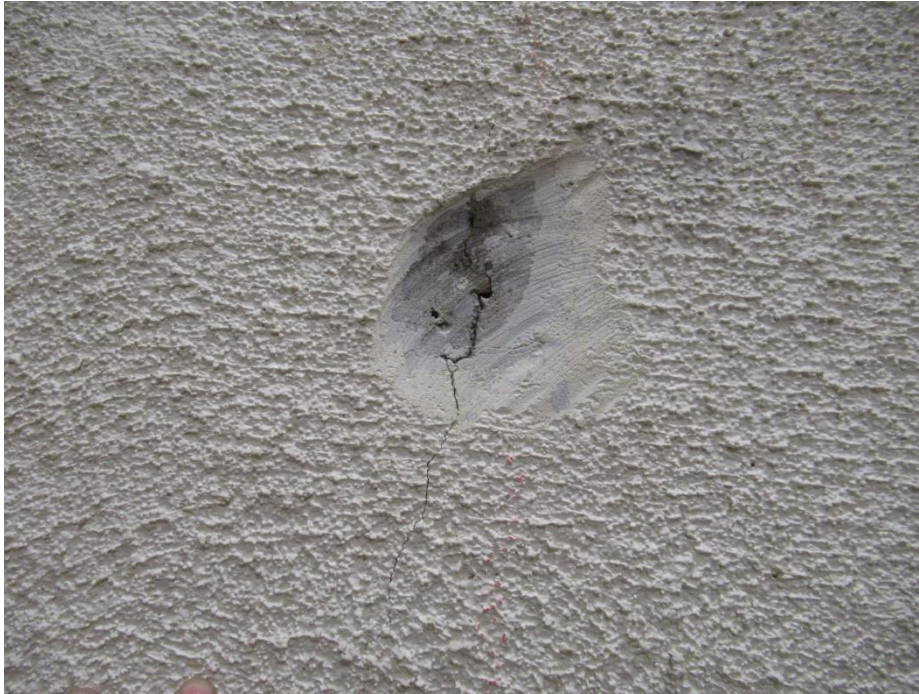
Figure 1. Typical coating installation at interior wall surfaces
