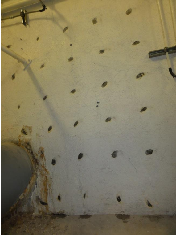
Figure 19. Overall view of HCP testing at north elevation wall
