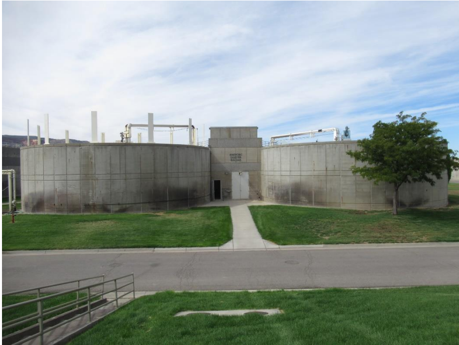
Figure 73. Overall view of the east elevation of the Anaerobic Digesters, with the Anaerobic Digester Building situated in the center
