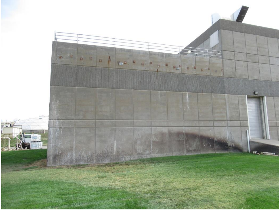
Figure 61. Overall view of the northwest corner of the Sludge Processing Unit
