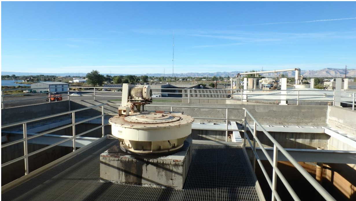
Figure 62. Overall view of the open-air framing above the blending tank
