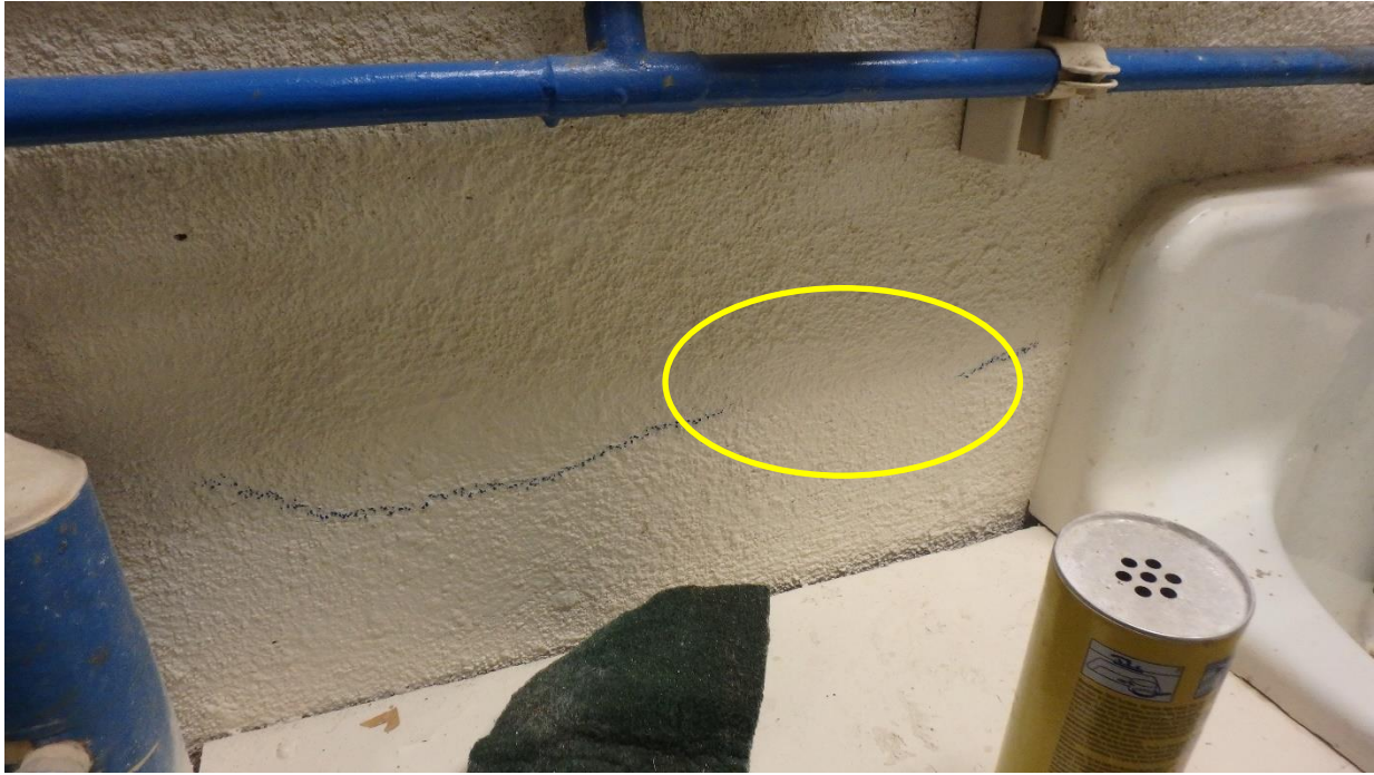
Figure 75. Previous coating repair location at the south digester interior wall
