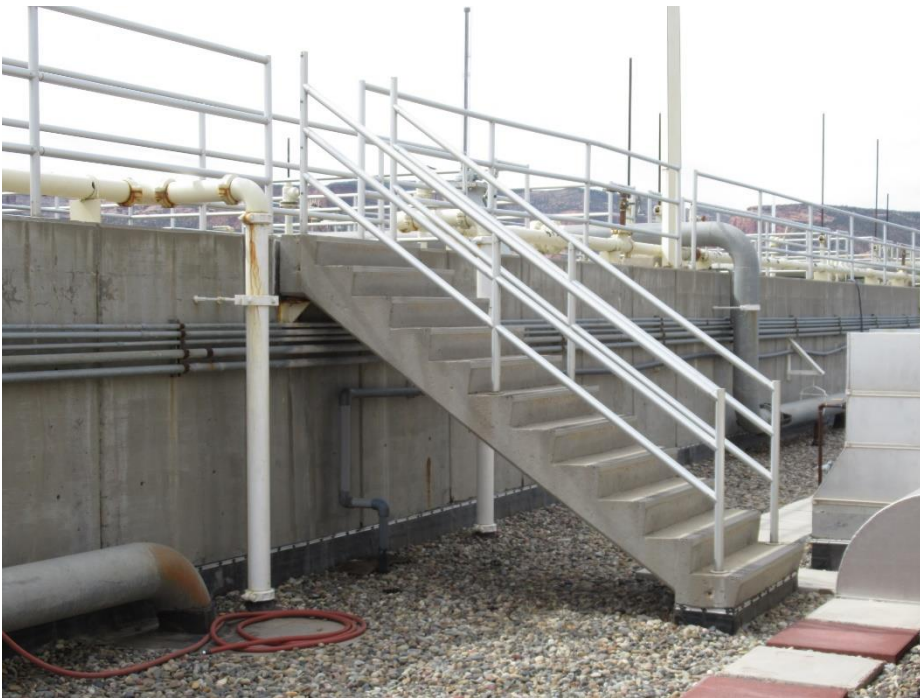
Figure 44. Stairwell leading to Aerobic Digester catwalks
