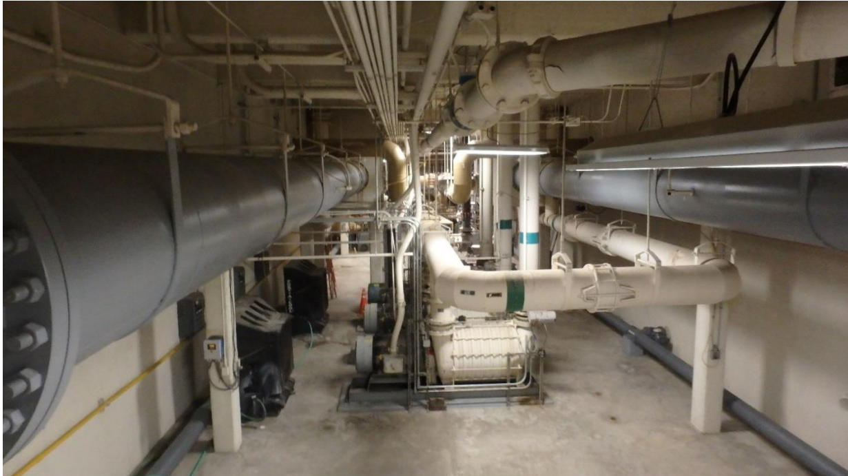
Figure 36. Overall view of the blower room, looking south
