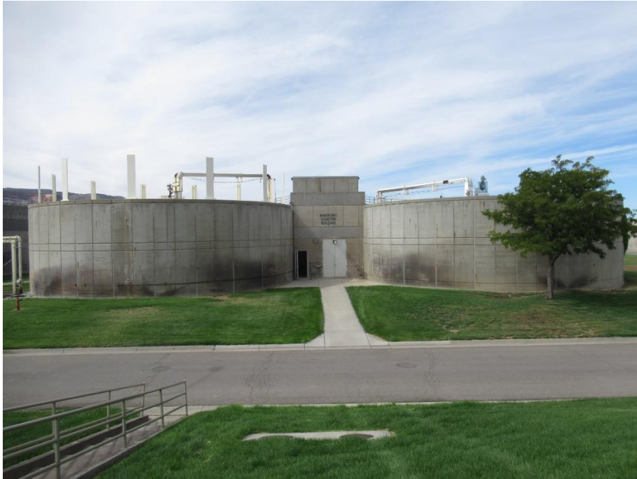
Figure 93. Overall view of the east elevation of the Anaerobic Digesters, with the Anaerobic Digester Building situated in the center
