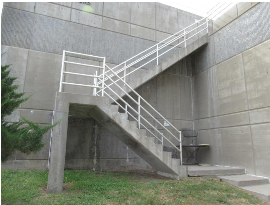
Figure 55. Ground level stairs located at northeast corner of Aerobic Digester
