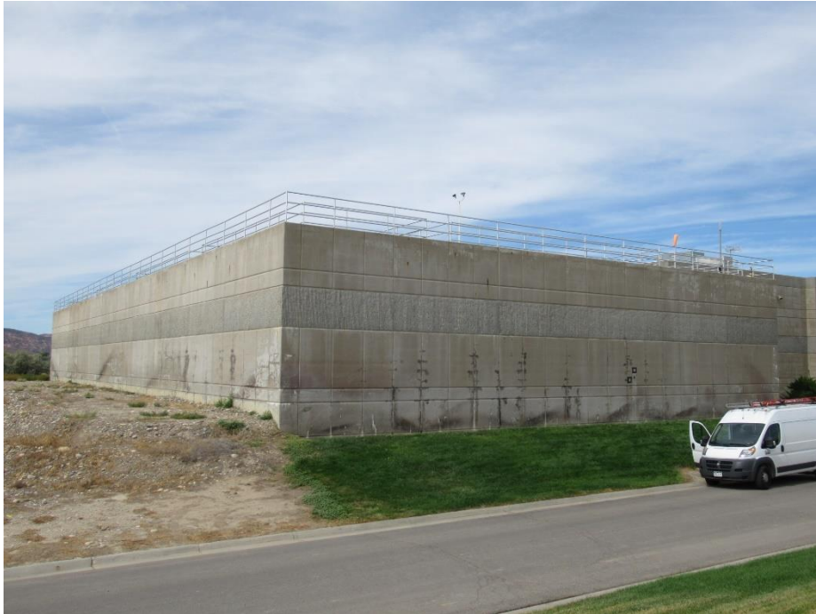
Figure 54. Overall view of the east elevation of the Aerobic Digester
