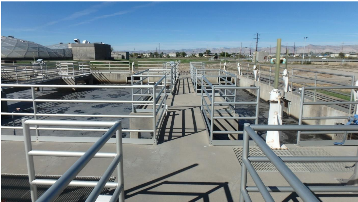
Figure 37. Overall view of the catwalks, looking north
