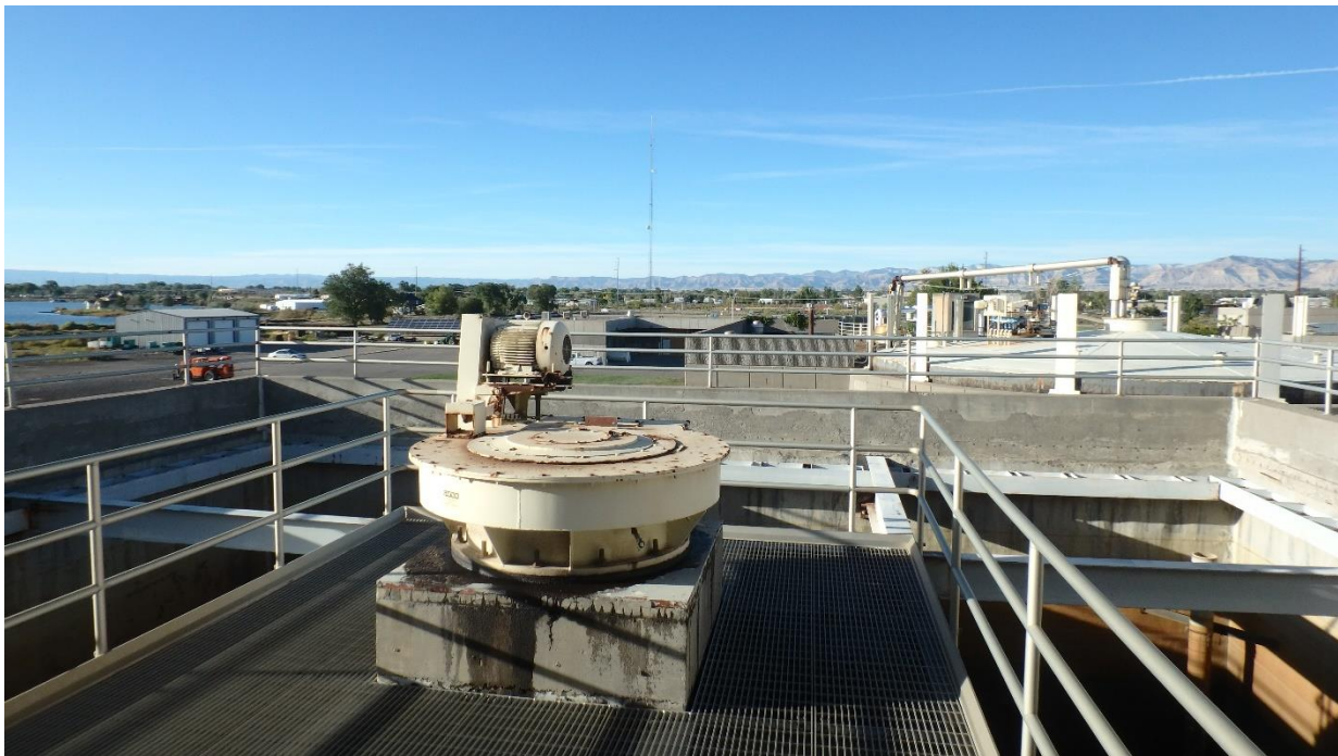
Figure 79. Overall view of the framing above the blending tank
