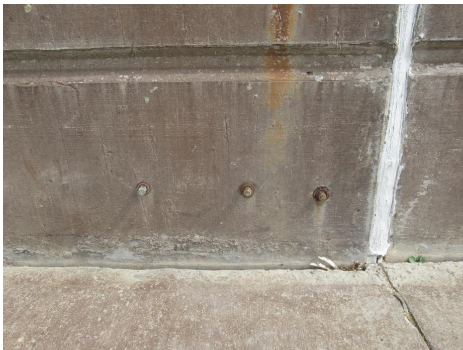
Figure 101. Supplemental attachment bolts at one panel at the south digester
