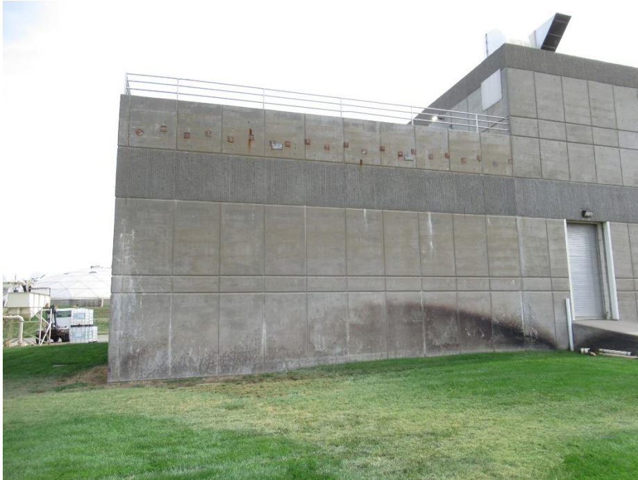
Figure 78. Overall view of the northwest corner of the Sludge Processing Unit
