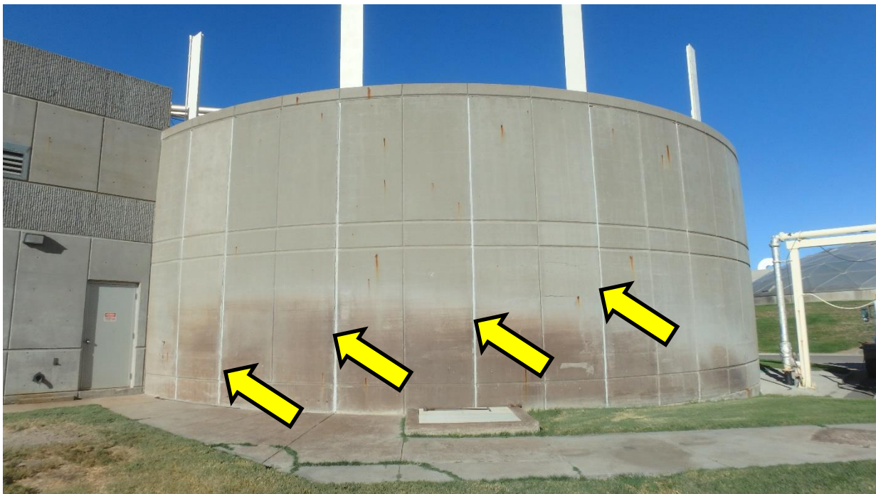
Figure 94. Overall view of the exterior panels and sealant joints (arrows)
