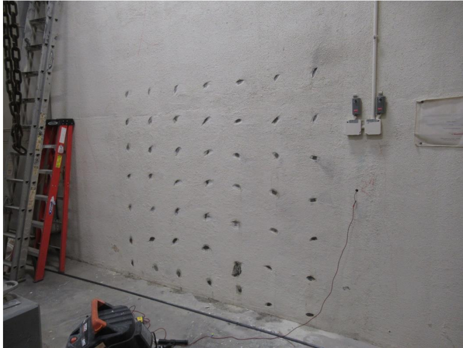
Figure 19. Overall view of HCP testing at south elevation wall
