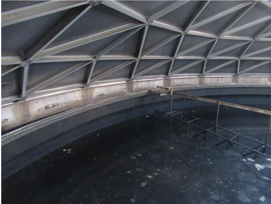
Figure 26. Overall view of the interior of the primary clarifier
