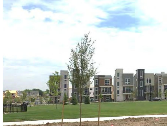
Figure 10: Single-family detached homes on small lots. In Littleton Village, these tall, narrow single-family detached homes provide additional density with a much smaller building footprint and on much smaller lots. Similar products may be appropriate in some locations in Parker, provided appropriate design and development standards are in place.
