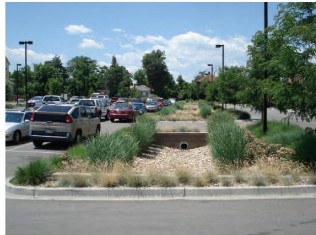
Figure 19: Bioretention swale. The bioretention swale in the image above collects water from the parking area to slow runoff and improve water quality before it leaves the site. These types of green infrastructure options can be encouraged through reduced parking incentives.
