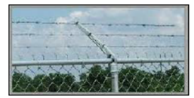
F 3-STRAND BARBED WIRE SECURITY TOP NOT TO SCALE
