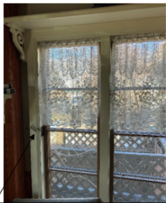
Inside. Since the window is an awning window, the mechanism is located halfway up the window on the side, instead of at the bottom like an actual casement window. This has put undue stress on the mechanism and the window, affecting its operation. Also, the snap-in screens are starting to splinter apart in multiple places.
